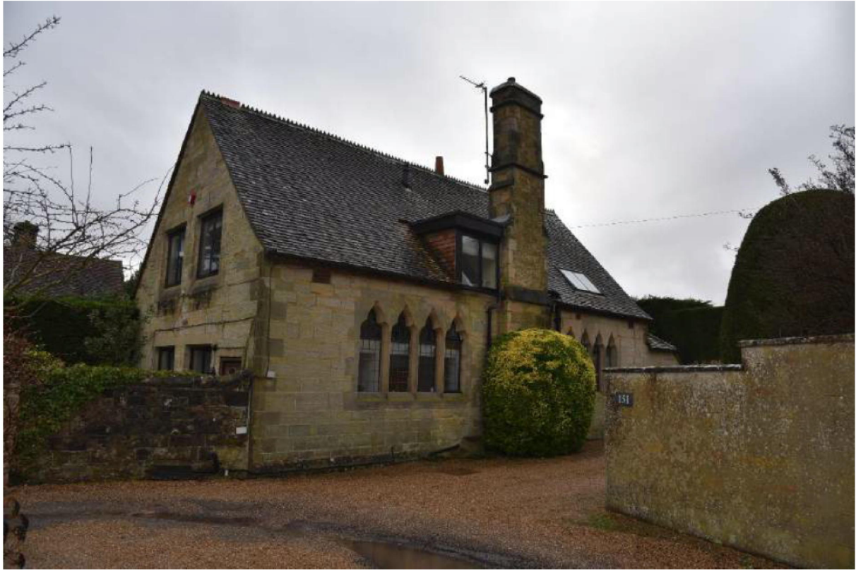
Plate 31: The north school building, facing south-west.
