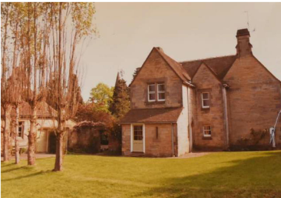
Plate 12: The house prior to its extension (provided by client).
