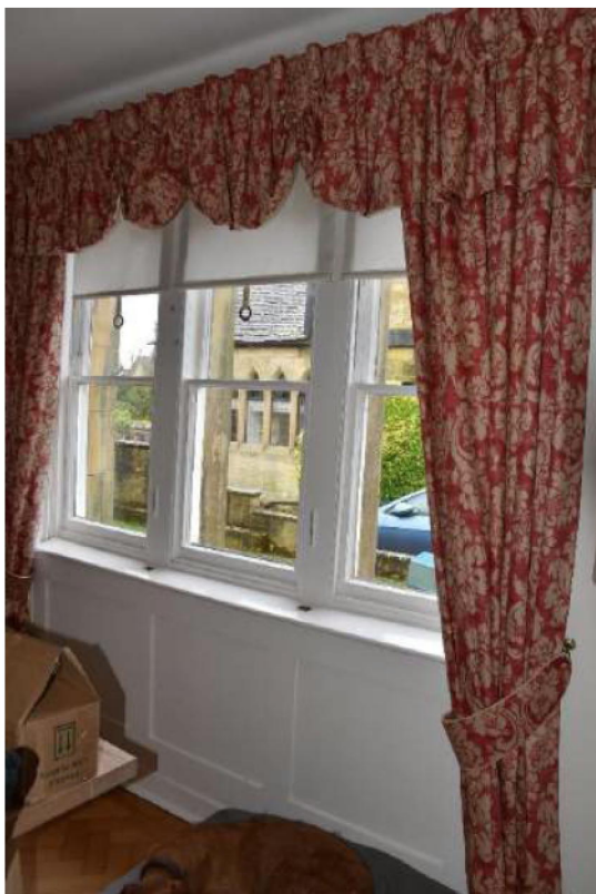
Plate 6: The east ground-floor window on the south elevation, showing the boxing which houses the vertically-sliding shutters.
