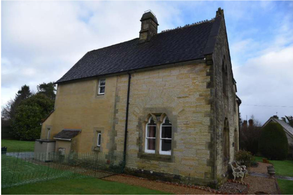
Plate 5: The west elevation.
