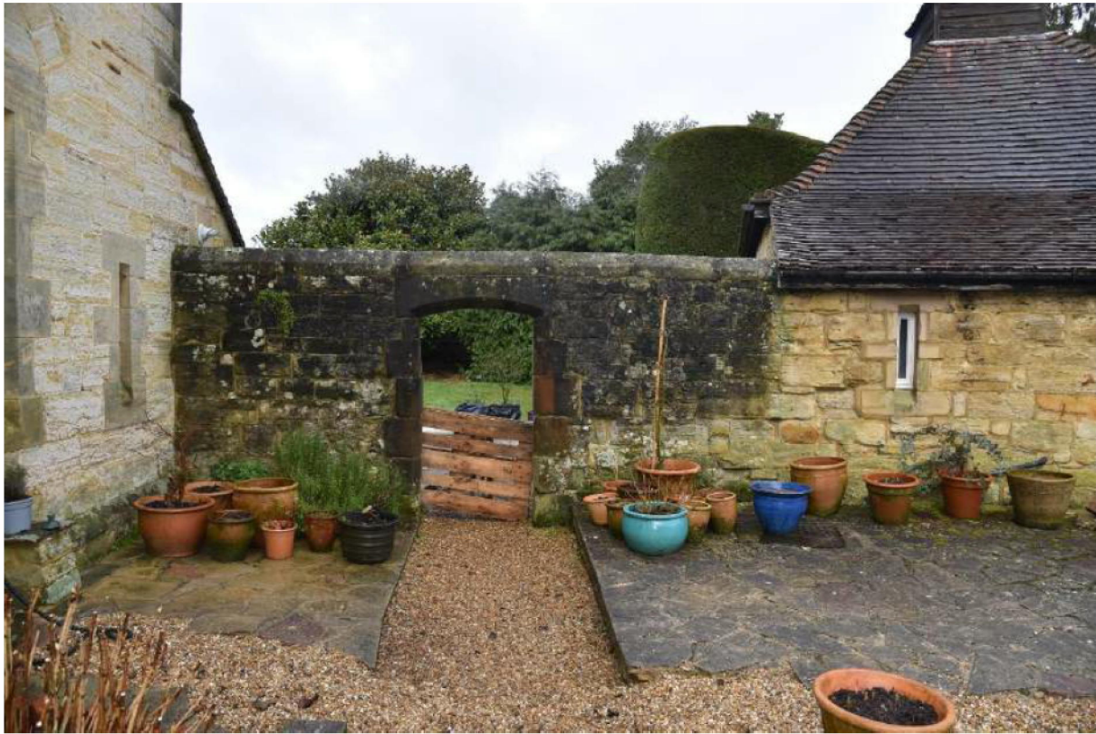
Plate 23: The screen wall, facing north.
