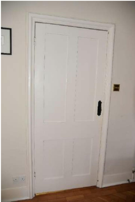
Plate 11: The ground-floor doorway to the service range, with plain four-panel door and typical chamfered architrave.
