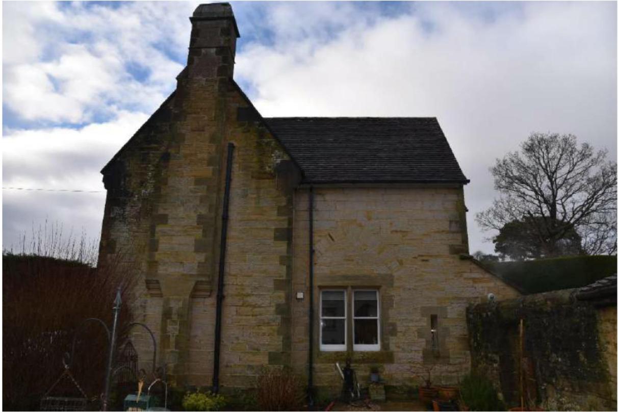
Plate 7: The east elevation.
