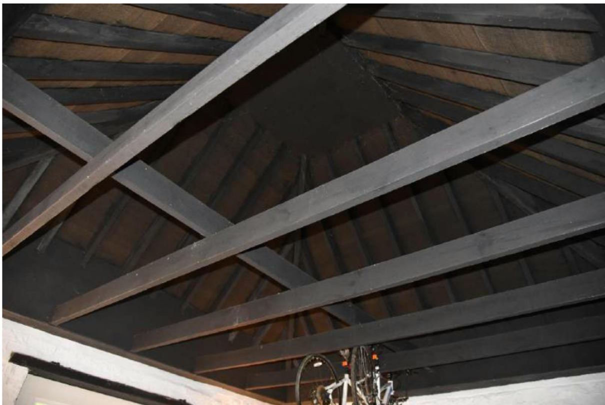
Plate 22: The outbuilding roof structure.
