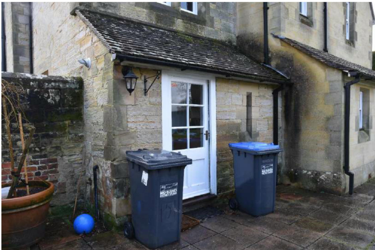
Plate 10: The rear lean-to, facing south-west.
