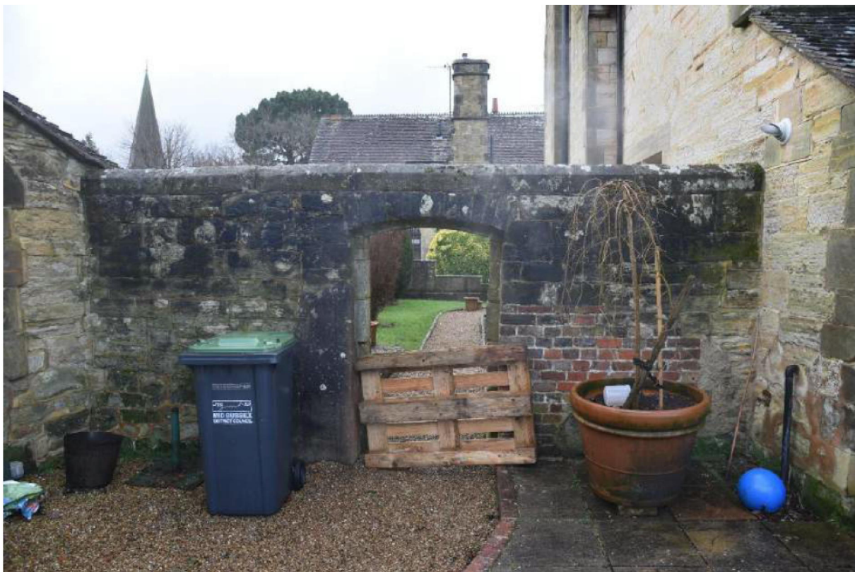
Plate 24: The screen wall, facing south.
