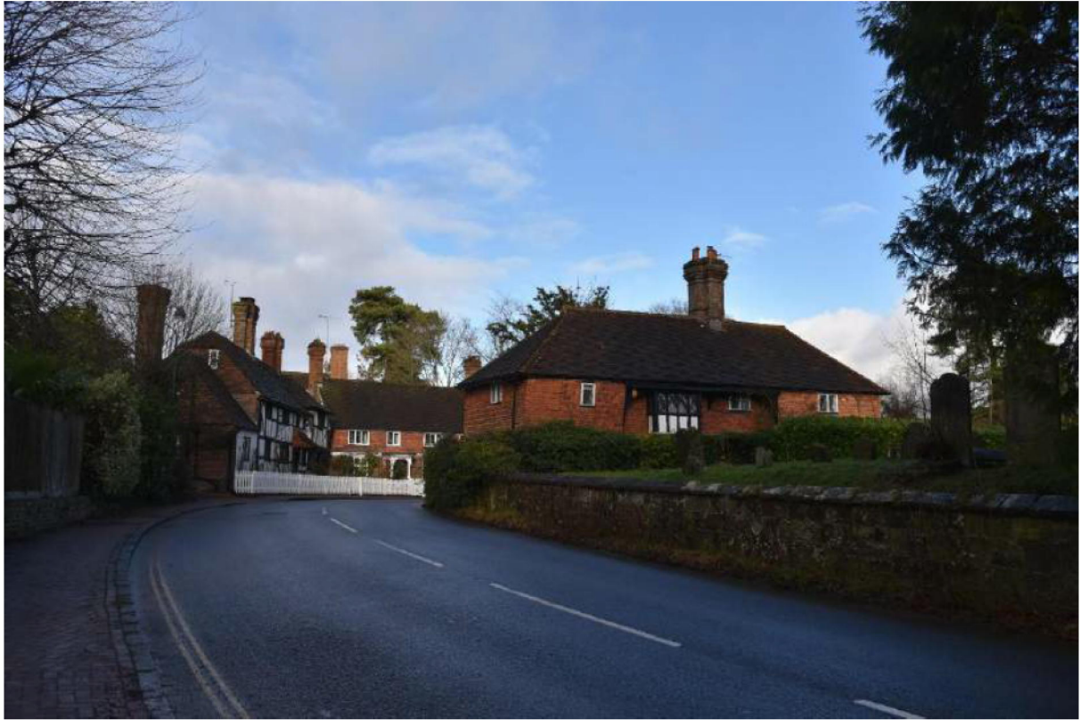
Plate 25: The group of historic buildings at the bend in the road north of the church, facing north.
