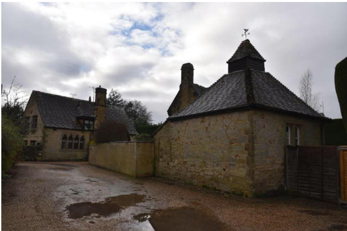
Plate 18: The outbuilding, facing south-west. The former school building can be seen beyond.
