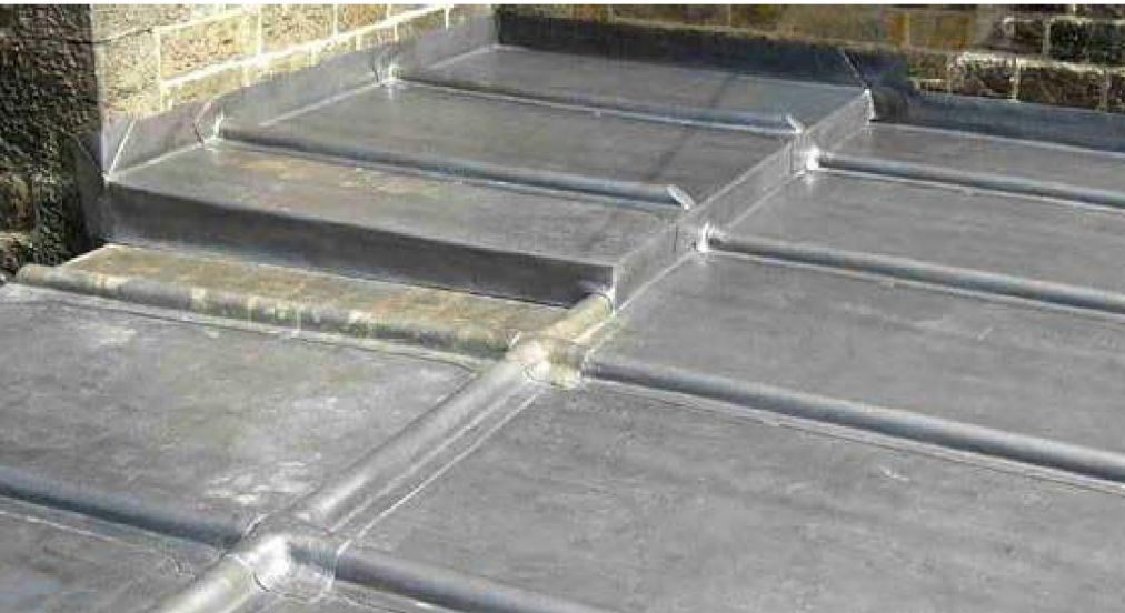
Stepped lead roof to rear and side extensions.
