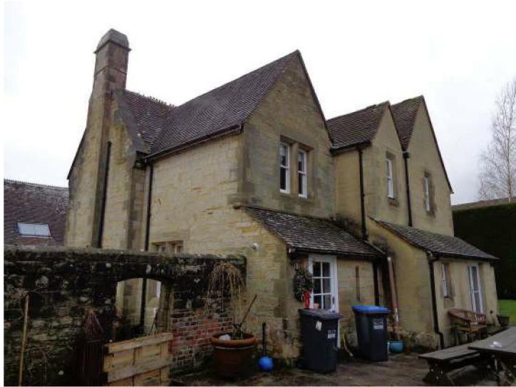
Rear (North Eastern) View of House
