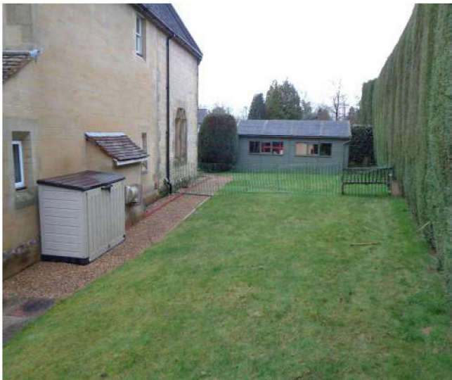
Side view of existing garage.
