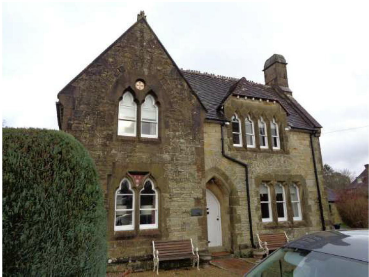
Front (South Western ) View of House
