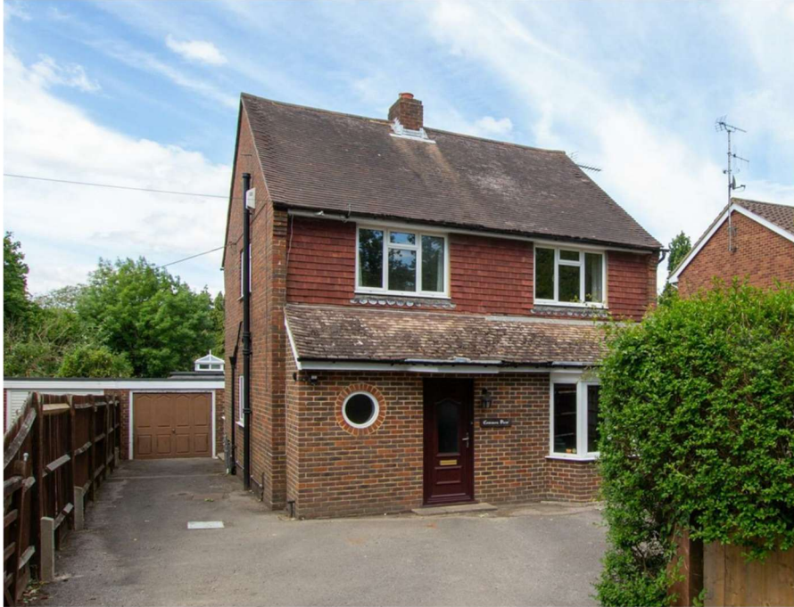
Photograph showing front of the property, location of the small extension to the first floor and front dormer.
