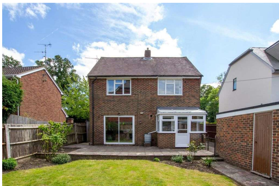
Photograph showing the existing rear garden, conservatory to be removed and neighbouring dwellings.
