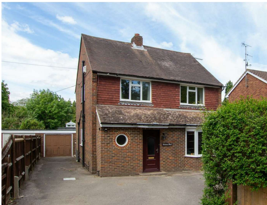
View of the existing building looking South
