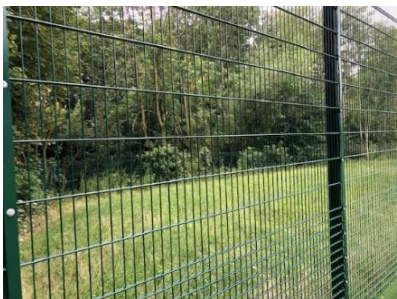
Rigid panel ballstop fencing to perimeter of facility, powder coated dark green to be discrete against a rural backdrop
