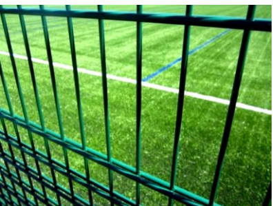
Rigid panel ballstop fencing to perimeter of facility, powder coated dark green to be discrete against a rural backdrop
