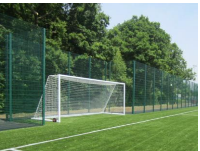
Rigid panel ballstop fencing to perimeter of facility, powder coated dark green to be discrete against a rural backdrop
