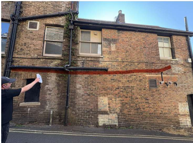
Image to show new position of soil vent pipe from new ladies' toilet facilities located at ground floor level
