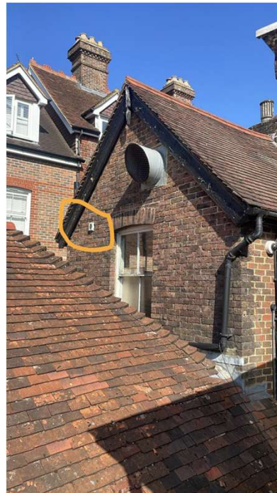
Image to show existing vent grill to be re used for the mechanical extraction to the new ladies' toilet facilities.
