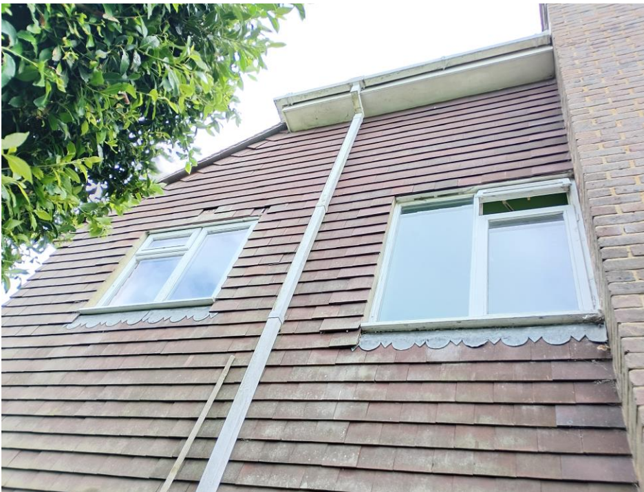
Img.7. Showing broken fascia and gaps in tiling where bats are most likely entering/emerging from.
