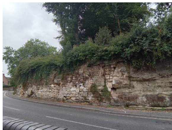
Photo 3: Section of wall denoted W3
