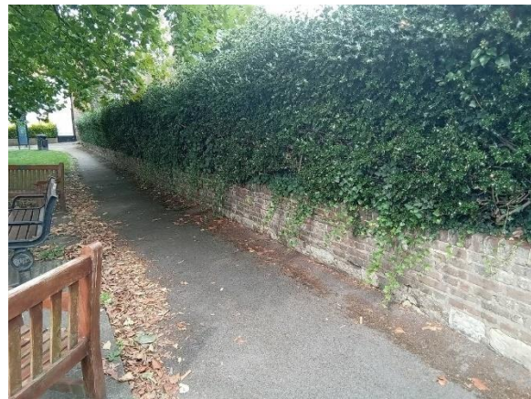
Photo 1: Section of wall denoted W1
