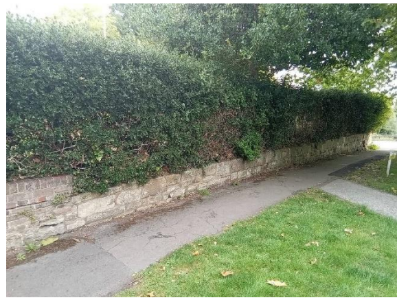
Photo 2: Section of wall denoted W2
