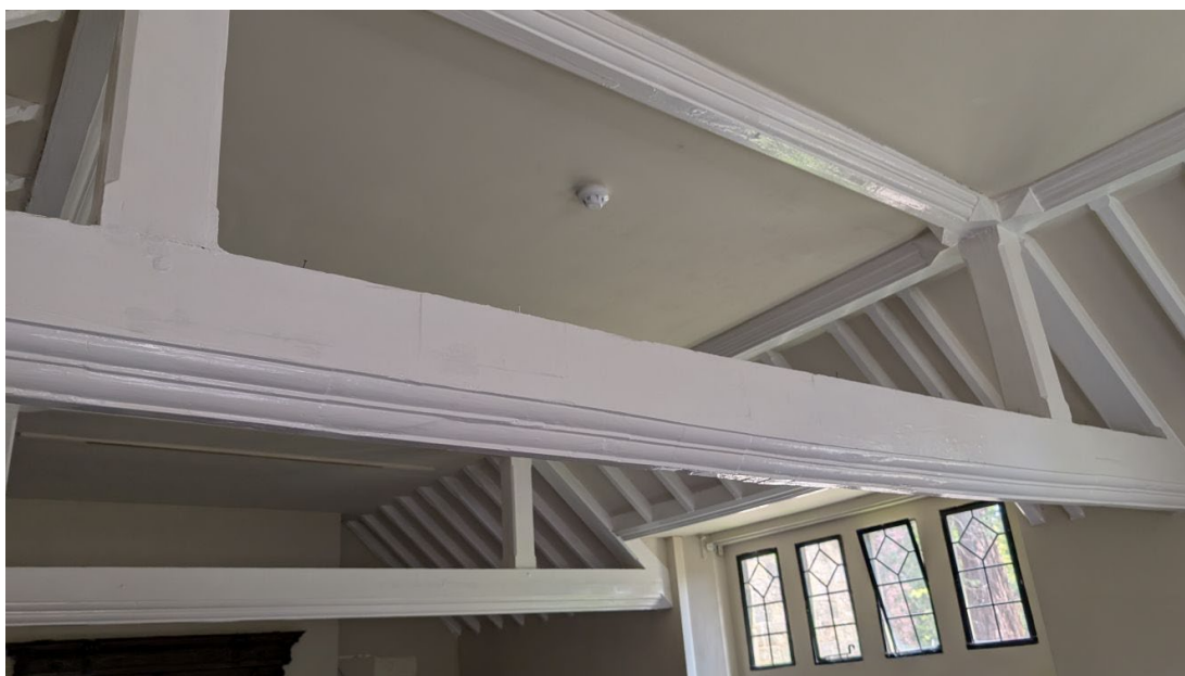
-6 Billiard Room truss.
