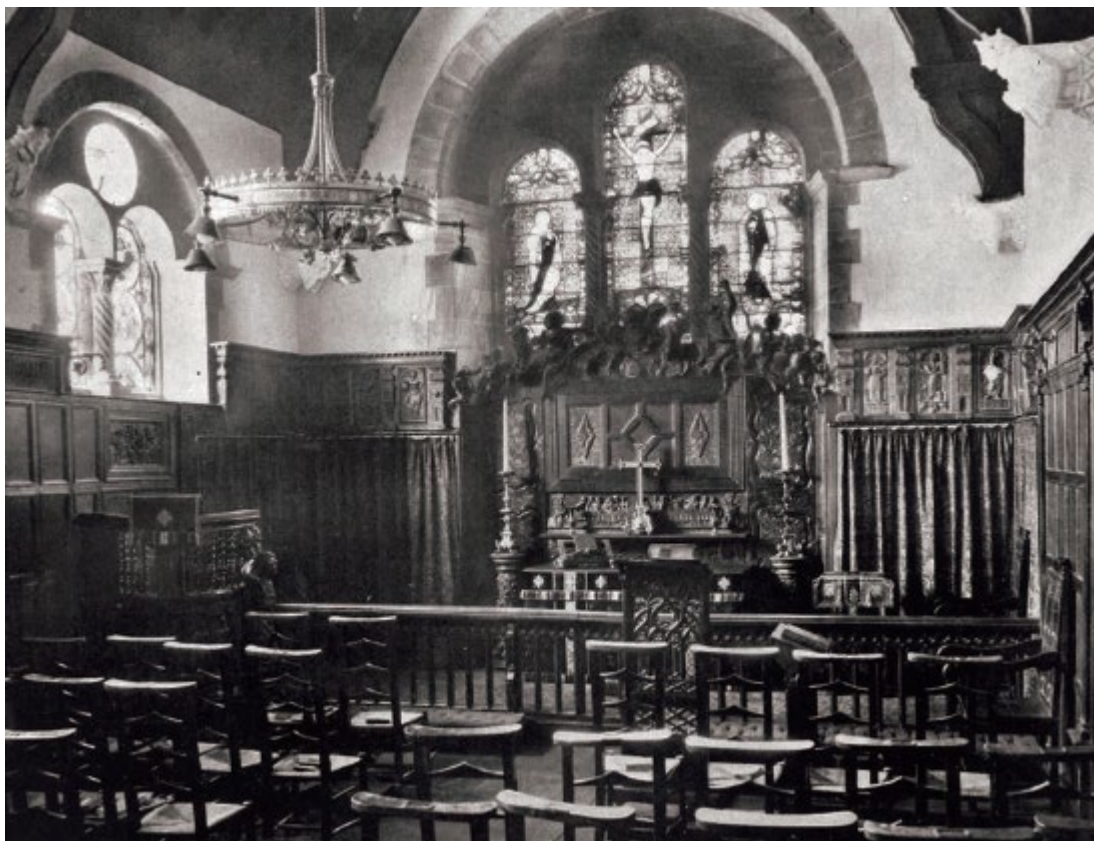
-1 Chapel in the Loder Period, between 1903-1936 (facing east, away from the chimney protrusion)
