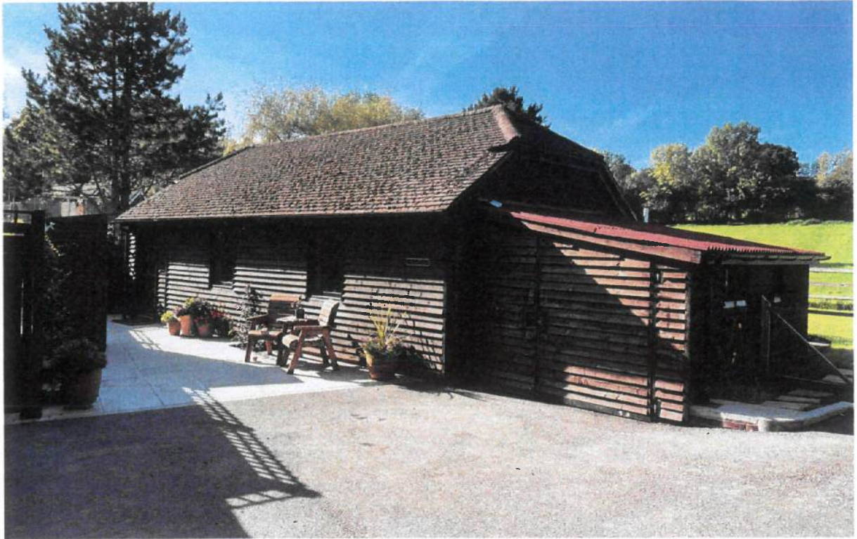
FRONT - ROCK LODGE COTTAGE
