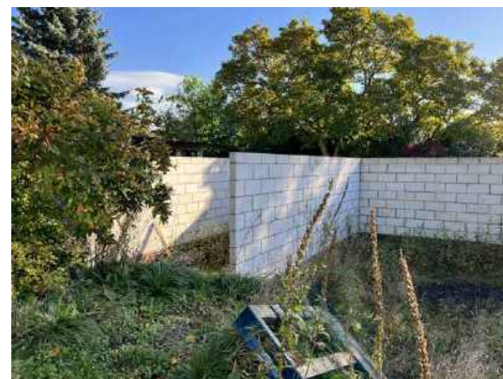
Garage walls constructed
