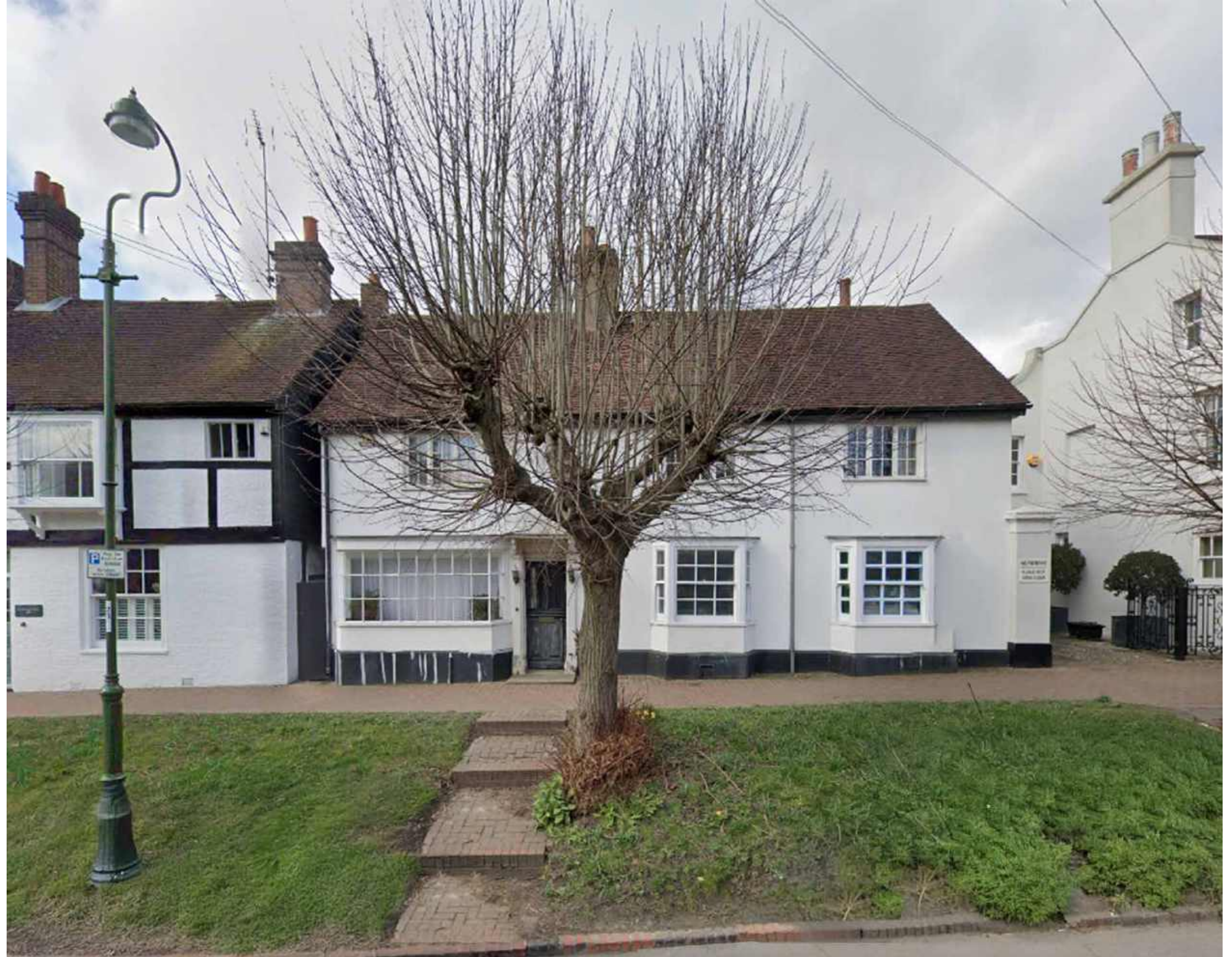
Street view of the facade.
