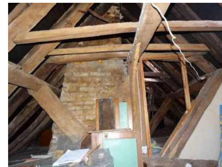
Attic, chimney stack in the background
