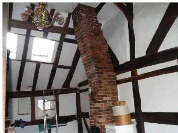
First floor bedroom, chimney stack
