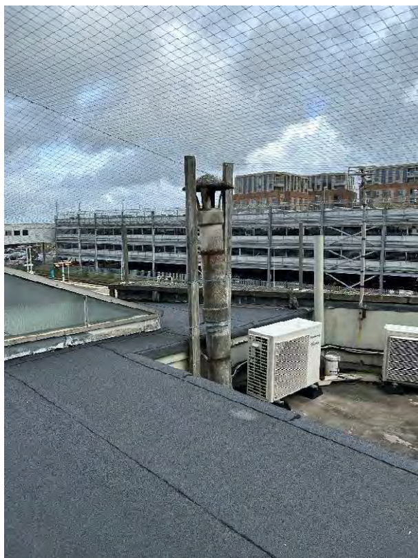
Photo 6. Asbestos cement boiler flue.
