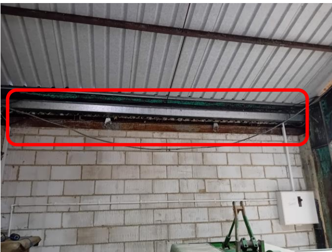
Plate 5: The edge of a corrugated asbestos cement sheet roof to the neighbouring barn is visible on part of the southern elevation of the barn.
