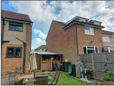
4 - Rear elevation looking to No. 77
