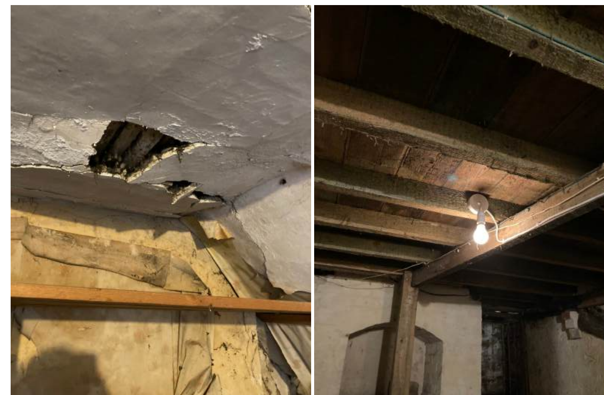
Insulation to be installed to attic rooms (left) and cellar's ceiling (right).
