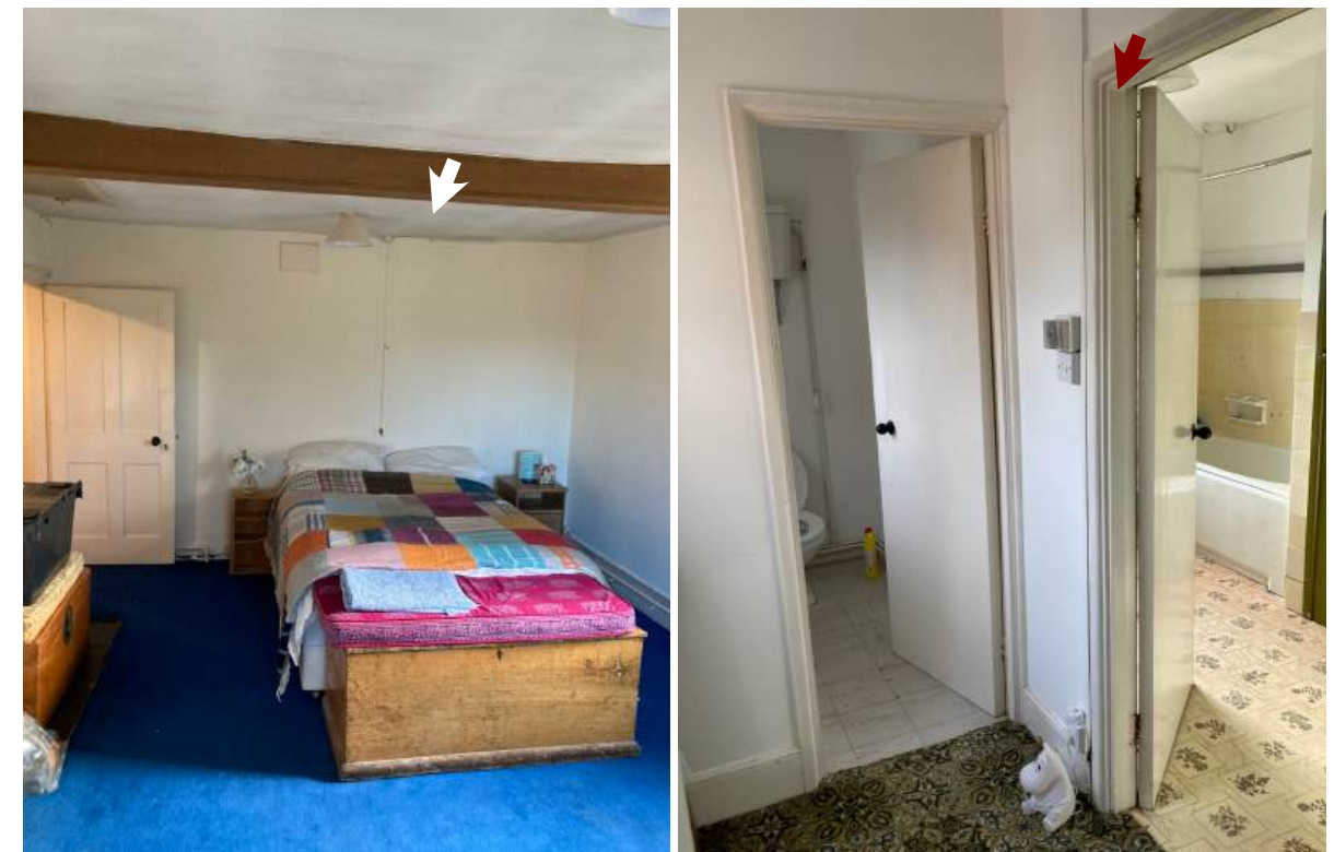
Location of new partition for en-suite (left) and wall between upstairs WC and bathroom to be removed (right).
