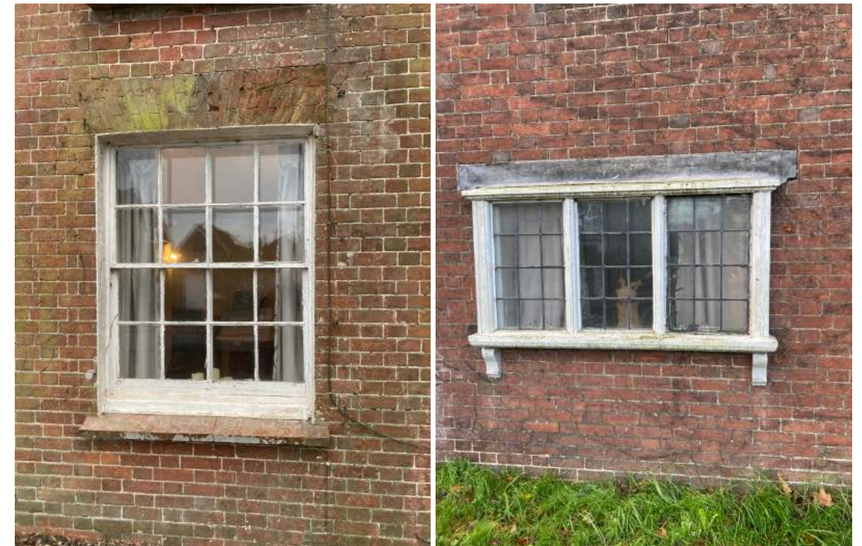
Example of historic windows to be repaired.
