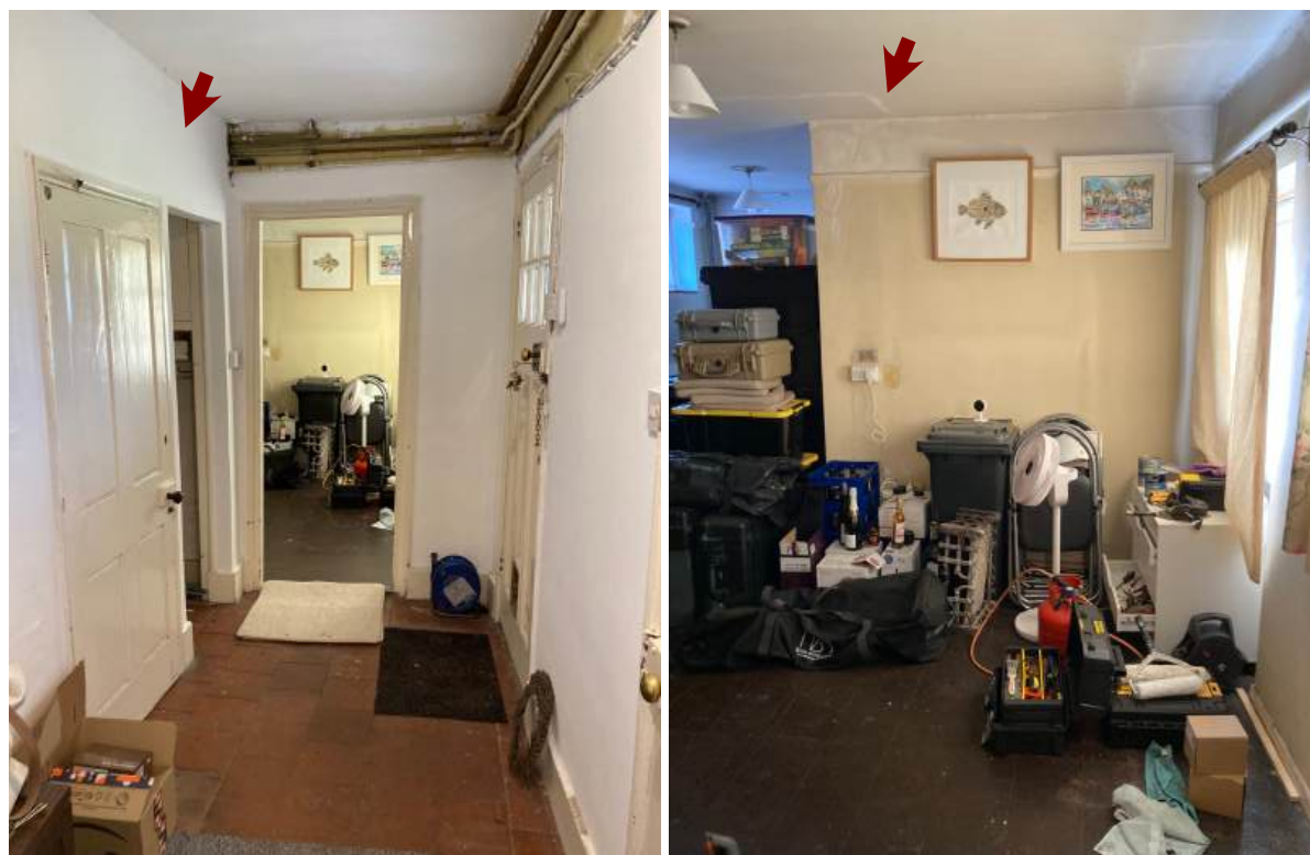
1950s wall to be removed (left) and log store's partitions to be removed (right).
