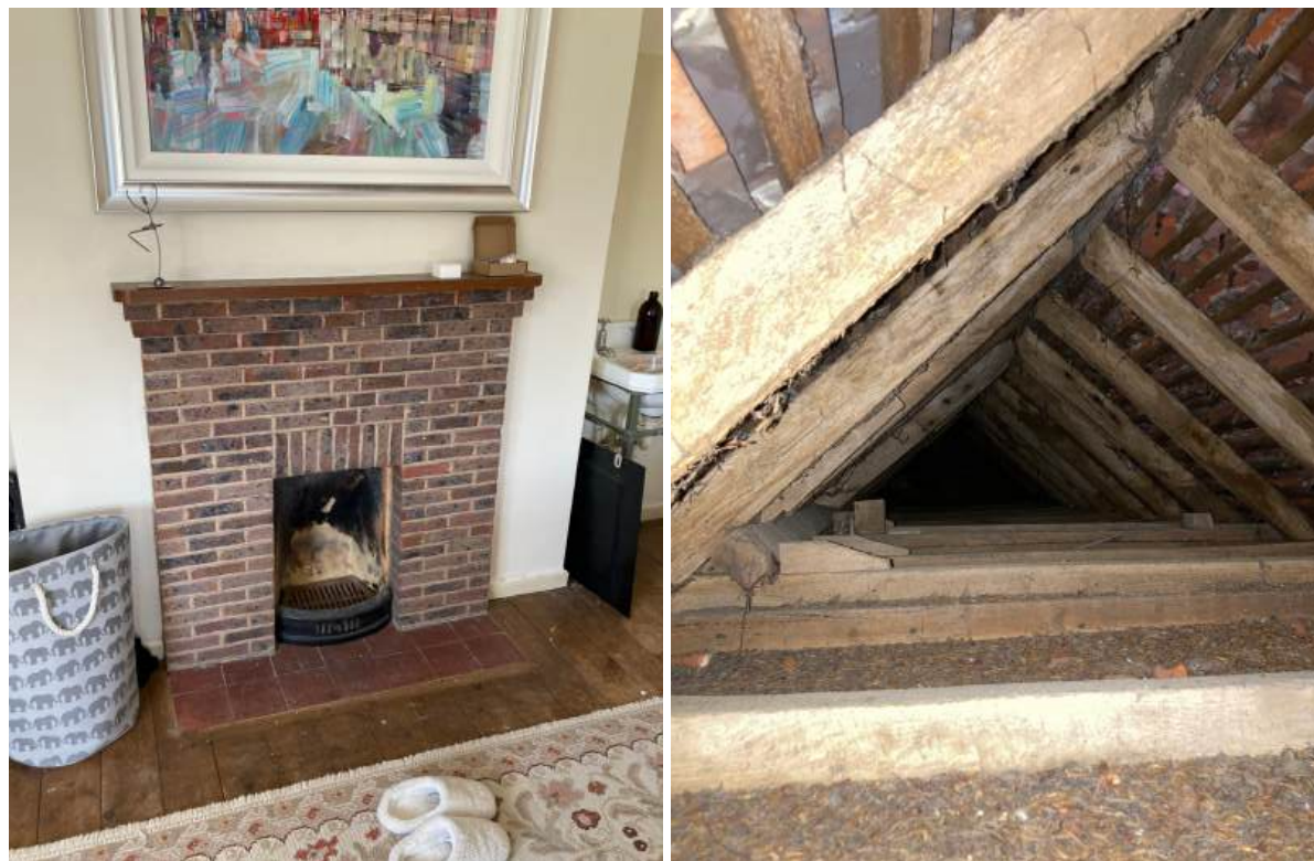
1950s brick insert to be removed (left) and modern collars to be raised (right).
