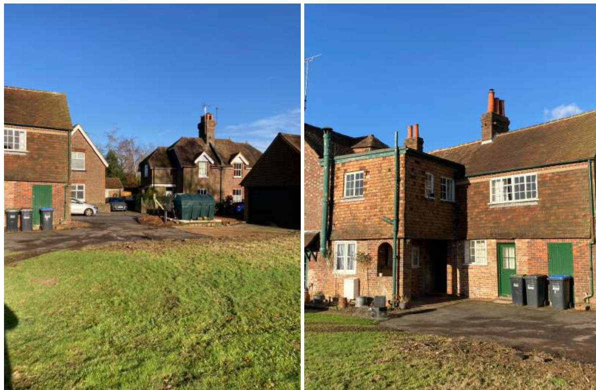
Oil tank to be removed and driveway extended, and location of new gates (left) and patio to be extended (right).
