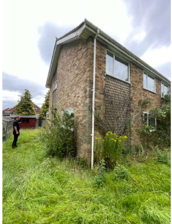
View looking south-east showing side & rear elevation
