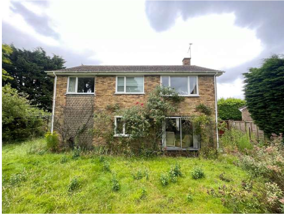
View looking north-east showing side elevation
