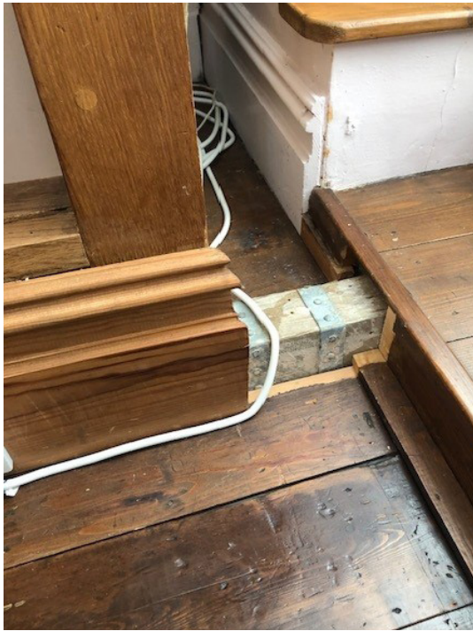
Existing floor joist in floor Revealed
