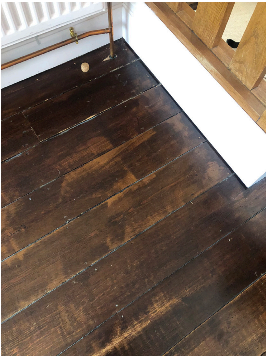
Existing flooring within dining room.
