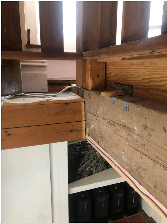
Exposed ground floor structure within basement stairwell.
