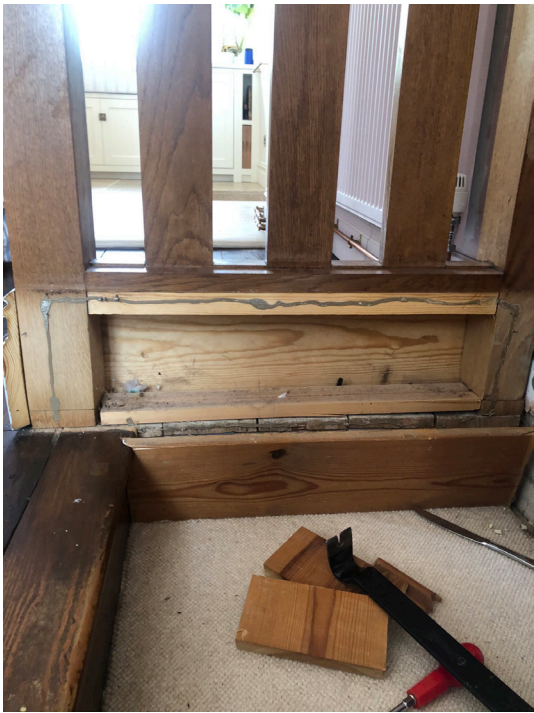
Exposed build up of existing balustrade.
