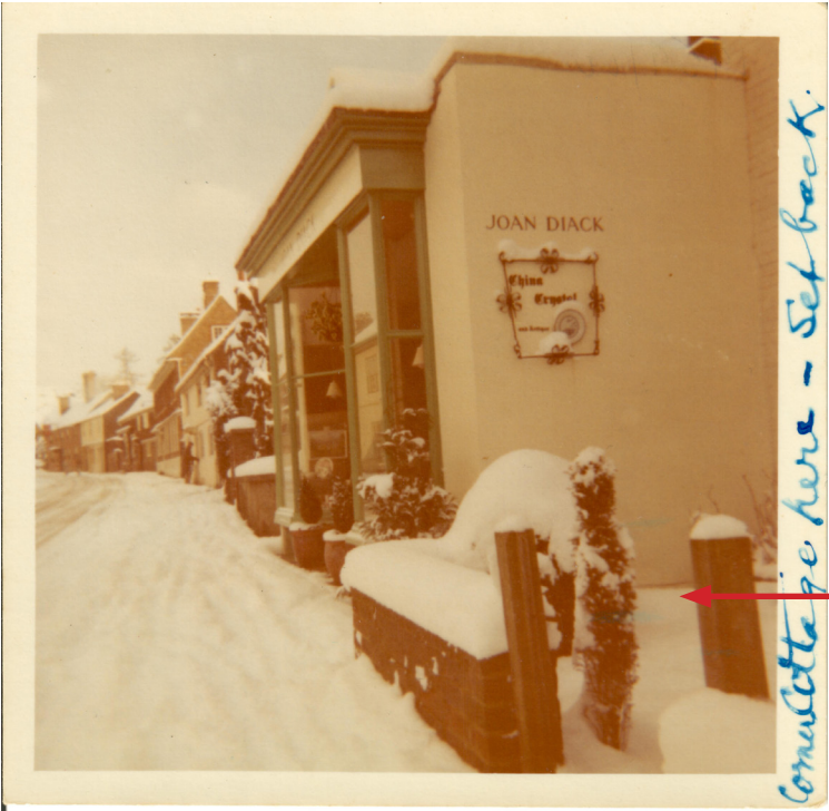
Photo taken between 1959/1960. No evidence of rooflight here.
