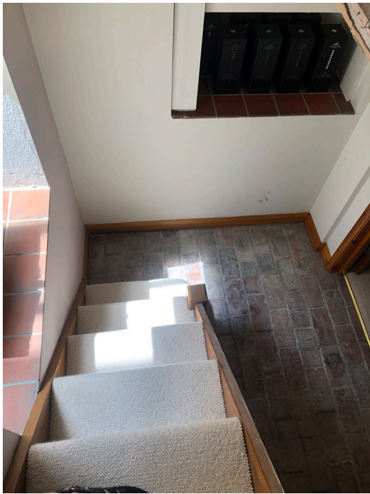
View of basement stair from ground floor.
