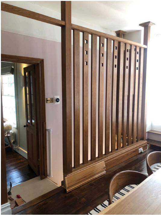
Existing stair balustrade
