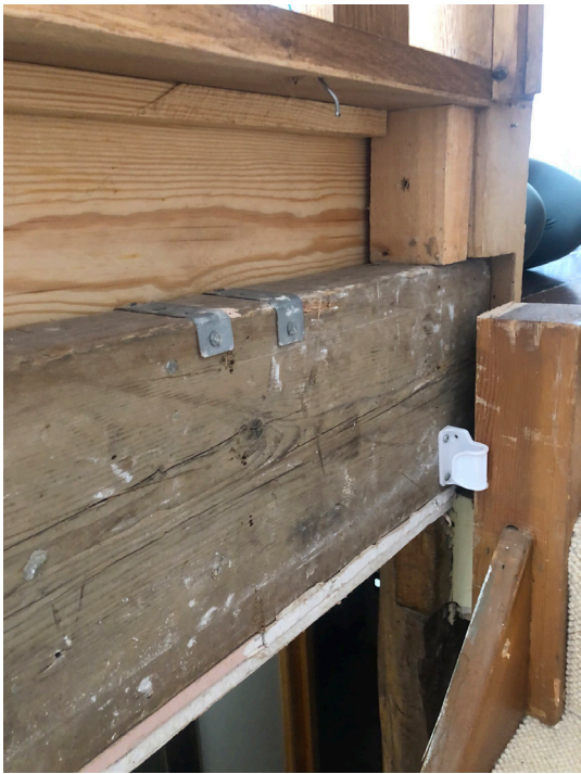
Exposed ground floor structure within basement stairwell.
