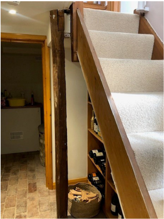
View of basement stair from basement level.
