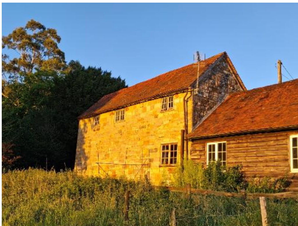
Image No. 01 – B1, northwestern building elevation (SP1).
