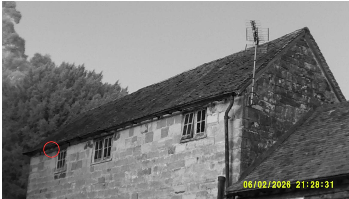
Image No. 05 – B1, northwest aspect. Re-entry at 21:29 on 02/06/2026 between guttering and eaves. Entry point location circled in red.
