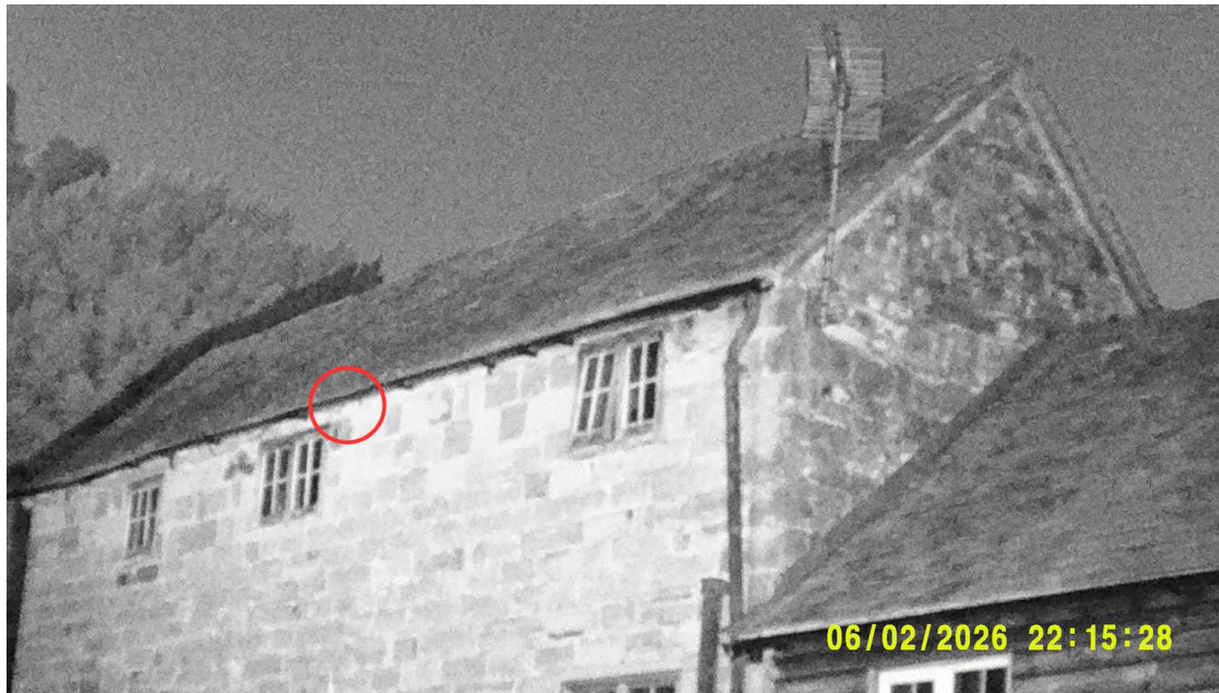
Image No. 07 – B1, northwest aspect. Emergence at 22:15 on 02/06/2026 between guttering and eaves along a central point. Emergence point circled in red.
