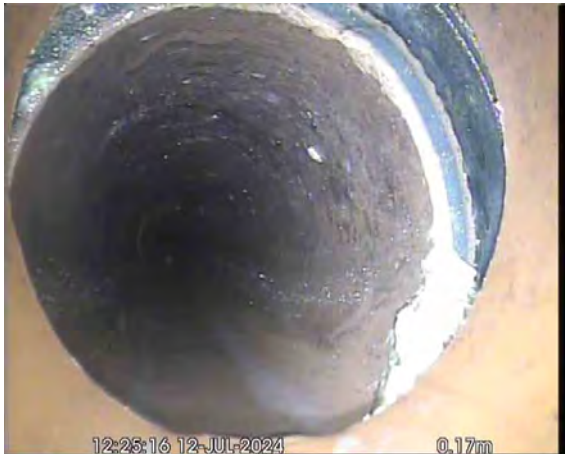
MH5X_e186920a-c72e-48a4-9a6e-cd2a8489a0ab_20240725_094708_970.jpg, 00:00:46, 0.17 m Size changes, new size(s), 100mm high
