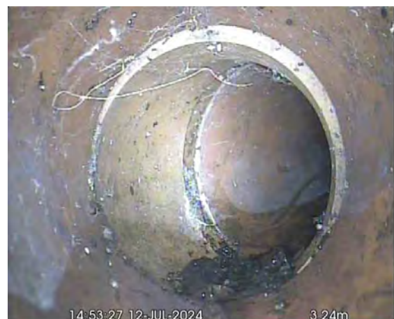
RWDPX_b04b44a7-7c3f-4146-a3f3-0906ec81aae0_20240725_101714_425.jpg, 00:00:58, 3.24 m Line deviates right
