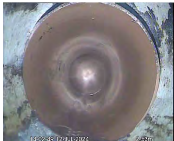
GULLYX_ae4d2037-60f9-42b2-acb6-9ea13a7fabb5_20240725_101346_335.jpg, 00:01:00, 2.53 m Size changes, new size(s), 110mm high
