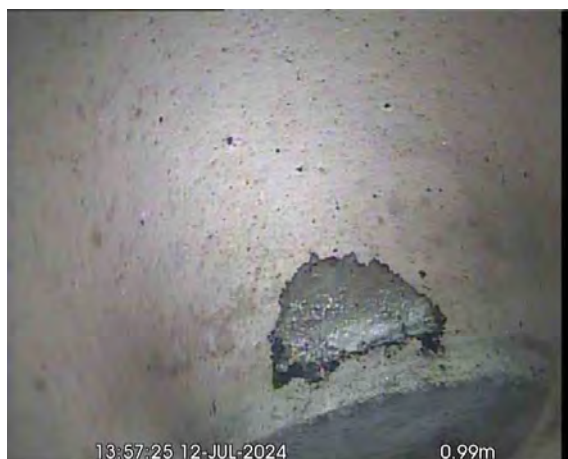
GULLYX_6d63e6bc-a192-46ee-bb28-5b54a1a3e0d8_20240725_095748_794.jpg, 00:00:39, 0.99 m Finish node, gully, reference: GULLY
