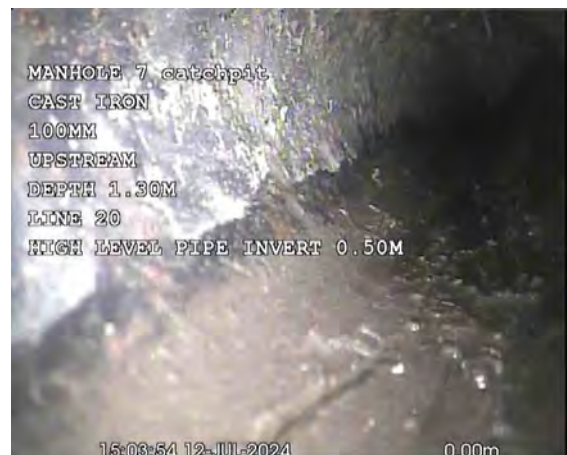
MANHOLEX_057cd0e1-2aeb-4f6e-ab3b-a7fcd1b02335_20240725_102146_679.jpg, 00:00:25, 0.00 m Water level, 0% of the vertical dimension
