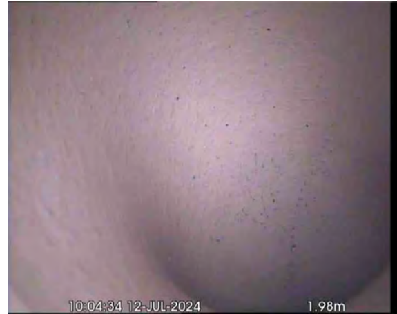
GULLYX_ea8e3b67-ae80-4672-8aa1-6d7696ac026d_20240725_090241_494.jpg, 00:01:10, 1.98 m Finish node, gully, reference: GULLY
