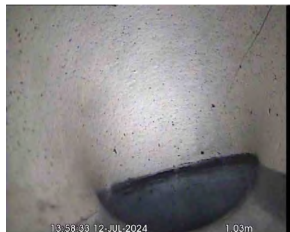
GULLYX_c67647b2-92e2-40c2-a9d7-fb213594d517_20240725_100025_314.jpg, 00:00:28, 1.03 m Finish node, gully, reference: GULLY
