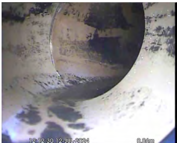
MH4X_047d0d34-fc87-401f-a4c3-3433783703f4_20240725_093918_923.jpg, 00:00:42, 0.06 m Line deviates right
