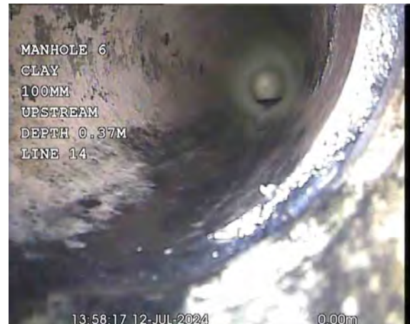
GULLYX_94a6fb12-c47d-431c-aea1-e051d22a5117_20240725_095957_784.jpg, 00:00:12, 0.00 m Water level, 0% of the vertical dimension
