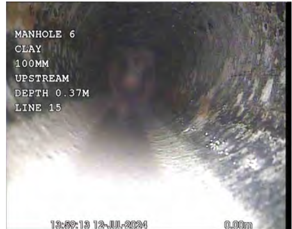
BASINX_b5442afa-9474-4cc7-a6b7-a40489fc90f7_20240725_100946_511.jpg, 00:00:17, 0.00 m Water level, 0% of the vertical dimension
