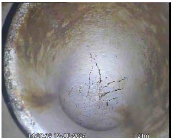
GULLYX_0146e961-7b26-494e-83c0-d047bf27c81e_20240725_101142_978.jpg, 00:00:31, 1.21 m Finish node, gully, reference: GULLY
