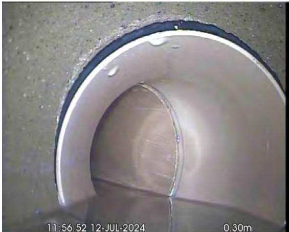
MH2X_b91b3937-c37a-452d-9c54-7c35945f681d_20240725_092617_600.jpg, 00:00:56, 0.30 m Material changes to polyvinyl chloride
