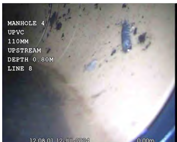
CAPPED OFFX_df637ed9-d0c0-475d-a9b9-2d9c6523196d_20240725_093402_548.jpg, 00:00:39, 0.00 m Start node, manhole, reference: MANHOLE 4 (MH4)
