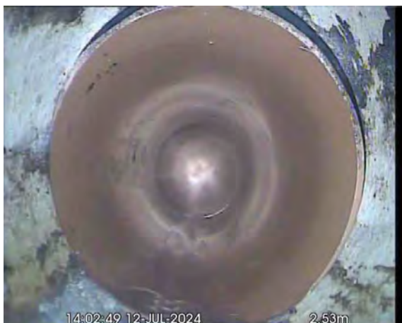
GULLYX_28ba29e2-e34d-48d9-9e89-110dddac1be6_20240725_101336_880.jpg, 00:01:00, 2.53 m Material changes to polyvinyl chloride
