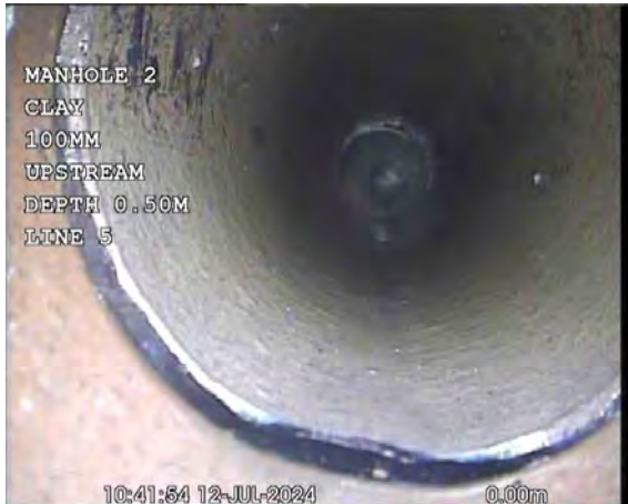
REDUNDANTX_b488a6b2-122d-414b-9b60-81161af3a98e_2 0240725_091111_708.jpg, 00:00:25, 0.00 m Start node, manhole, reference: MANHOLE 2 (MH2)
