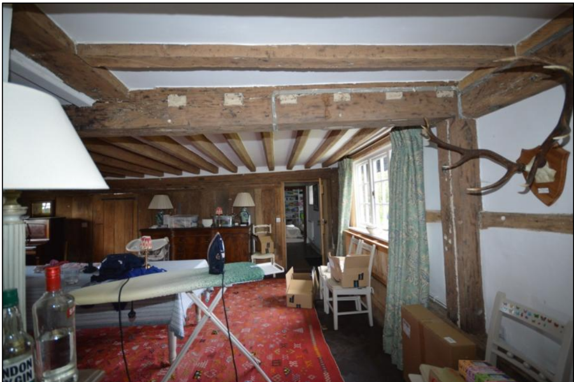
Plate 10: The south side of the inserted cross-beam at the T2 truss, showing the mortises for the original mid-to-late 16 th century floor at the eastern side of the restricted smoke-bay
