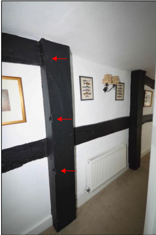
Plate 52: The two principal posts flanking the chimney bay on the south side of the cross-wing, at first floor level, the T6 post includes a series of notches, suggested as fixings for the frame of a doorway/ part of a partition added to the over-length east chamber
