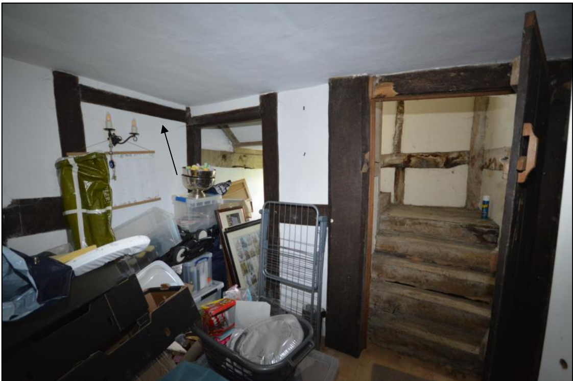
Plate 21: Three original doorways, two on the north side of the cross-wing leading to the closet and stairs within the stair turret and the third, now blocked, providing access to the west chamber (bay 7), indicated by arrow
