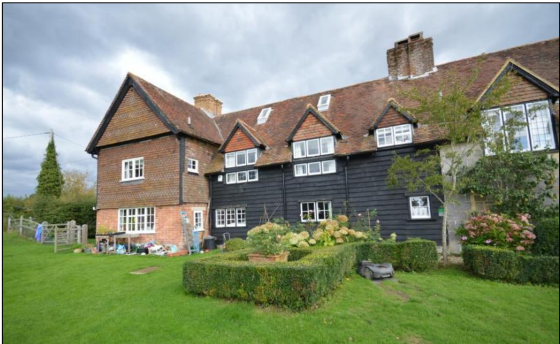
Plate 49: The west side of the property showing the brickwork of the rebuilt ground floor parts of the cross-wing, the weather-boards to the main range and the altered fenestration
