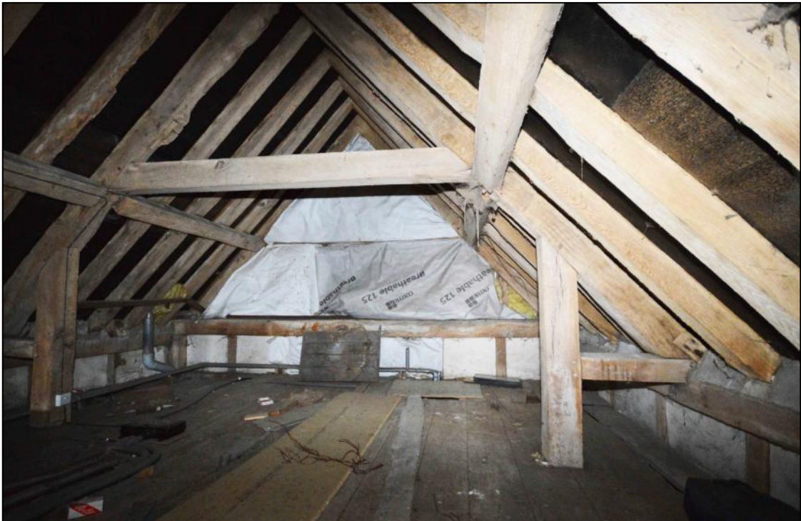
Plate 18: Interior of the attic of bay 7 showing the east-west oriented floorboards
