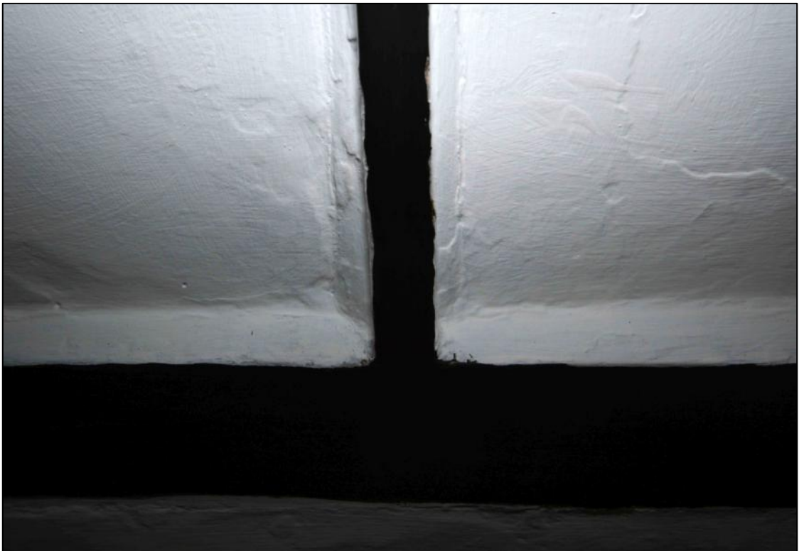
Plate 24: Detail of the ovolo-moulded mullion
