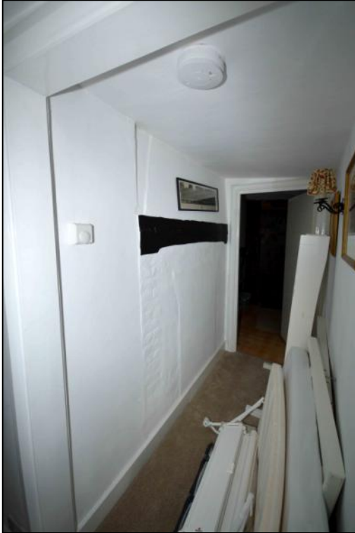
Plate 25: The blocked east fireplace in the multi-flue chimney stack in the cross-wing: note that there are two phases of blocking within the former fireplace
