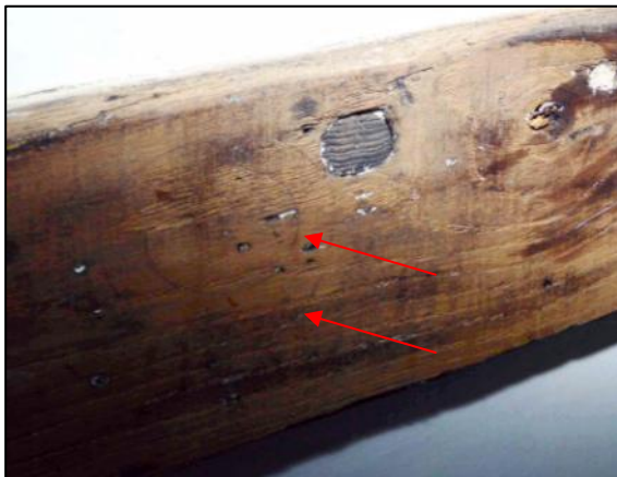
Plate 8: Peg-hole evidence (arrows) for the south jamb of the hall window; note also the double-pegs at the head of the post on its south side, indicative of a doorway head plate or lintel (black arrow). Red square marks the location of the apotropaic mark
