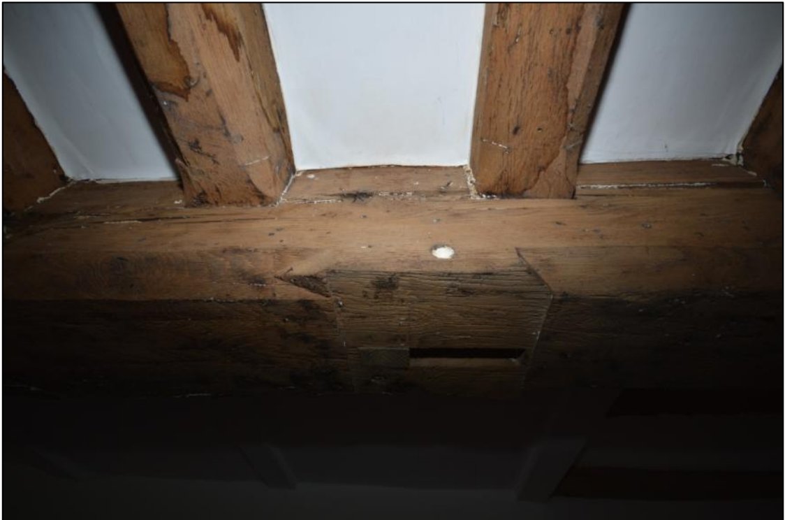
Plate 12: Detail of the chamfer and chamfer stop, and the stud mortise, marking the boundary between the west doorway and the fireplace of the smoke bay
