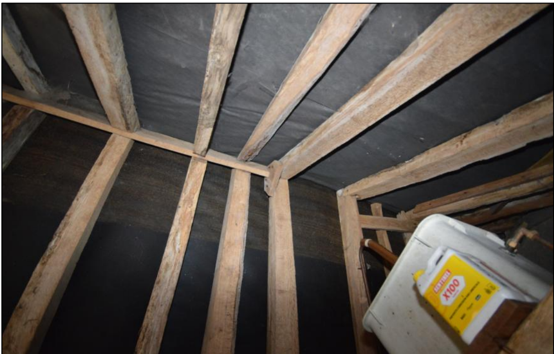
Plate 44: The north end of the roof showing the method of carrying the end of the ridge-board
