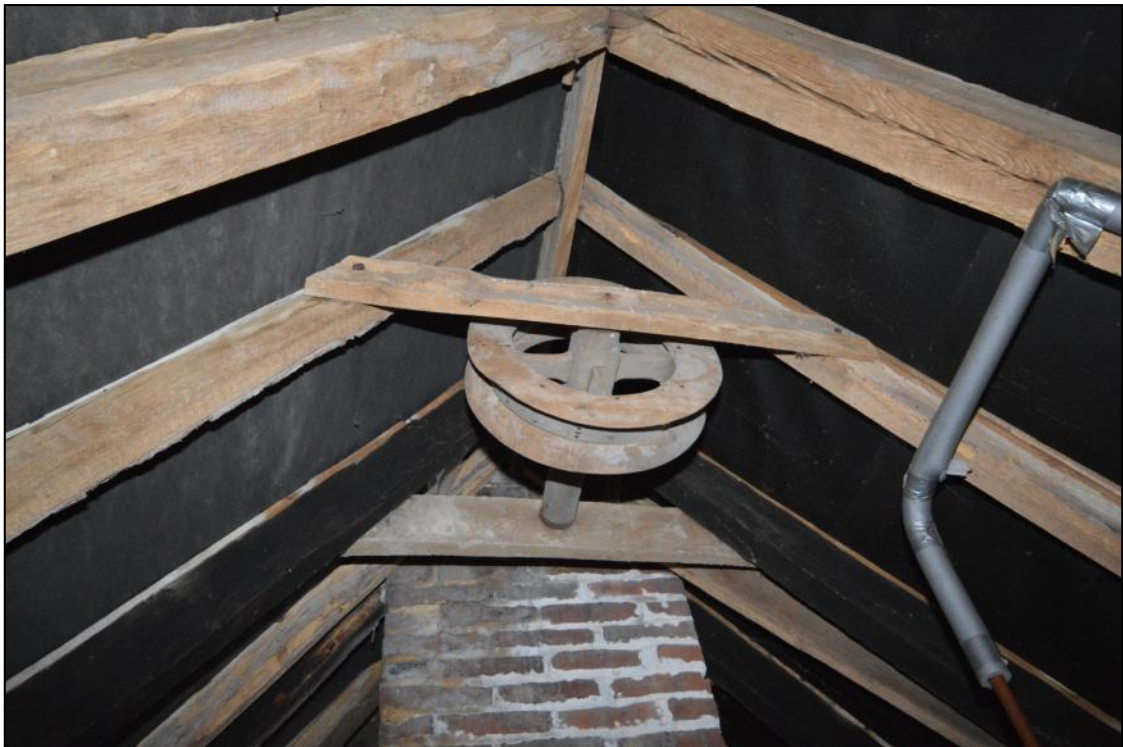
Plate 45: The wooden hoist-wheel nailed to the mid-to-late 18 th century roof in front of the main range chimney stack
