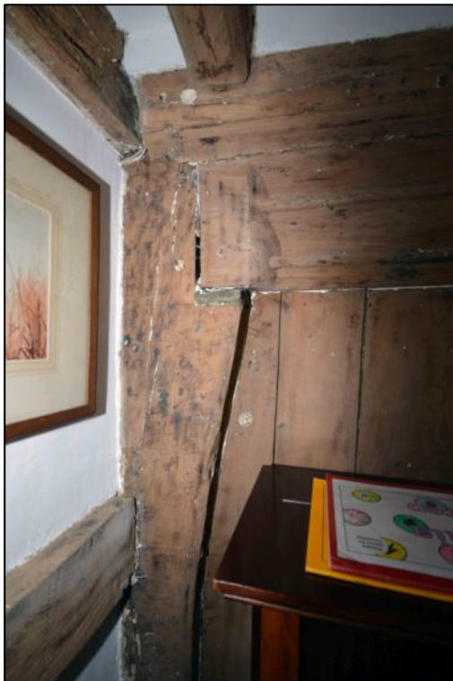
Plate 7: Jowled head to the principal post of the T3 truss where it meets, and carries, the moulded dais beam (west side of the dais partition)
