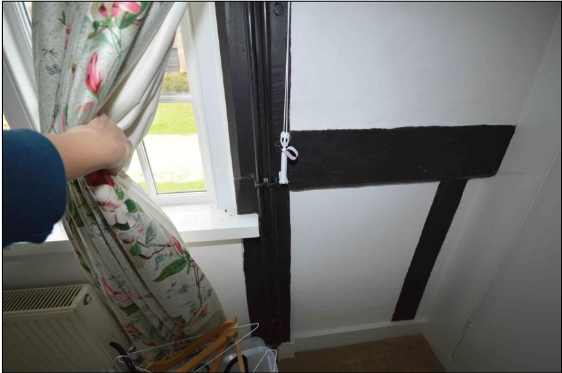
Plate 22: Chamfer and stop detail to the south jamb of the east window in the first floor of the cross-wing, indicating the position of the original window
