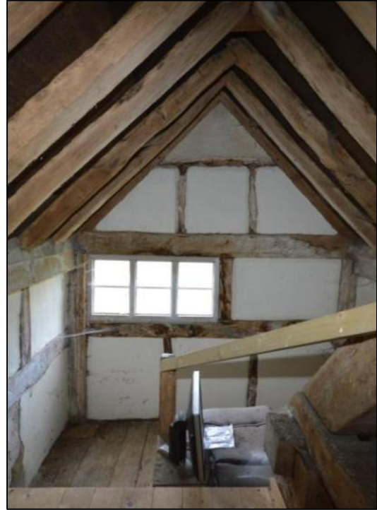
Plate 28: Detail of a queen stud and interrupted tie-beam arrangement and view of the queen-stud truss at the gable of the stair turret
