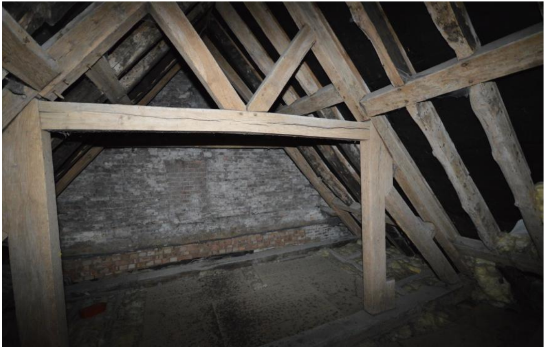
Plate 39: The staggered butt-purlin construction with interrupted rafters and engineered truss over bay 1
