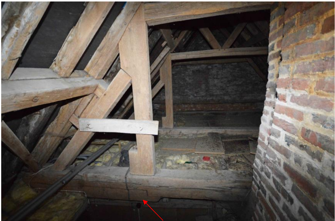
Plate 41: The east side of the T10 truss showing the top of the knee (arrow)
