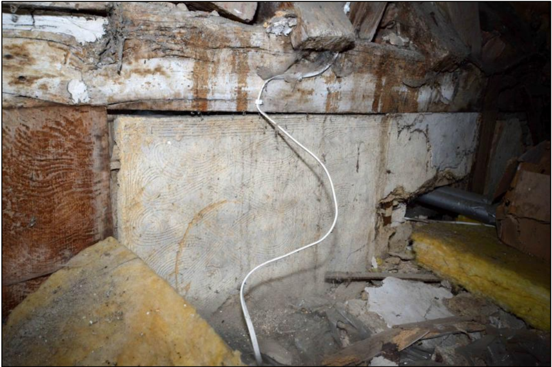
Plate 14: Comb-decorated daub (bay 5) on the south side of the cross-wing visible within the loft over the main range
