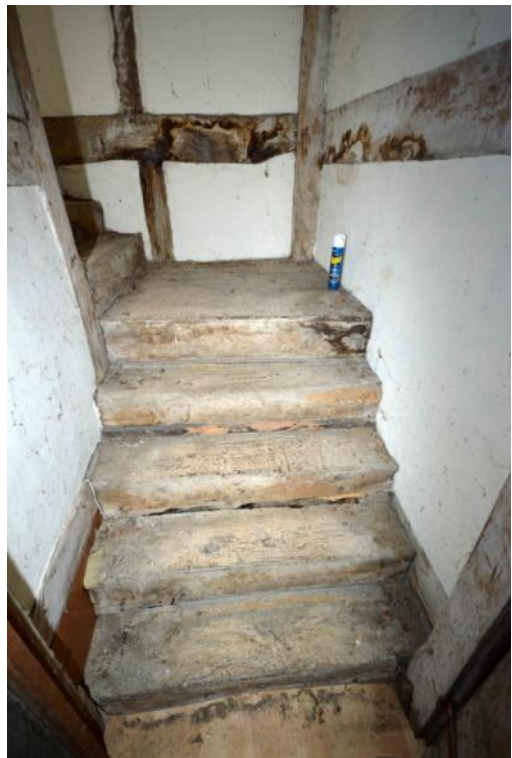
Plate 26: The central well, solid-tread staircase within the stair turret with original cupboard, the door hung on butterfly hinges
