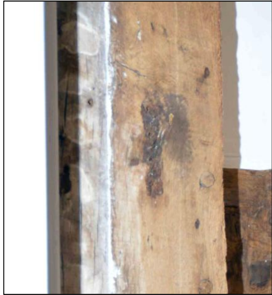
Plate 19: The principal south post of the T6 truss showing the mortise for the head-plate of a doorway (black arrow) and detail of scars and stains left after the removal of a hinge (above)
