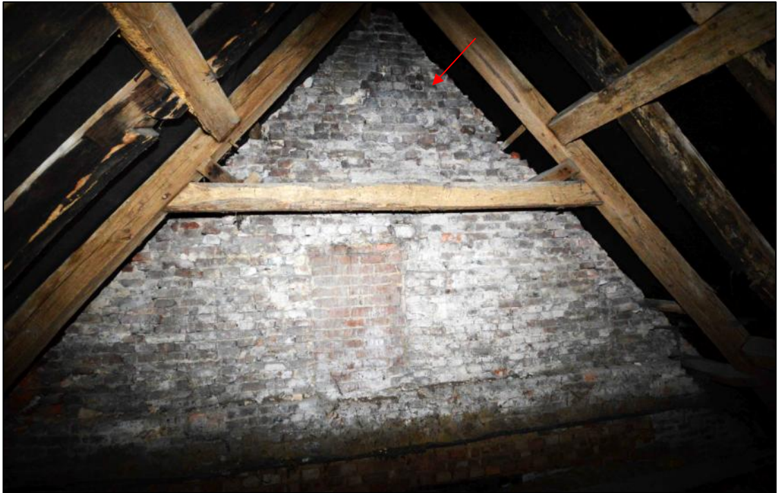
Plate 33: Interior of the south gable with blocked window, note also the off-set for rafters that are no longer in situ (arrow)
