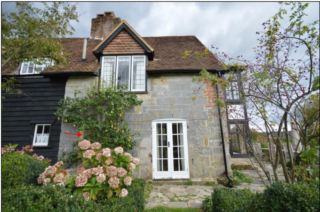
Plate 54: The west side of bay 1, showing the window converted to a doorway and the blocked window to the north of it (arrow)
