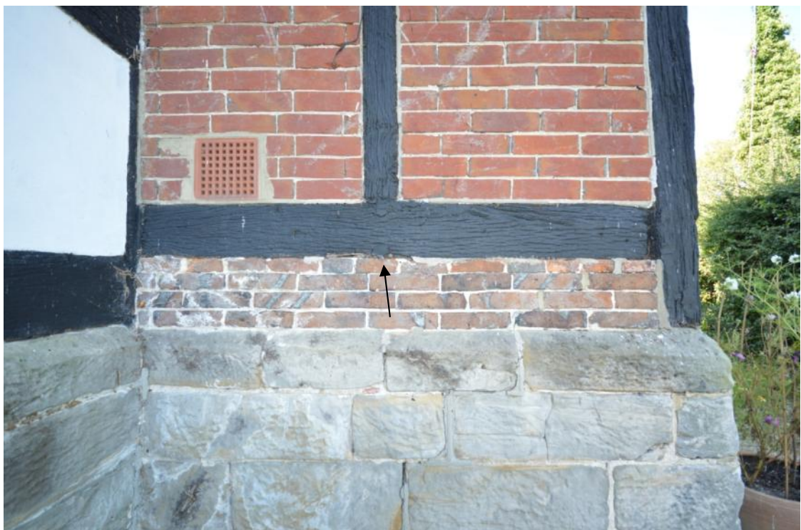
Plate 36: Underbuilt timber frame of the stair tower, with early brick between the new masonry plinth and the timber; note the peg-hole below the stud for a lower stud, removed when the frame was underbuilt (arrow)
