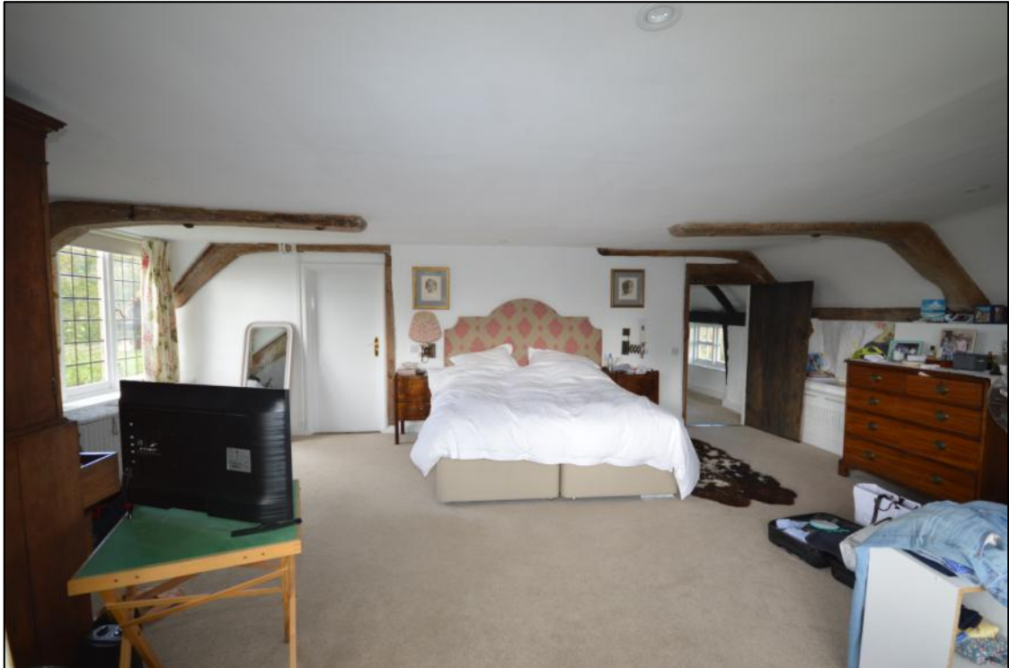
Plate 42: The knee part of the T9 and T10 trusses viewed from the south chamber, supporting the high-set tie-beam and serving as a continuation of the principal rafters
