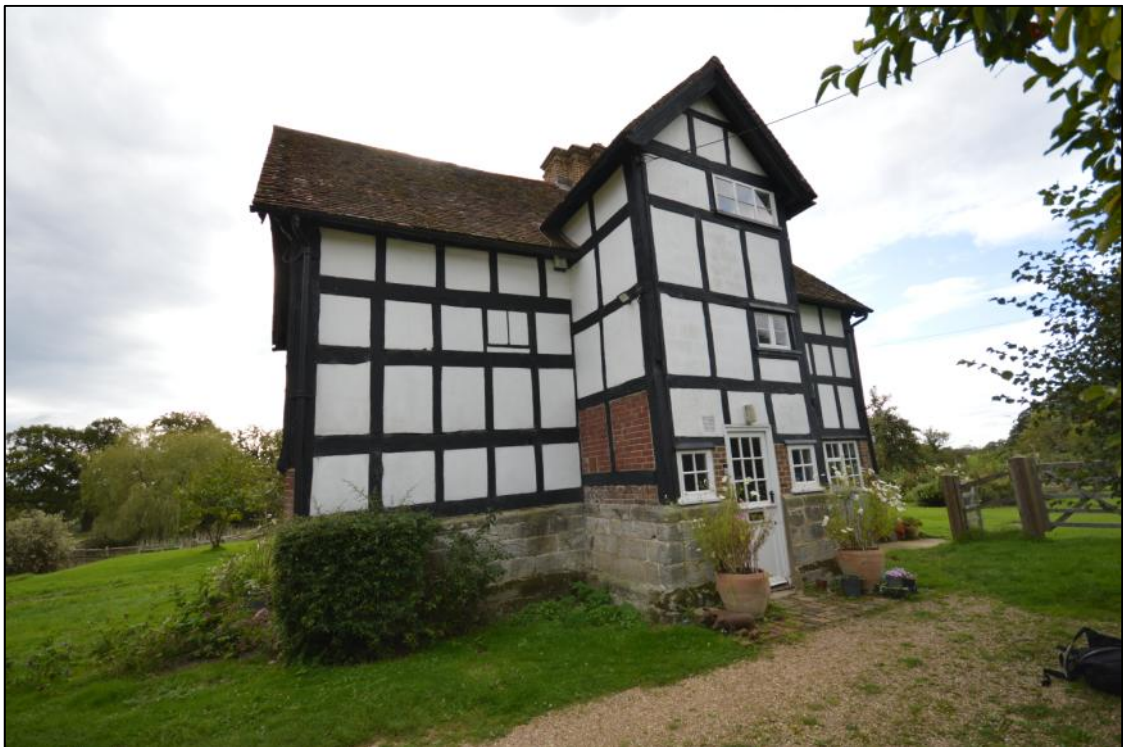
Plate 13: The small-panel framing of the wall construction of the new cross-wing and integral stair turret
