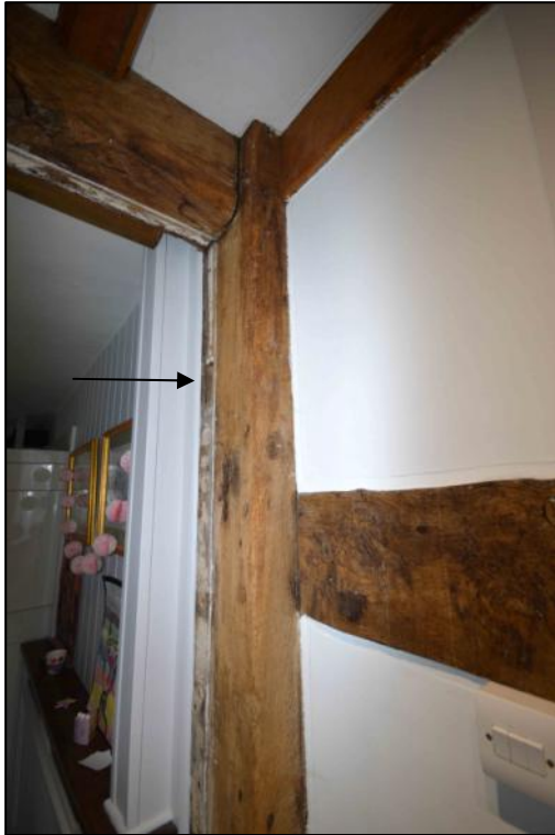
Plate 19: The principal south post of the T6 truss showing the mortise for the head-plate of a doorway (black arrow) and detail of scars and stains left after the removal of a hinge (above)
