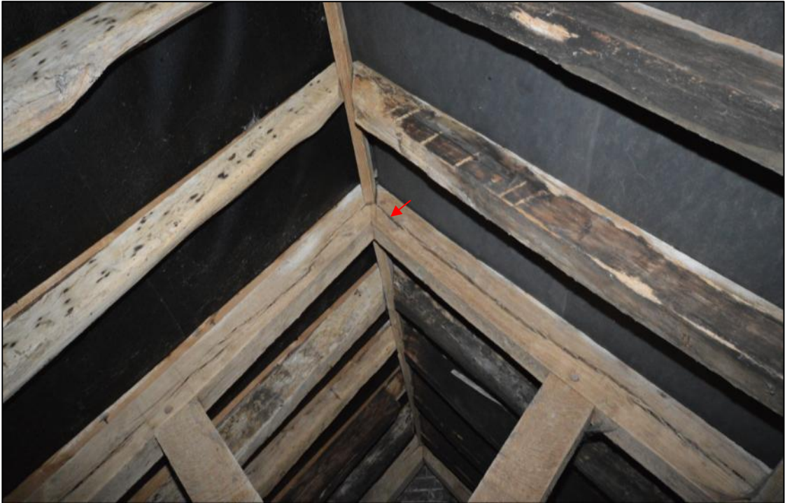
Plate 43: The roof over bay 1 showing the principal rafter and ridge-board arrangement, note the peg for the joint at the apex of the rafters (arrow)
