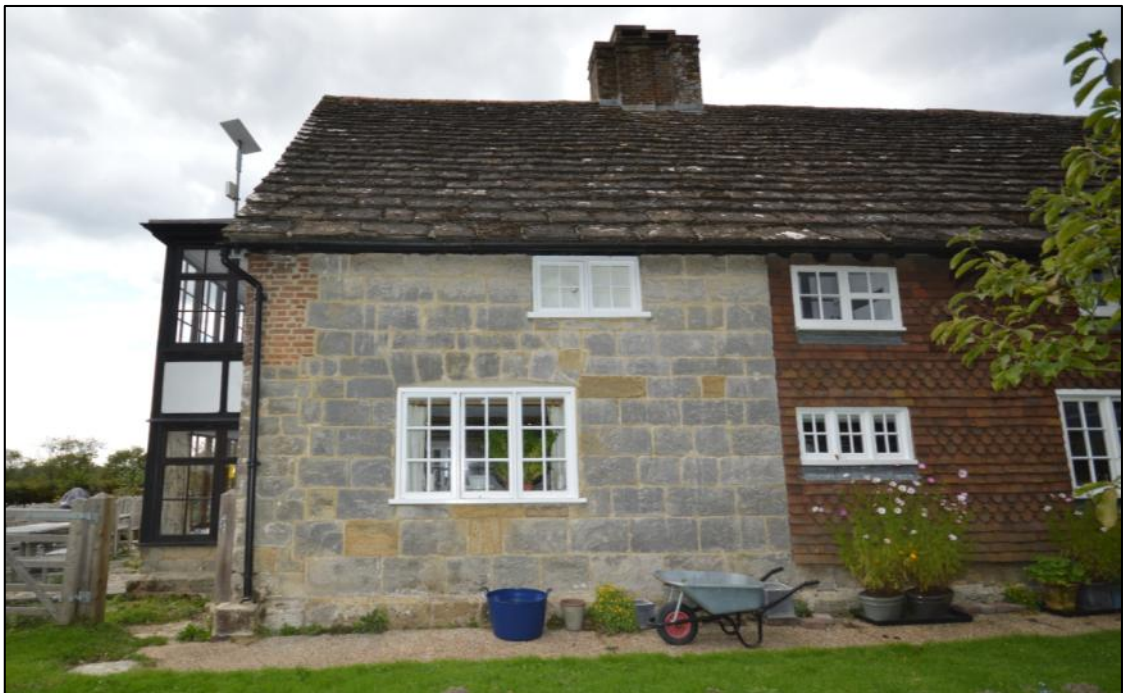
Plate 34: The re-faced eastern elevation of bay 1: note the clear junction between it and the earlier southern end elevation of the building
