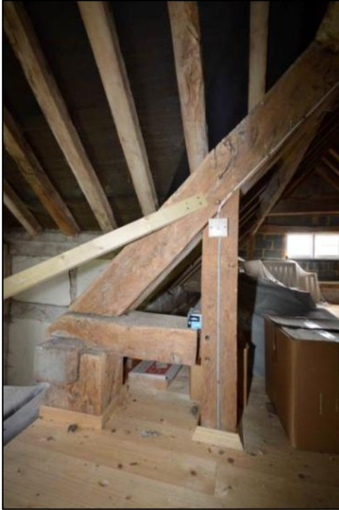
Plate 28: Detail of a queen stud and interrupted tie-beam arrangement and view of the queen-stud truss at the gable of the stair turret
