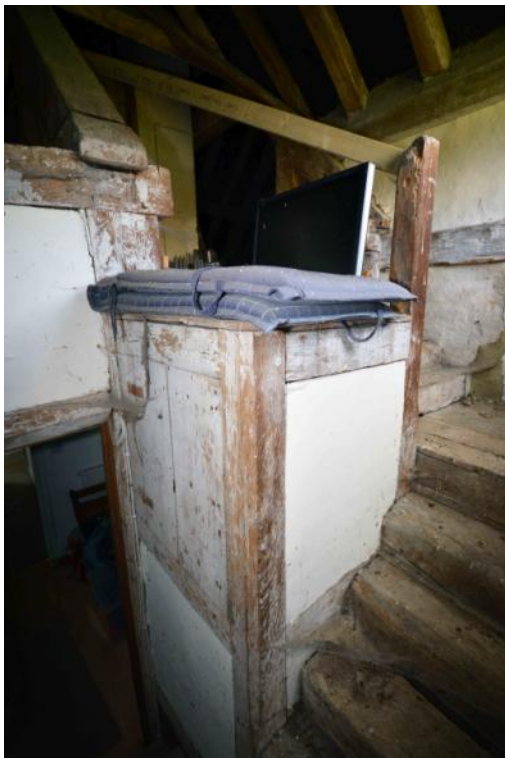
Plate 26: The central well, solid-tread staircase within the stair turret with original cupboard, the door hung on butterfly hinges
