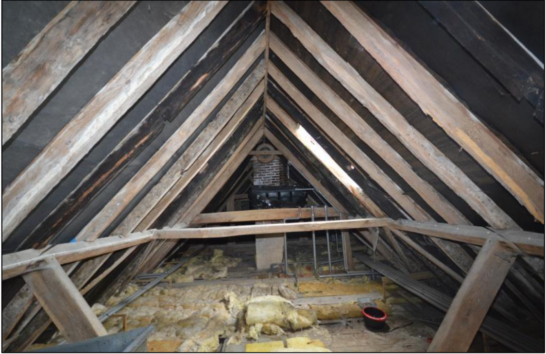
Plate 38: The interior of the roof over the main range with its in-line clasped side-purlins
