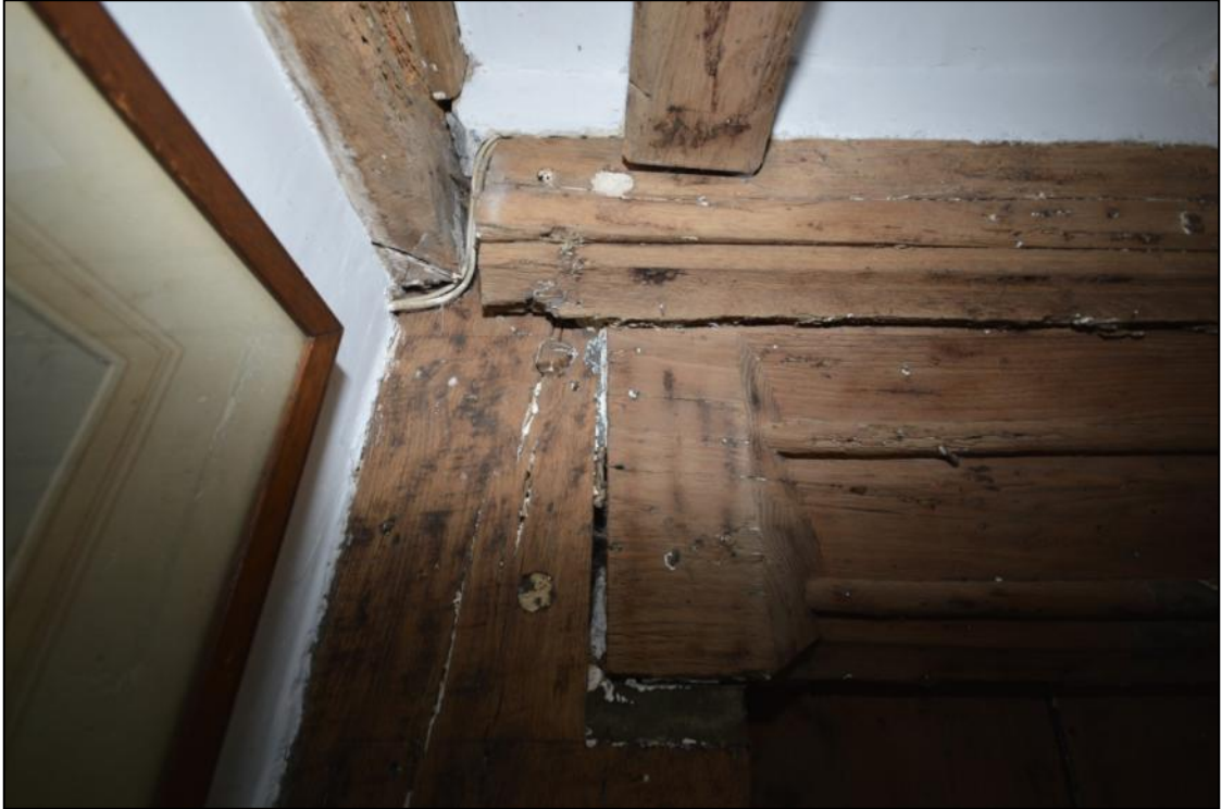
Plate 11: Detail of the western end of the moulded bearer applied over the phase 1 moulded dais beam
