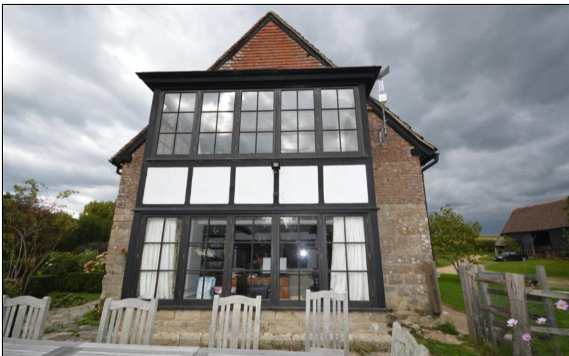
Plate 32: The south end elevation of the main range, the fabric, masonry and brick flanking the late 19 th or early 20 th century bay window is commensurate with a mid-to-late 17 th century origin
