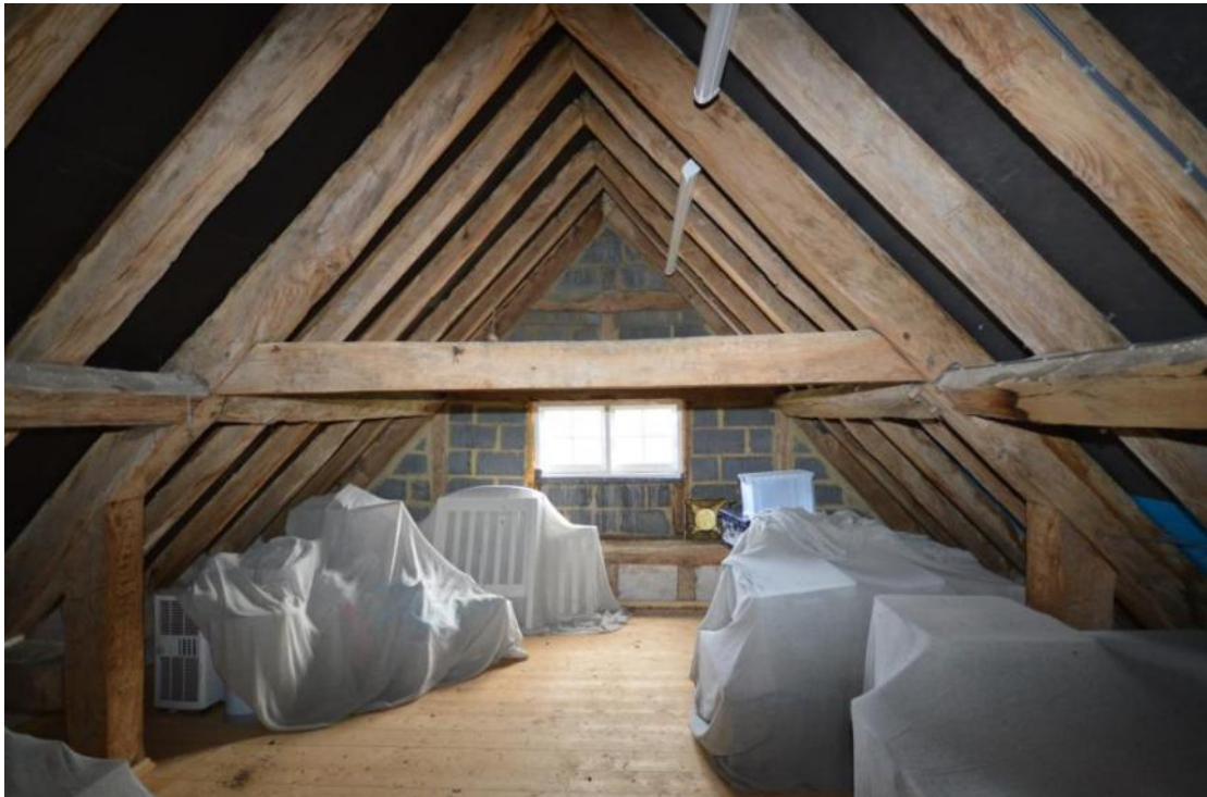
Plate 29: The east roof terminal and general view of the roof
