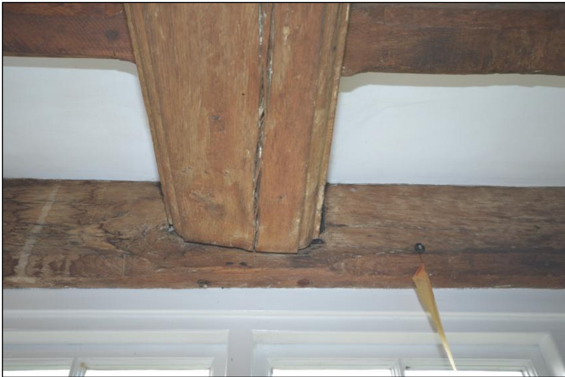
Plate 16: Ovolo moulded girder supporting the first floor in bay 7
