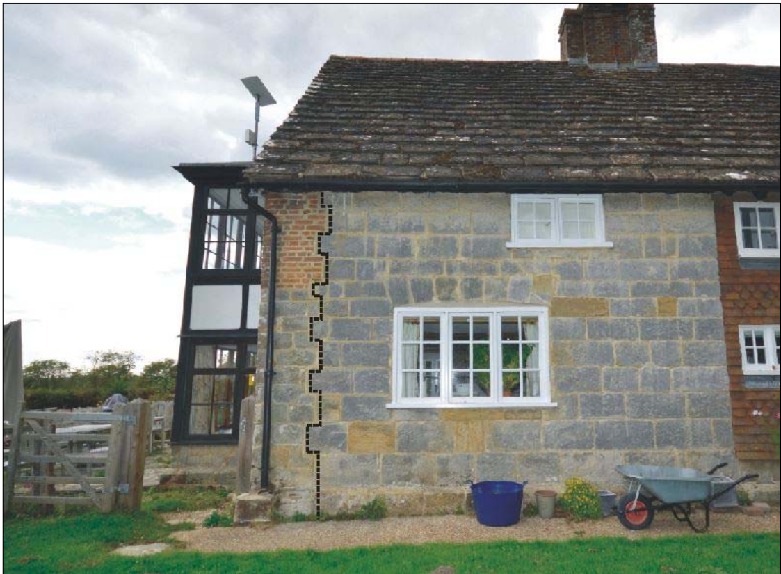
Plate 35: The clear junction between the earlier south end and the re-faced east elevation, compare with Plate 28 above
