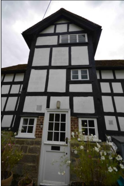
North side of turret showing pressure marks for block-work infill
