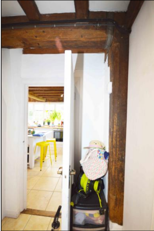
Plate 20: The doorway at the north side of the T7 partition truss, complete with moulded detail in the principal post
