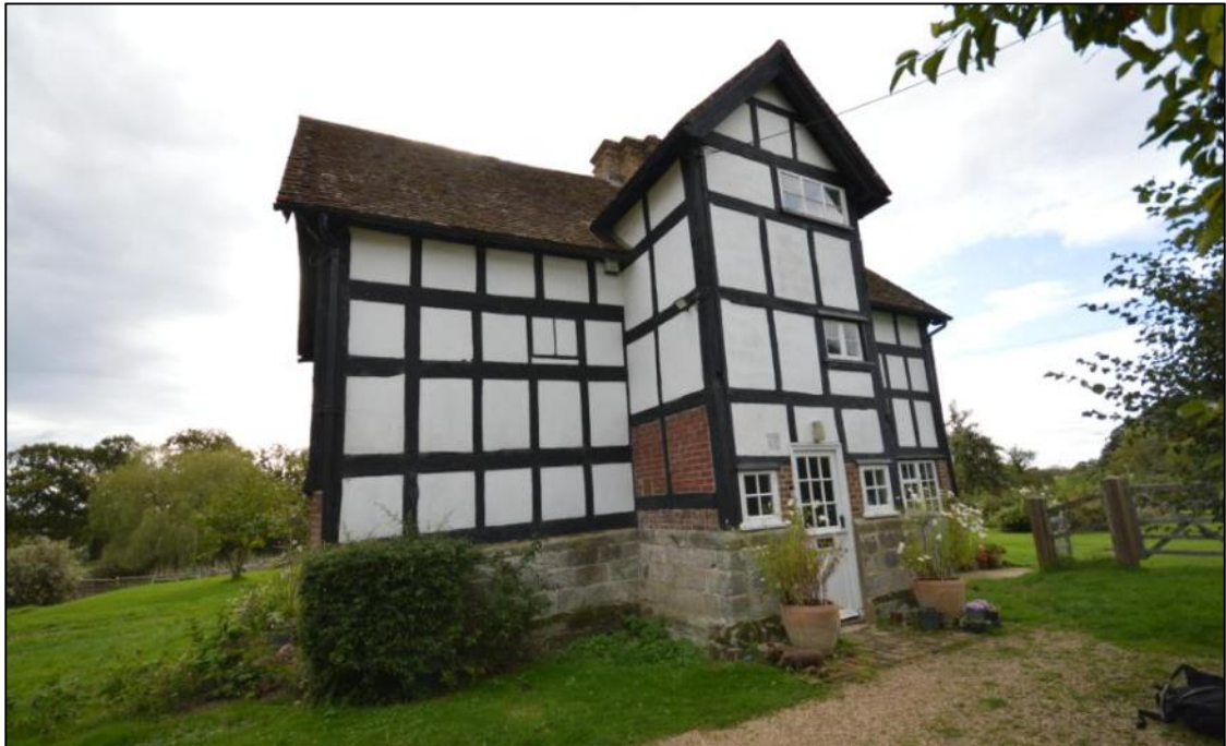
Plate 50: The north side of the cross-wing showing the masonry and brickwork
