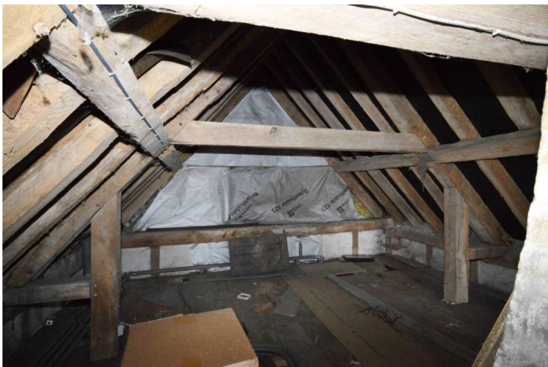
Plate 27: The roof structure with its in-line butted-side-purlins and wide-set queen studs carrying the inner ends of interrupted tie-beams
