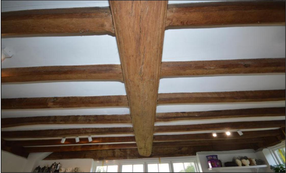
Plate 17: Chamfer and chamfer stops to the joists in bay 7
