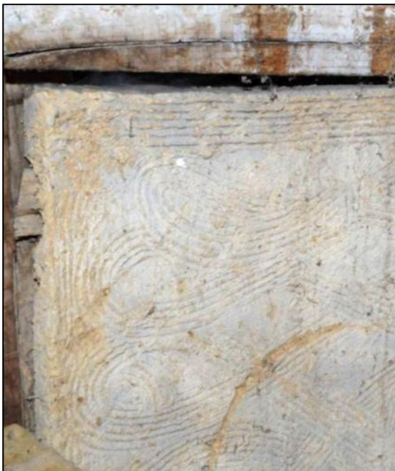
Plate 14: Comb-decorated daub (bay 5) on the south side of the cross-wing visible within the loft over the main range
