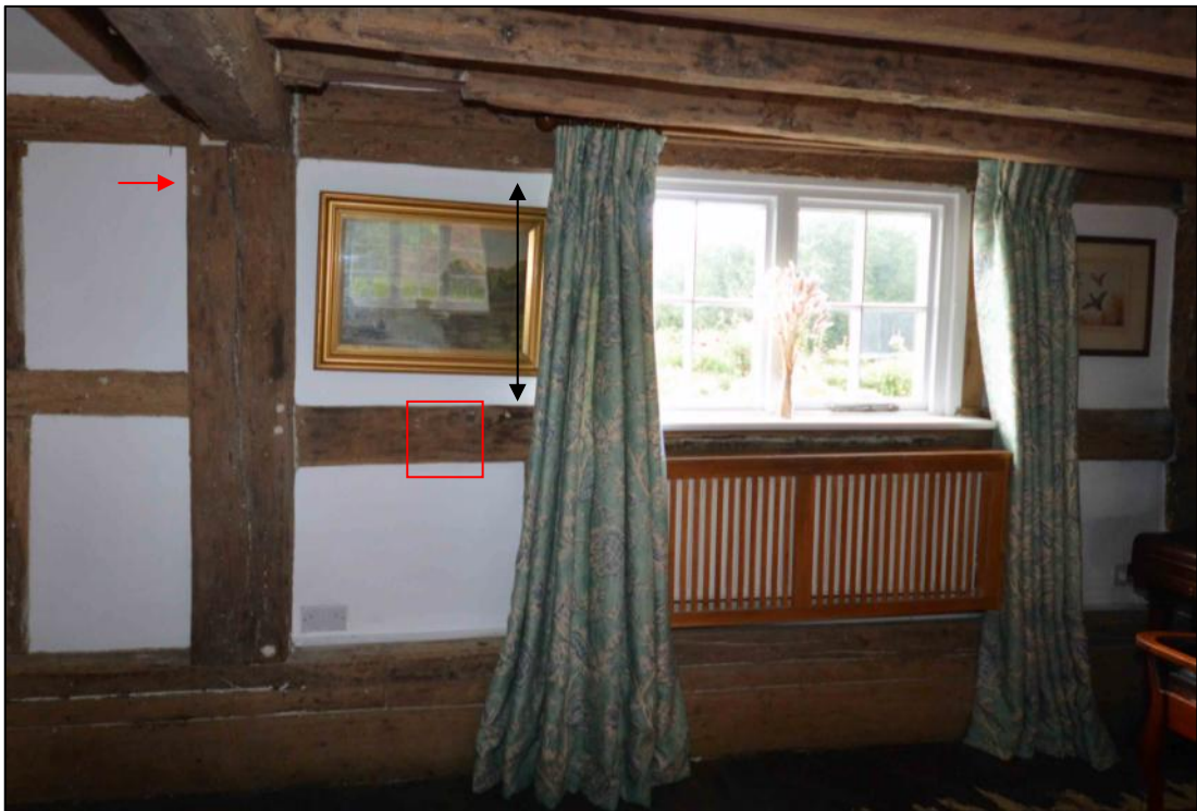
Plate 8: Peg-hole evidence (arrows) for the south jamb of the hall window; note also the double-pegs at the head of the post on its south side, indicative of a doorway head plate or lintel (black arrow). Red square marks the location of the apotropaic mark
