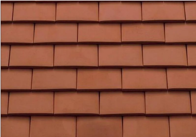
Roofing - Clay Tiles
