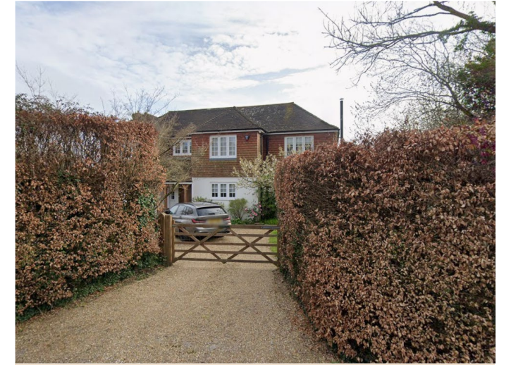
Render and UPVC Windows - 10 Top Street
