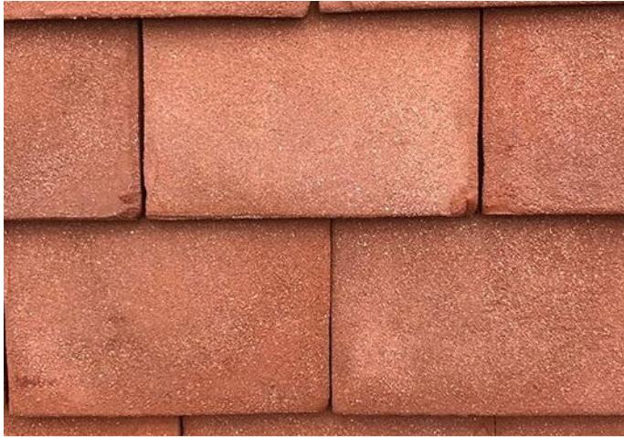
Walls - Tile Hanging (Close Up)
