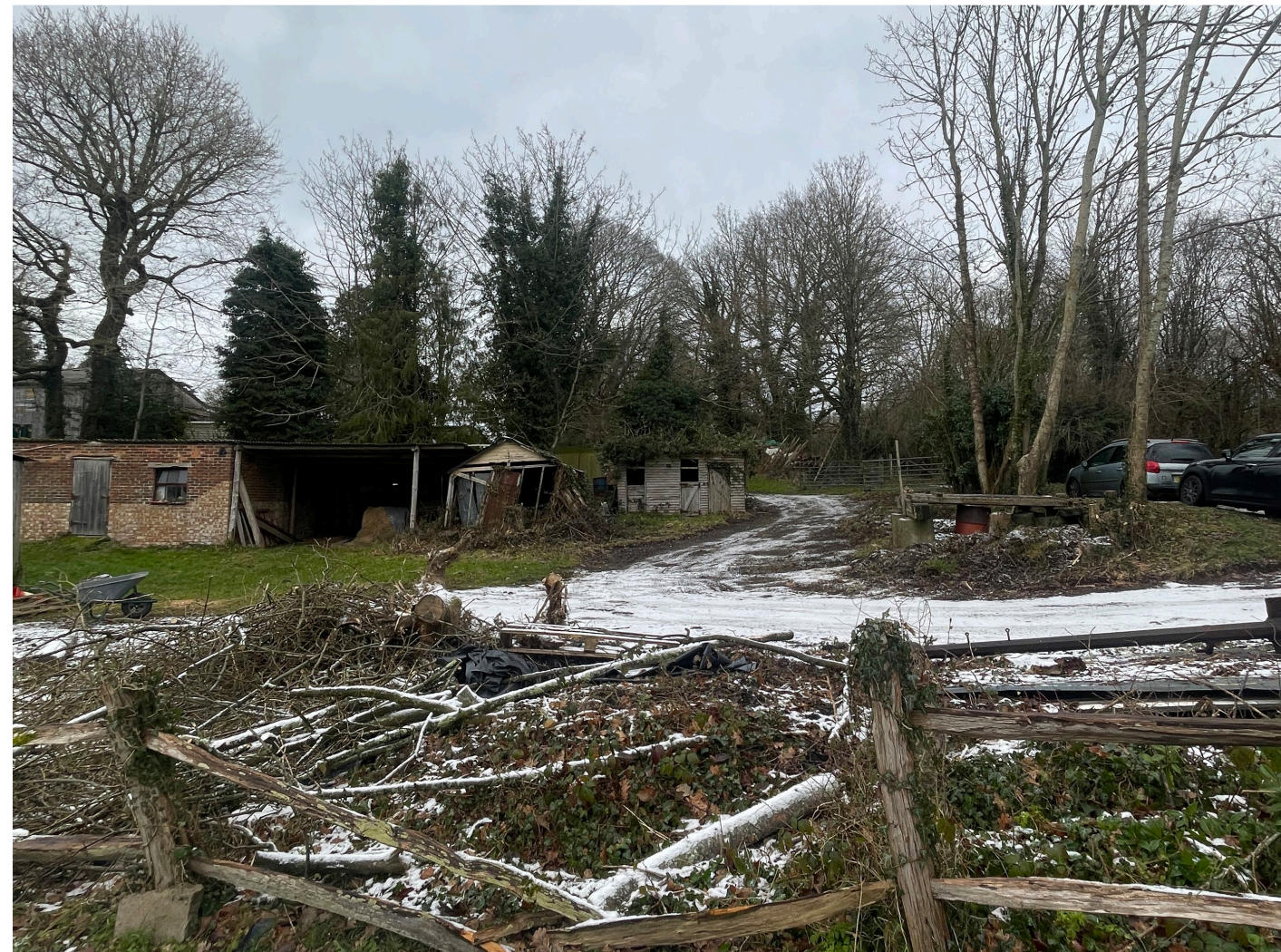
View of site from Southern Boundary
