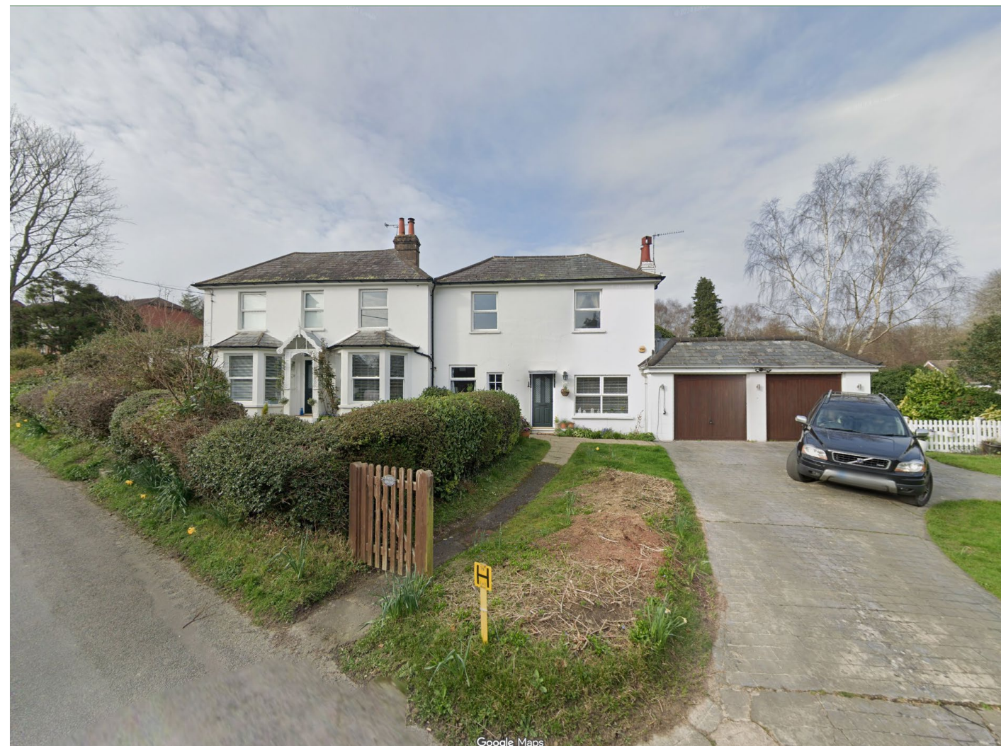
White Render and White UPVC Windows - 14 Tops Street
