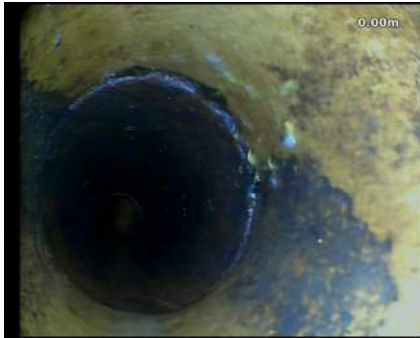
Observation [1]: Start Point: MH1
