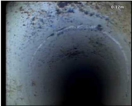
Observation [3]: CRACK
