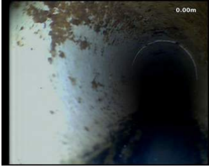
Observation [1]: Start Point: MH1
