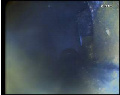
Observation [7]: End Point: INSPECTION CHAMBER -OB
