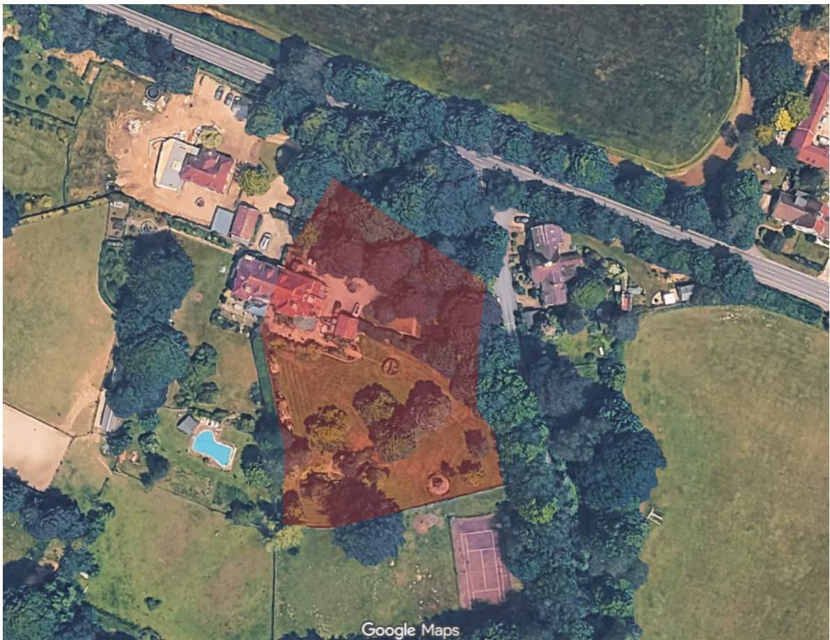
Figure 1 - Aerial photo showing site and immediate surroundings
