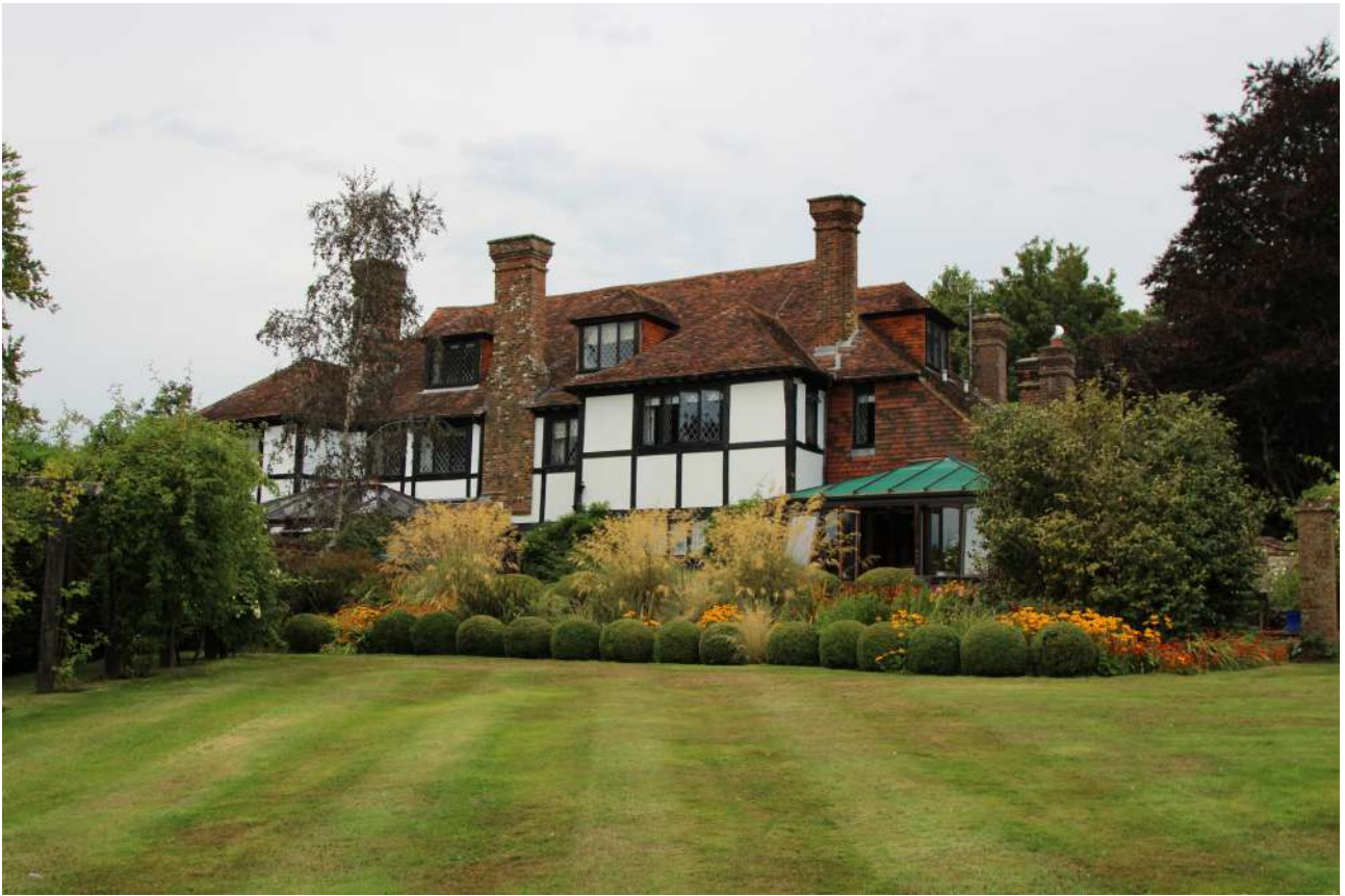
Main house standing south and looking north
