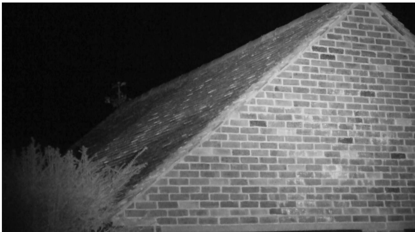
Figure 1. Darkest point from the night-vision camera focused on the northeastern elevation of the garage from the survey on 12 th August 2025.
