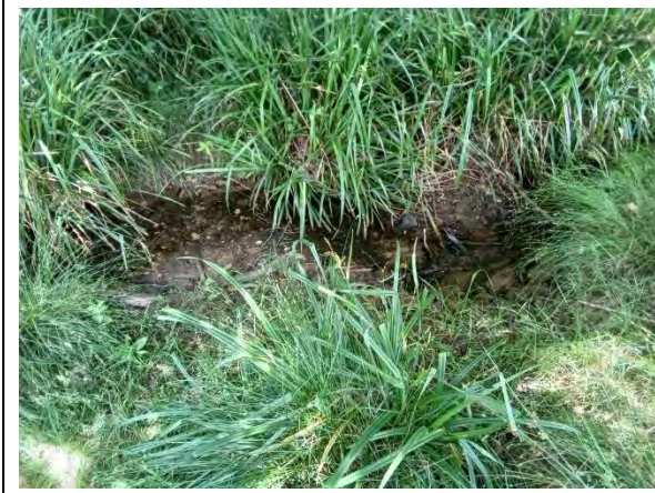
Photo 19. Ditch D2 (Running water)
