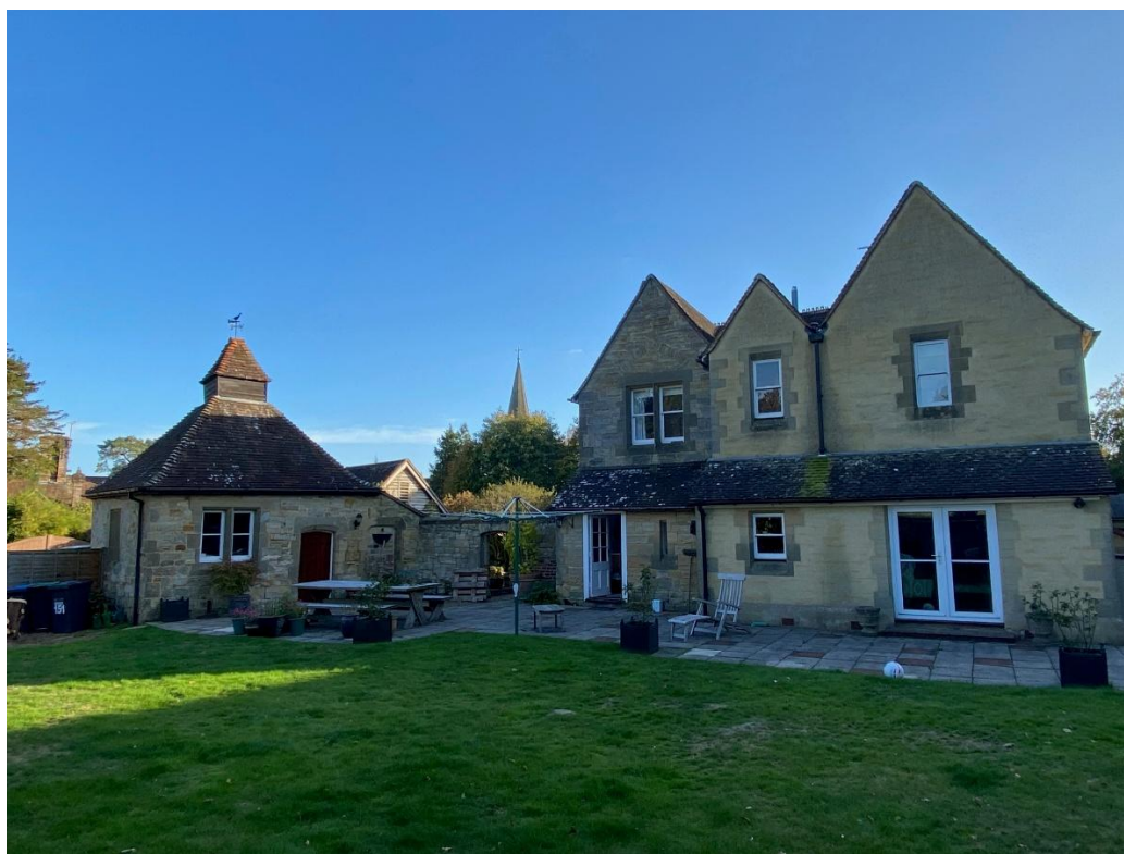
Figure 6: St John's Lodge viewed from the north. The 1984 extension is visible to the right (textured render finishes) and bothy outbuilding to left. The spire of All Saint's Parish Church is in the distance.
