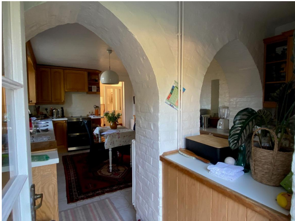
Figure 23: Arched openings into the rear lean-to which probably formed a pantry or larder abutting the kitchen.
