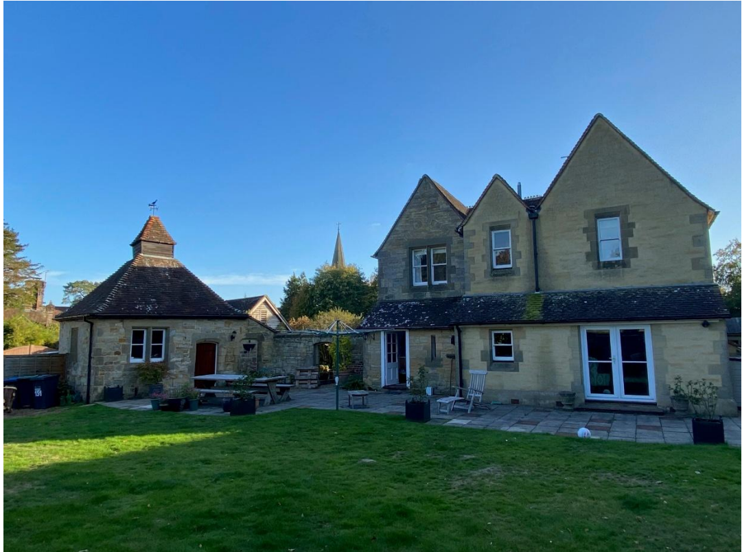
Figure 30: Looking southwest towards All Saints Church from the rear garden area.
