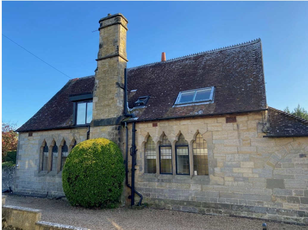
Figure 29: Former National School building to the south of St John's Lodge
