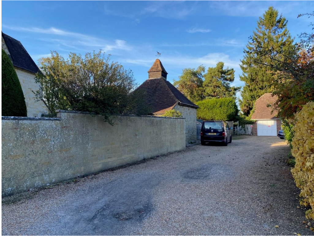
Figure 33: Cement rendered boundary wall to the east of St John's Lodge
