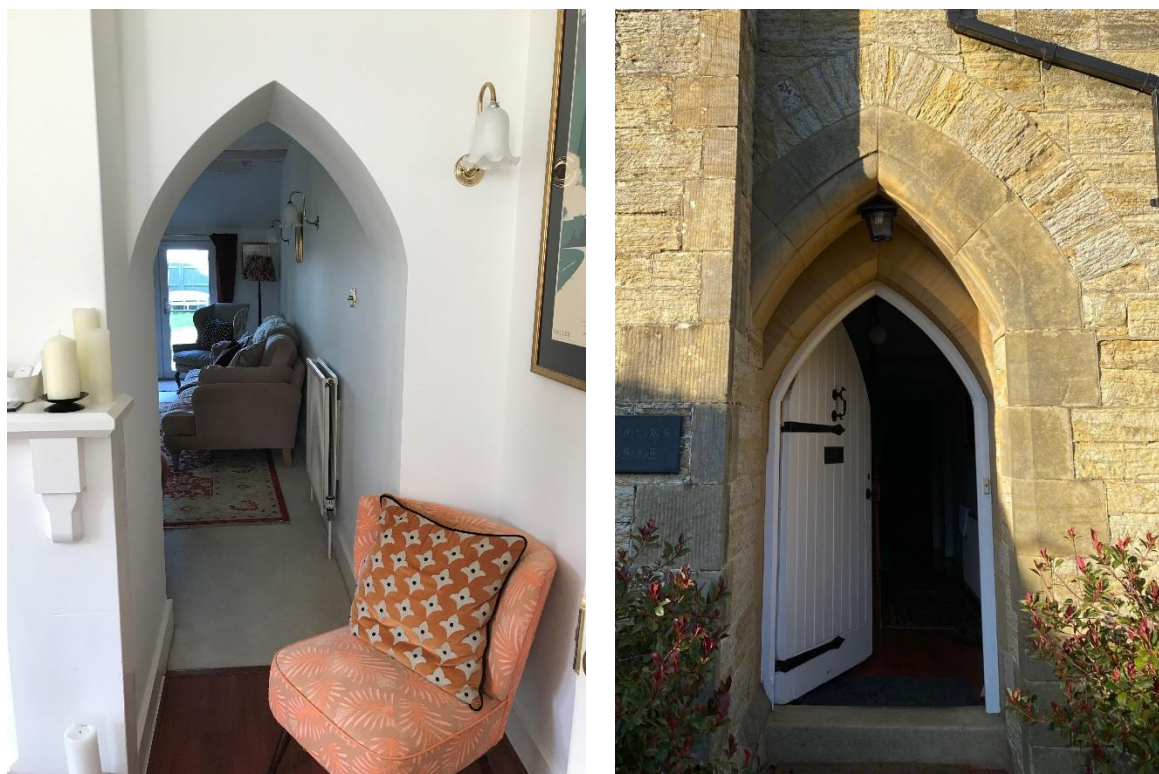
Figure 25: Two centred arch opening between the Snug and 1980s extension (left) and main entrance door (right).
