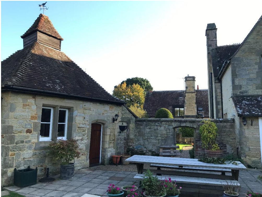
Figure 9: View of the bothy and wall linking to the former schoolmaster's house. The evidence of an additional structure to the north side of the wall in the location of the exposed brickwork corresponds to that shown on the 1875 OS Map (Figure 9). This is likely to have been a coal store or coal bunker with a sloping lid or roof.
