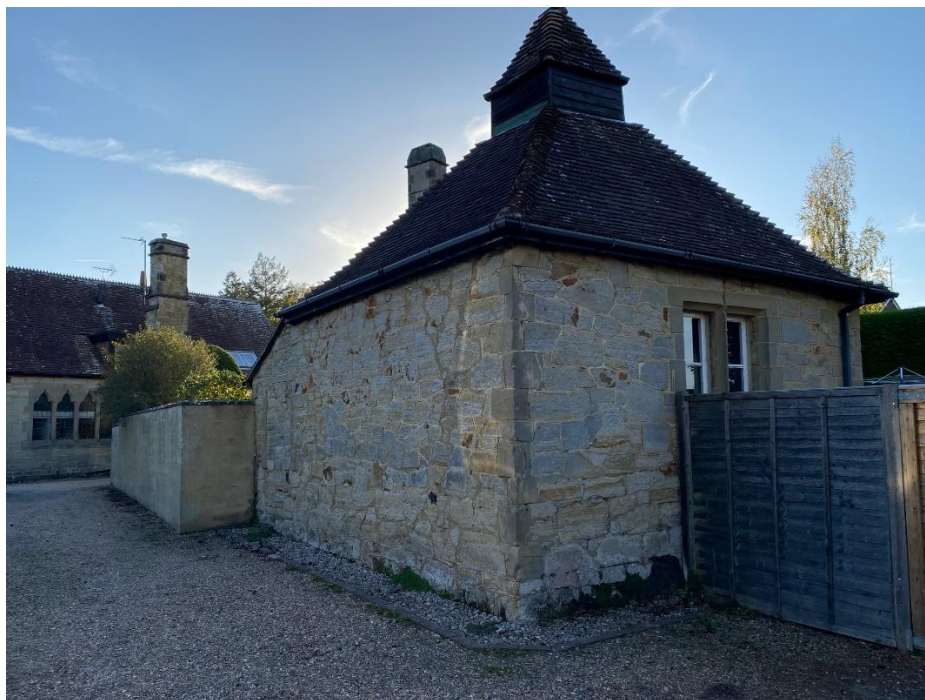
Figure 27: Bothy viewed from the northeast with blocked entrance just visible to left and former School beyond to left.
