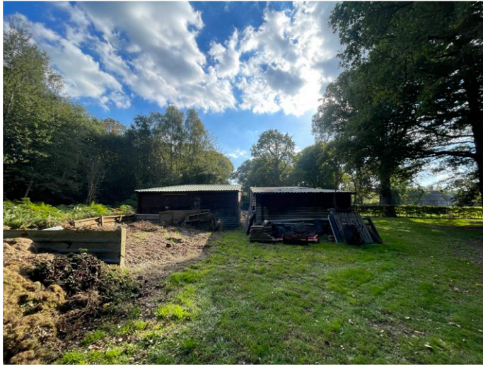
4. View of site from north.
