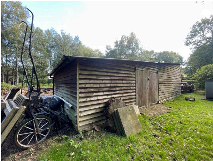
3. View of the existing barn from the north-west corner.
