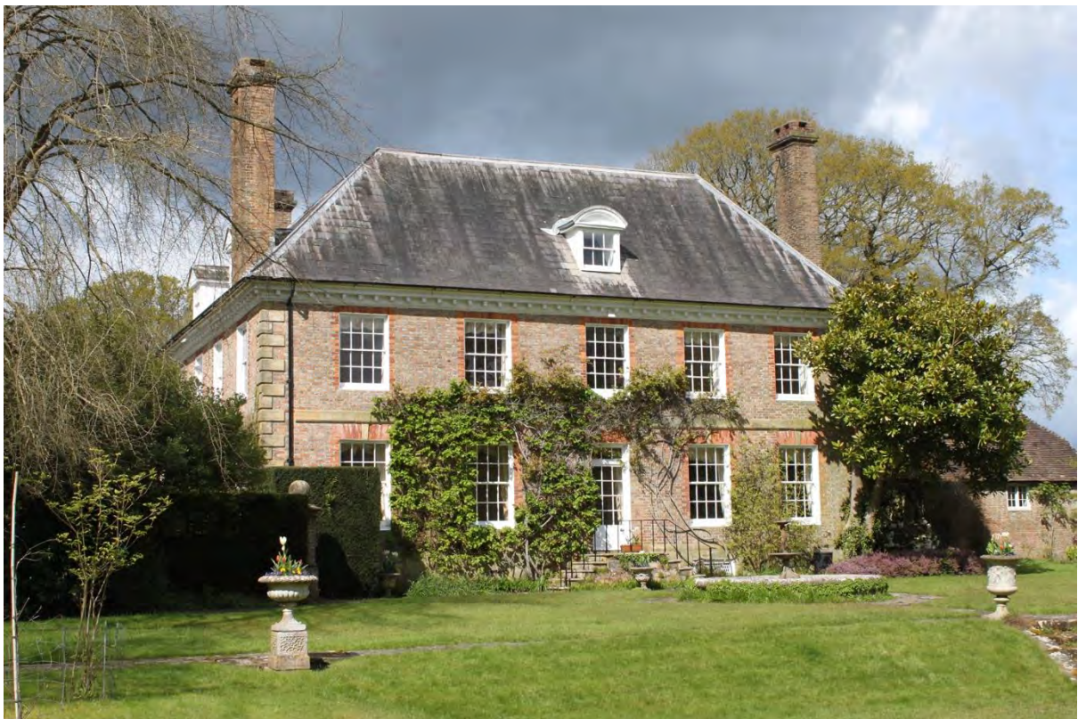
Figure 45: Plate 10 - View of the east elevation looking northwest from the south
