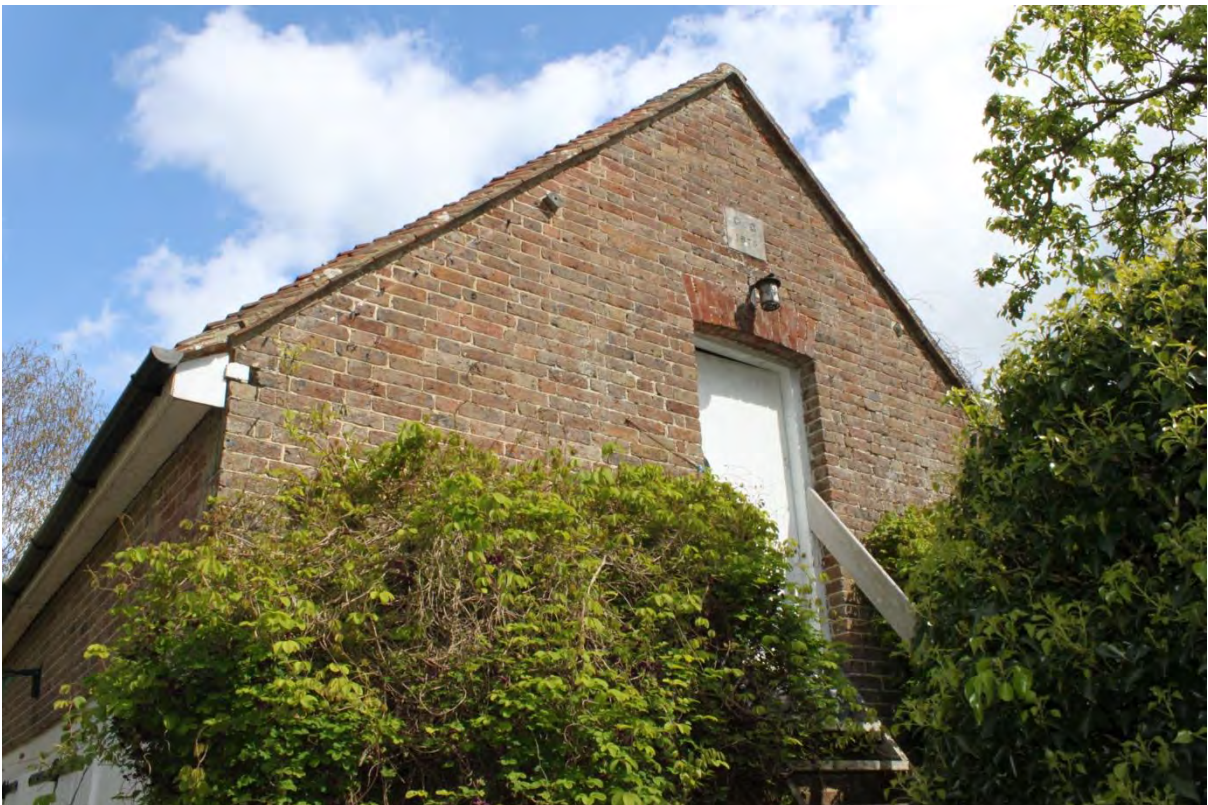
Figure 75: Plate 40 - South elevation of the garage looking northeast
