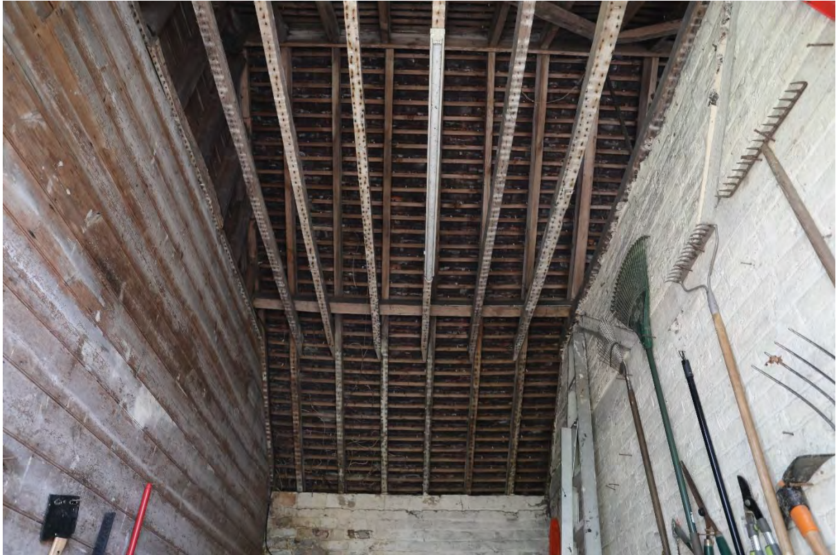
Figure 122: Plate 87 – Toolshed, view to the timber roof structure (19.03.25)
