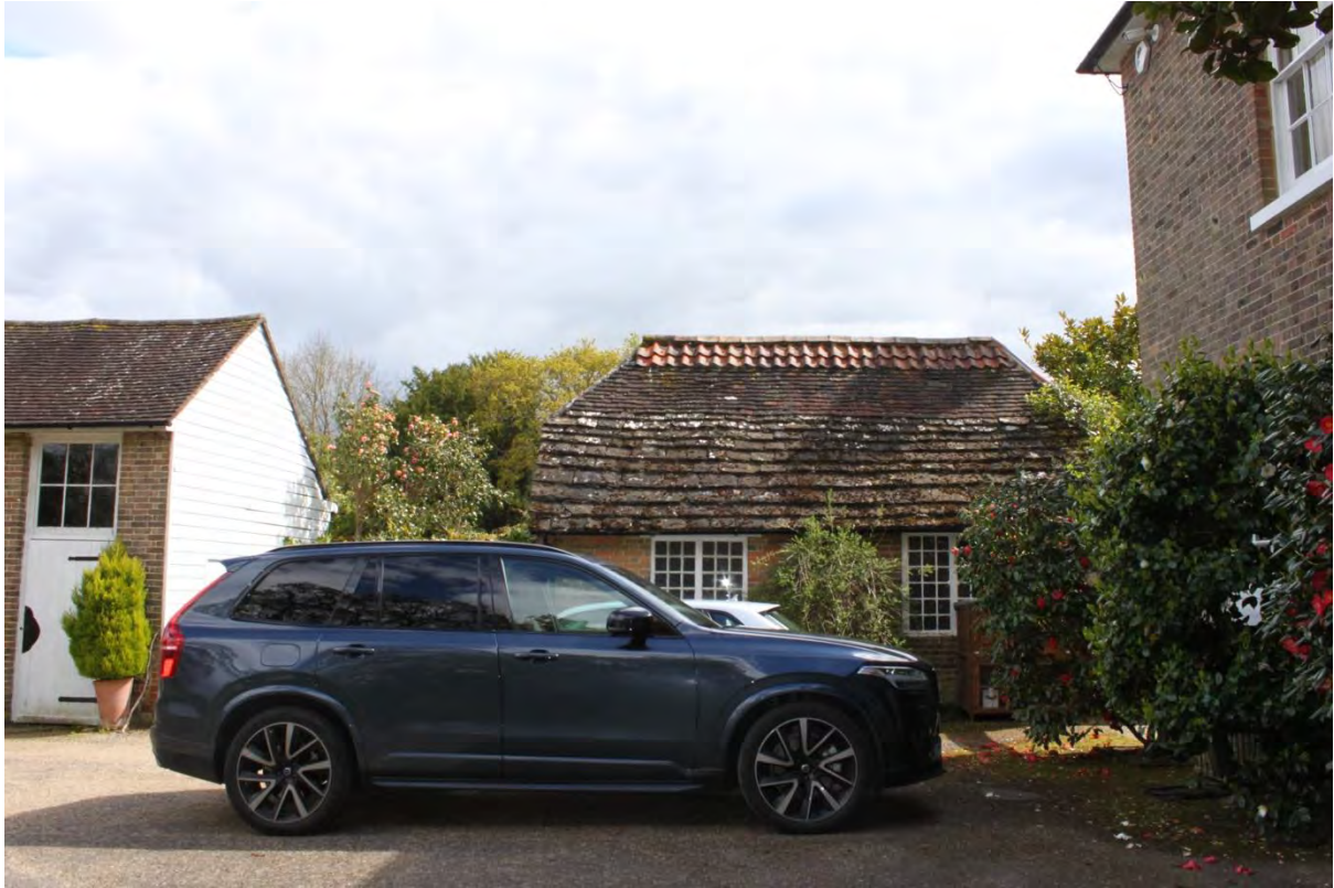
Figure 78: Plate 43 - View of the west elevation of the dairy from the west looking east
