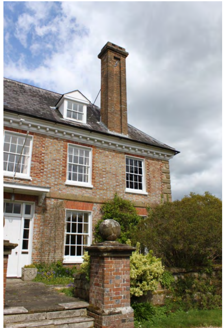
Figure 43: Plate 8 - View of the east section of the south elevation looking northeast
