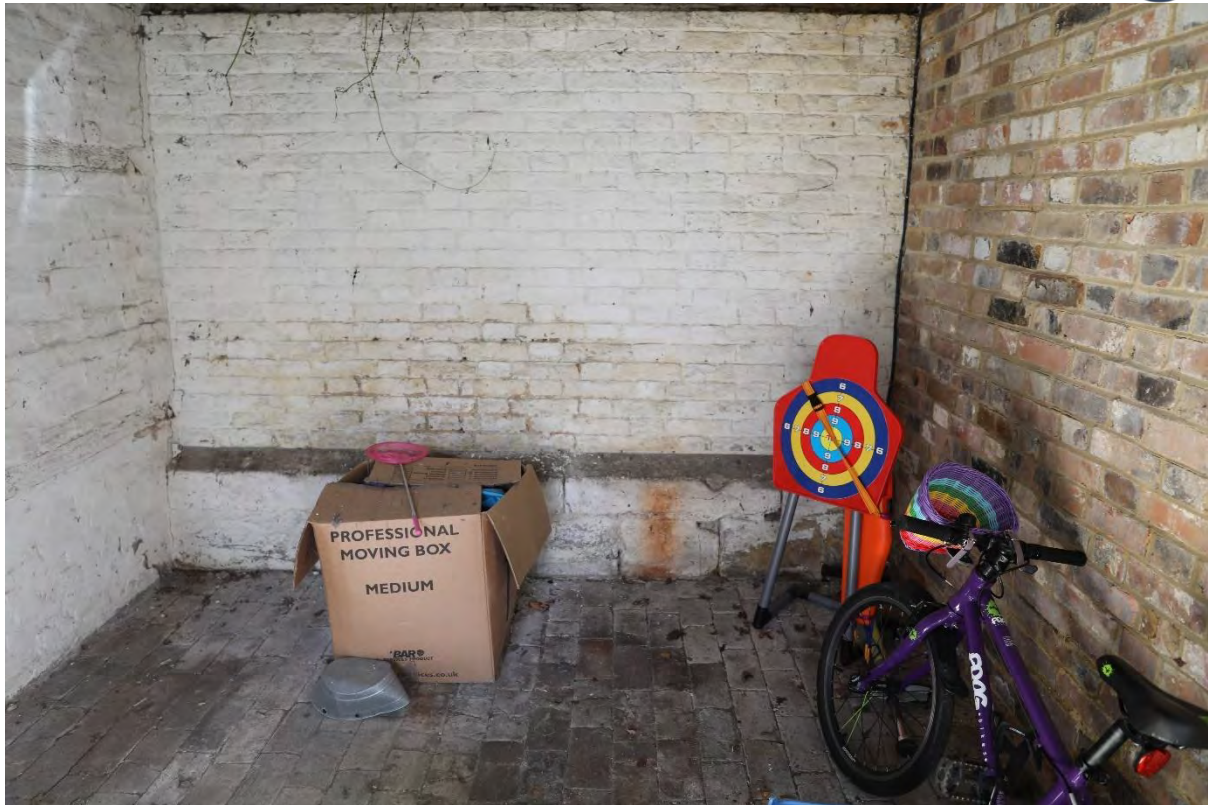
Figure 118: Plate 83 – Former Dairy, south section, view to the east wall (19.03.25)
