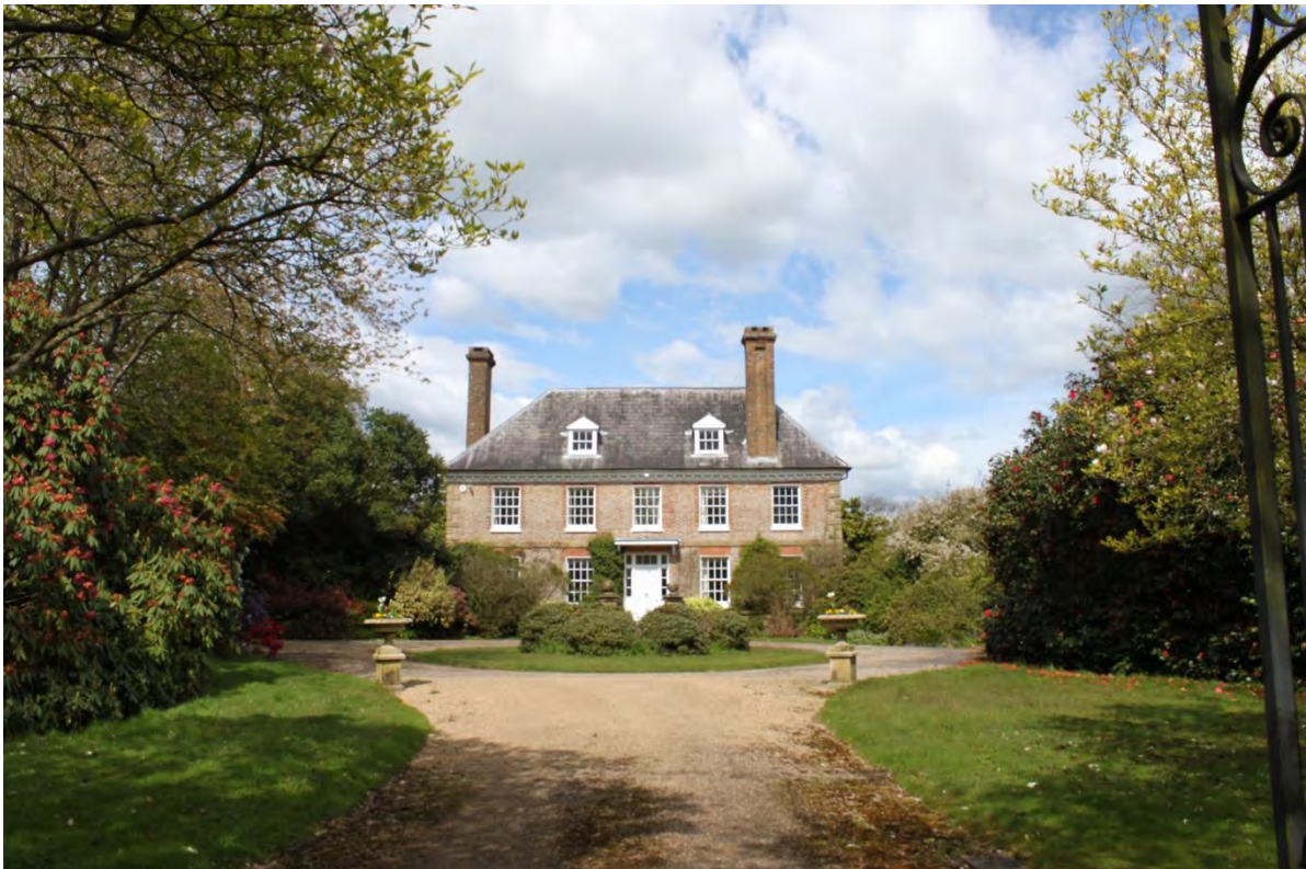
Figure 41: Plate 6 - View of the south elevation, circular drive and paths from the south looking north
