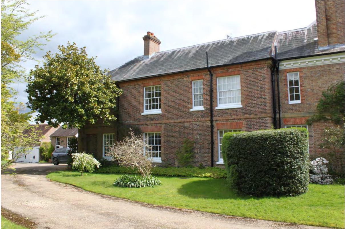
Figure 86: Plate 51 - West elevation from the south looking northeast
