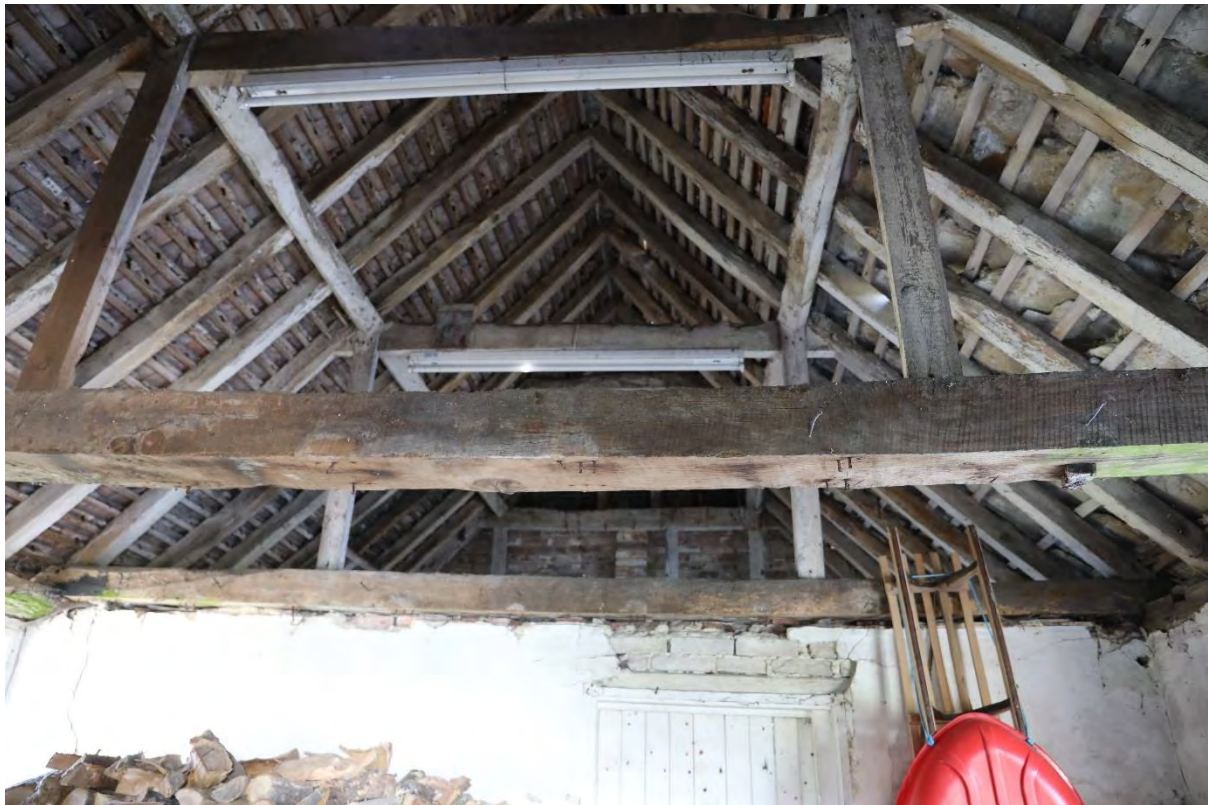
Figure 119: Plate 84 – Former Dairy, view to the timber roof structure (19.03.25)
