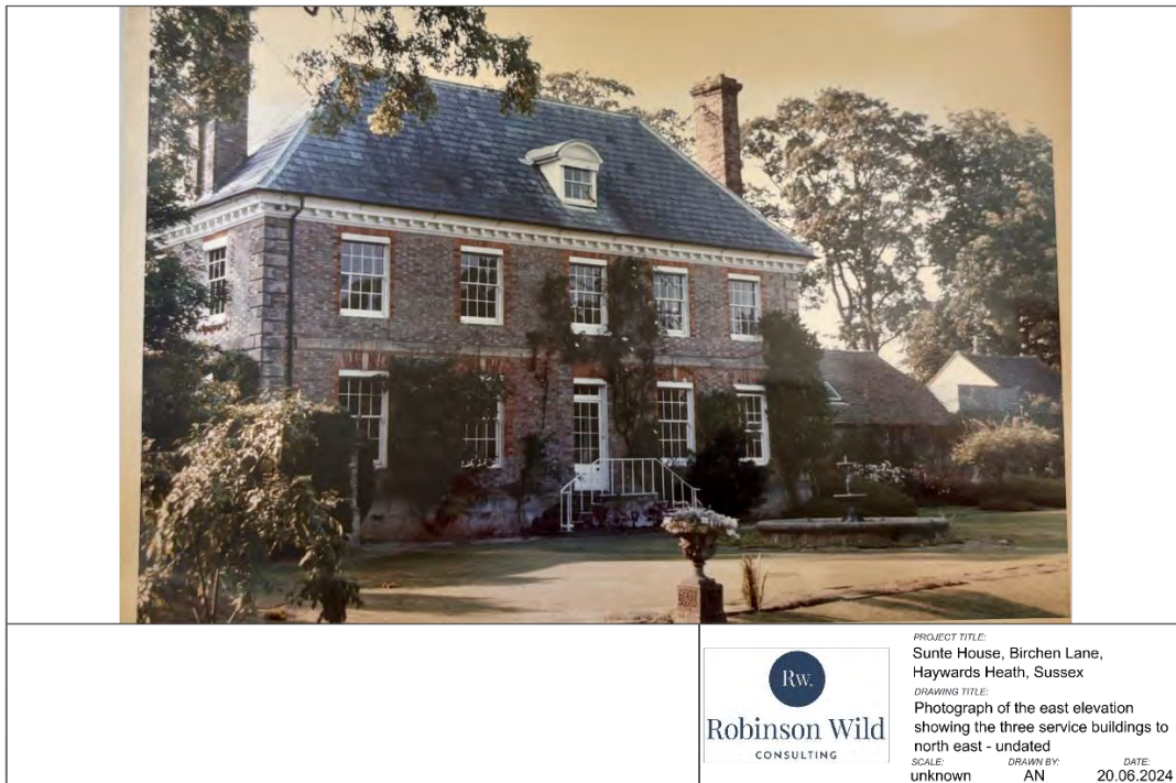
Figure 18: Undated Photograph of the east elevation showing the three service buildings to the north (source: Geoffrey Gorer Archive, ref: SxMs52/9/1/1/5)
