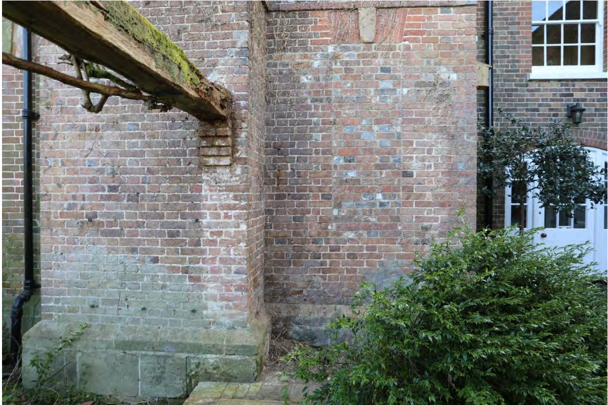
Figure 116: Plate 81 – North elevation, view to the scarring evidencing the historic abutment of the former dairy building, looking south (19.03.25)
