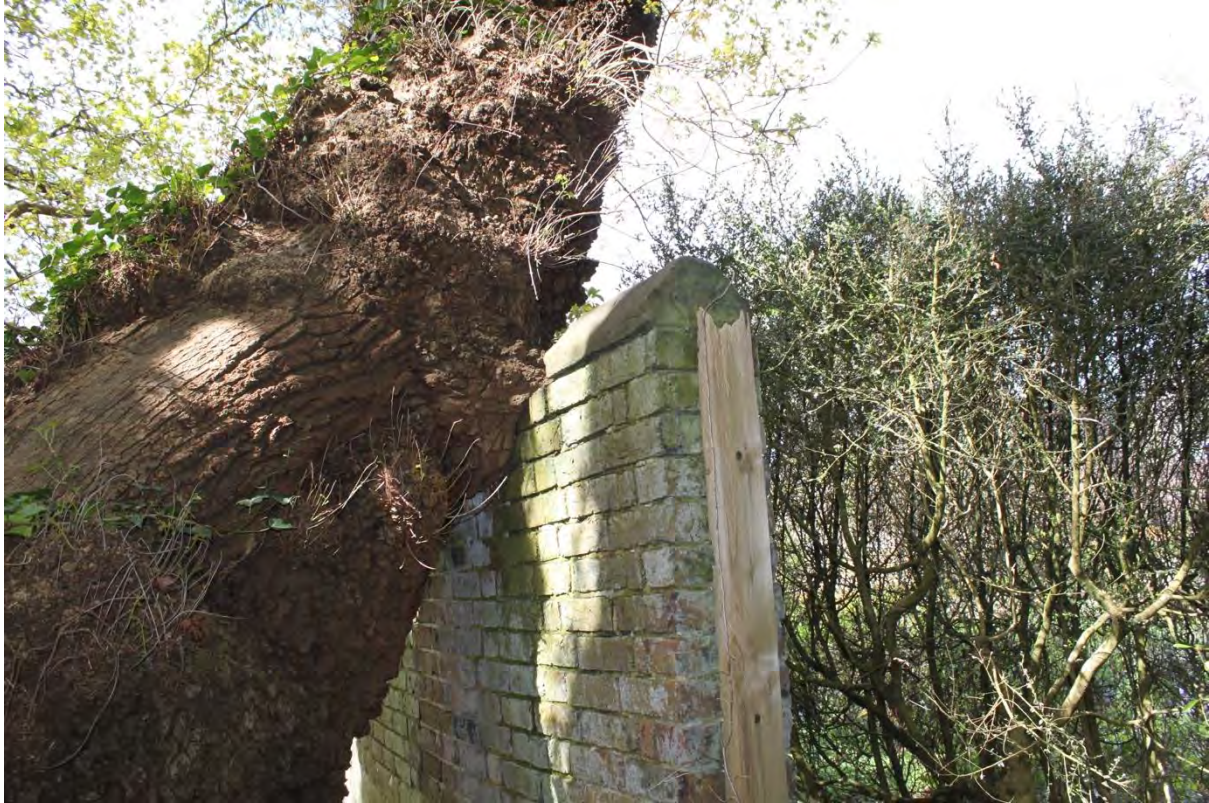
Figure 58: Plate 23 - View of the end of the listed garden wall looking northwest
