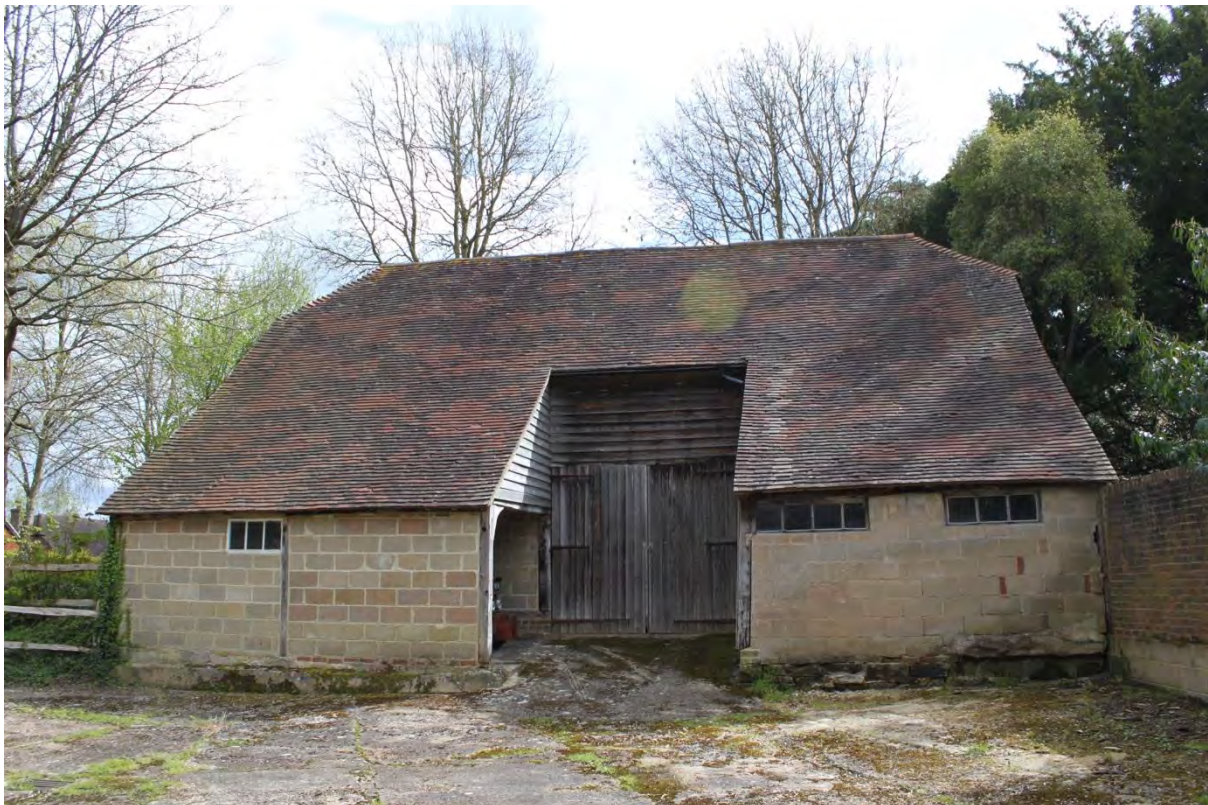
Figure 65: Plate 30 - View of the barn from the west looking east
