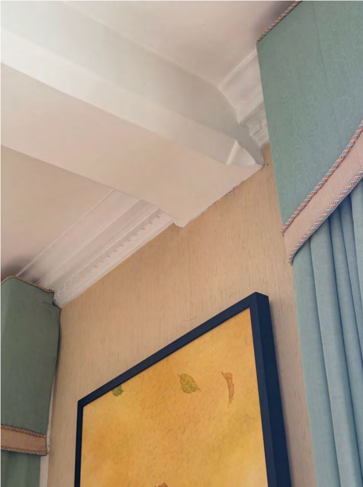
Figure 92: Plate 57 - Chamfered beam and cornice detail in the dining room
