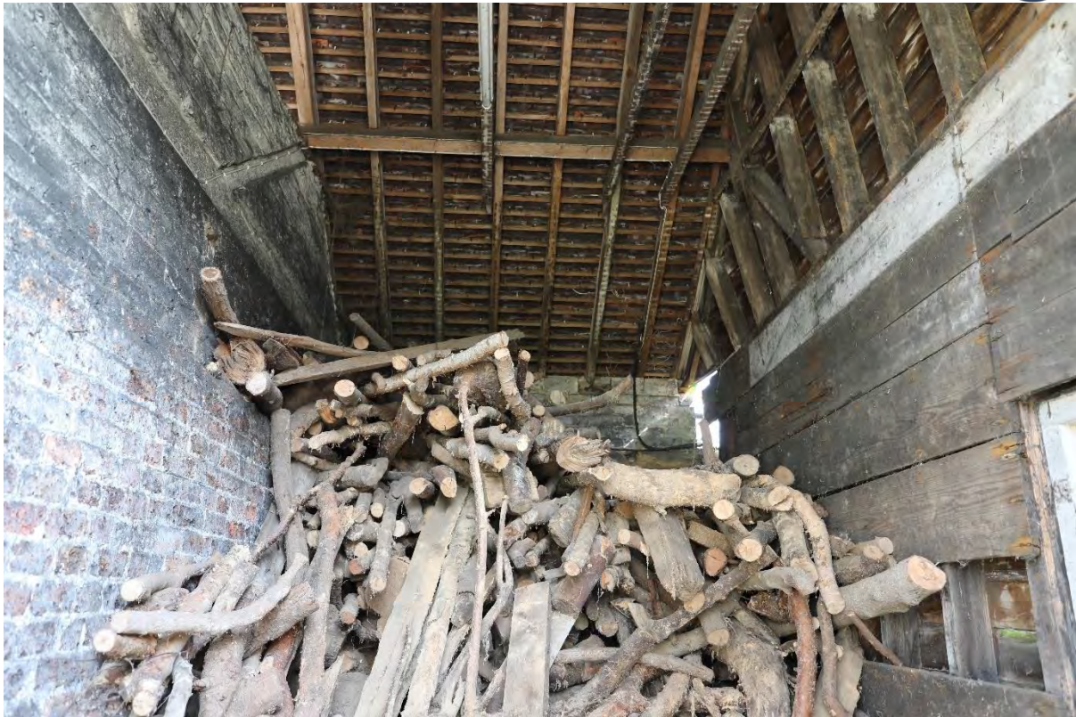
Figure 120: Plate 85 – Toolshed, view to the interior (19.03.25)
