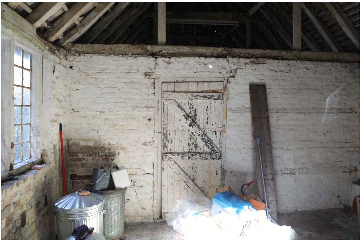
Figure 117: Plate 82 – Former Dairy, view to the brick partition wall, looking north (19.03.25)
