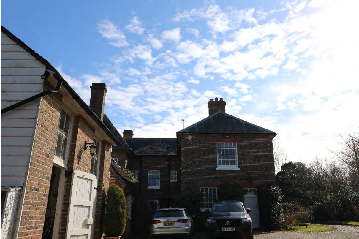
Figure 130: Plate 95 – View to the north elevation from the parking area to the north of the house, looking south (19.03.25)
