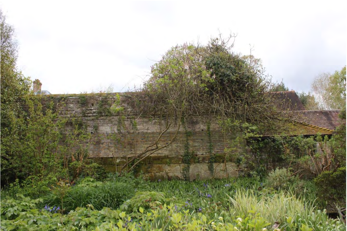
Figure 63: Plate 28 - View of the west wall from the east looking west
