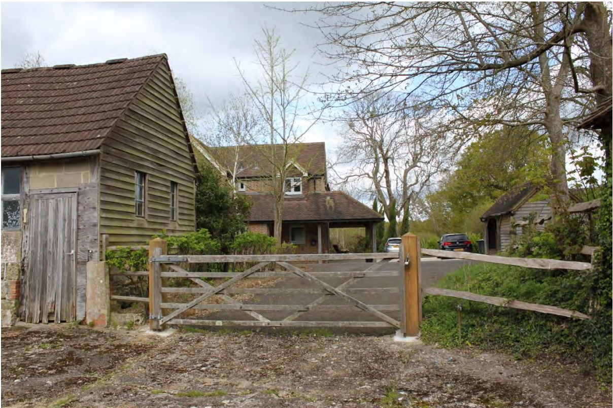
Figure 69: Plate 34 - View of development to the north of the farmyard looking north
