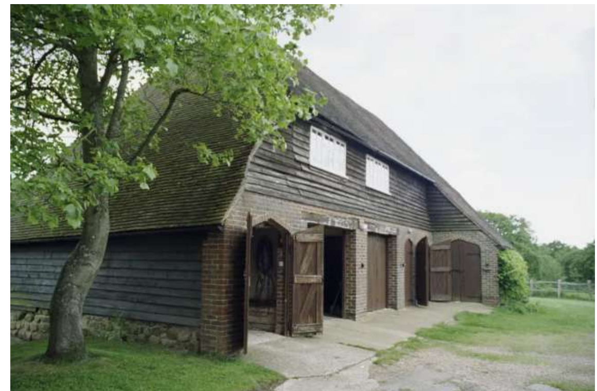
Barn to the South West of Old Beech Farm House - Historic England Archive, Mr John Francis, 2005
