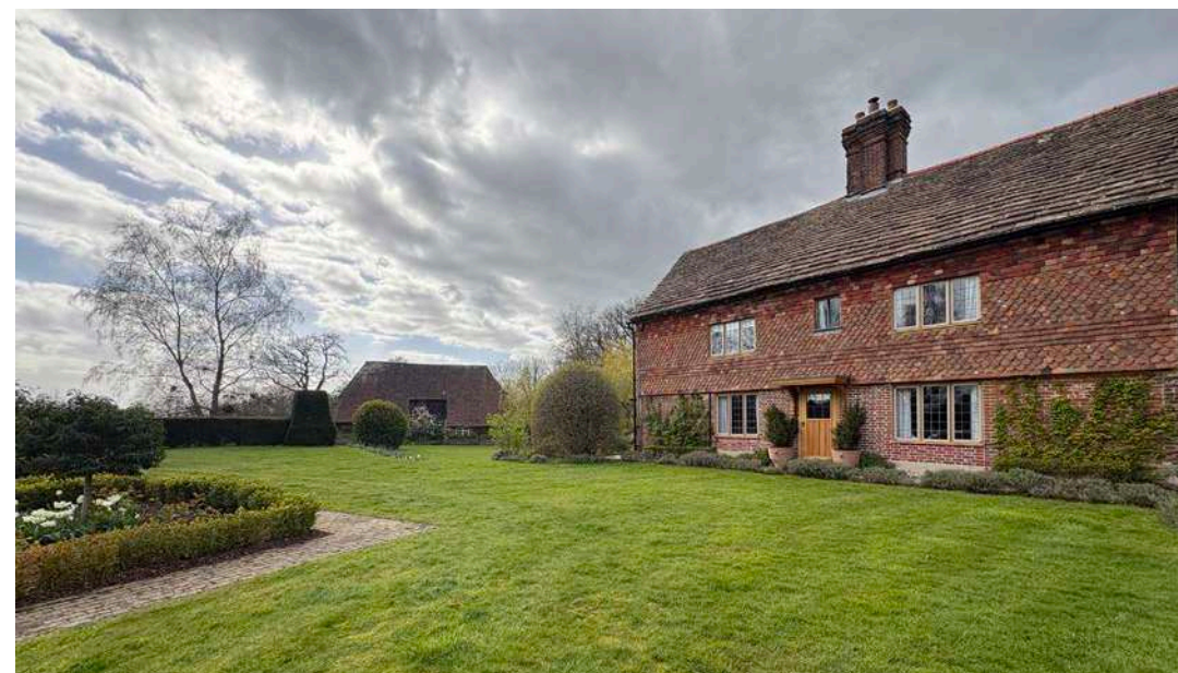
Old Beech Farmhouse, South-East Elevation
