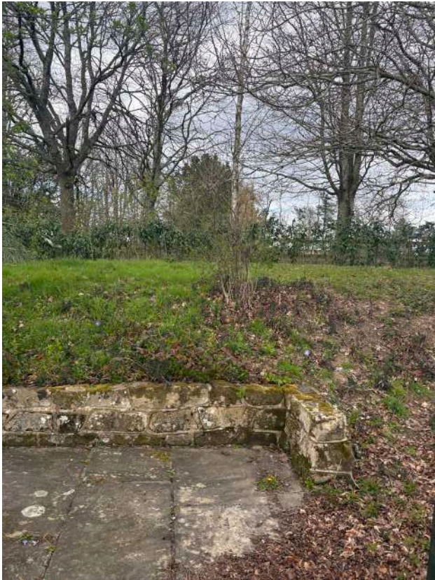
View of retaining wall to north of existing hardstanding
