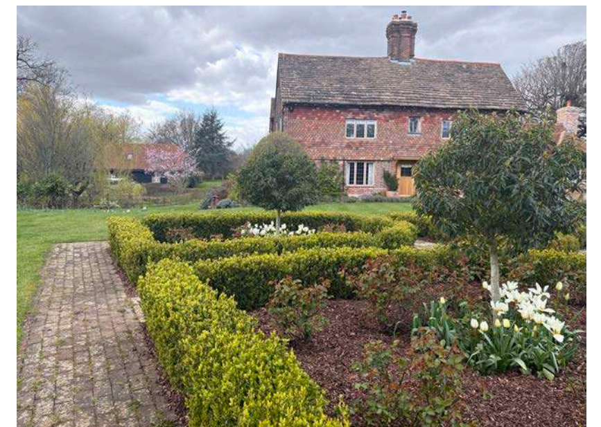
Old Beech Farmhouse, South-East Elevation, behind existing planting
