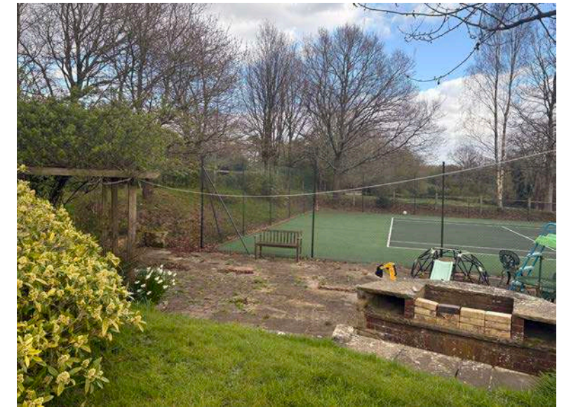
View looking east over existing hardstanding
