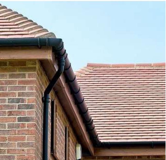
Cast iron rainwater goods To match farmhouse
