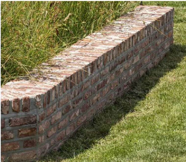
Red brickwork retaining walls in Flemish bond To match existing farmhouse and pool house
