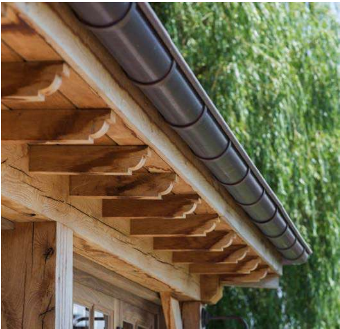
Oak eaves To match farmhouse extension
