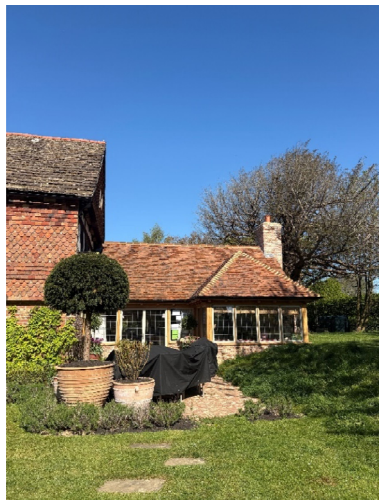
Figure 1: Existing farmhouse, kitchen extension
