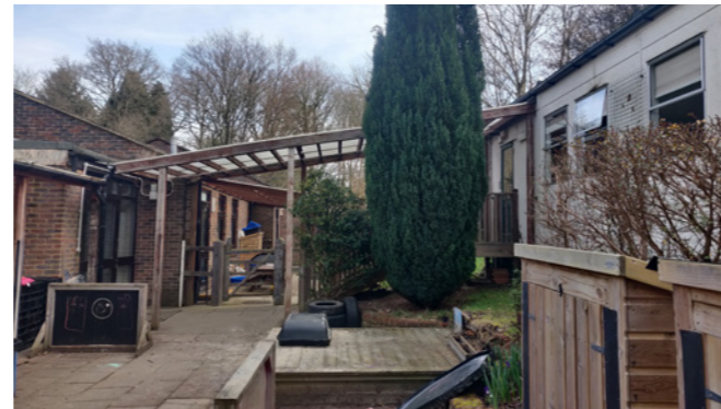
Image 11. Canopy for modular classroom
