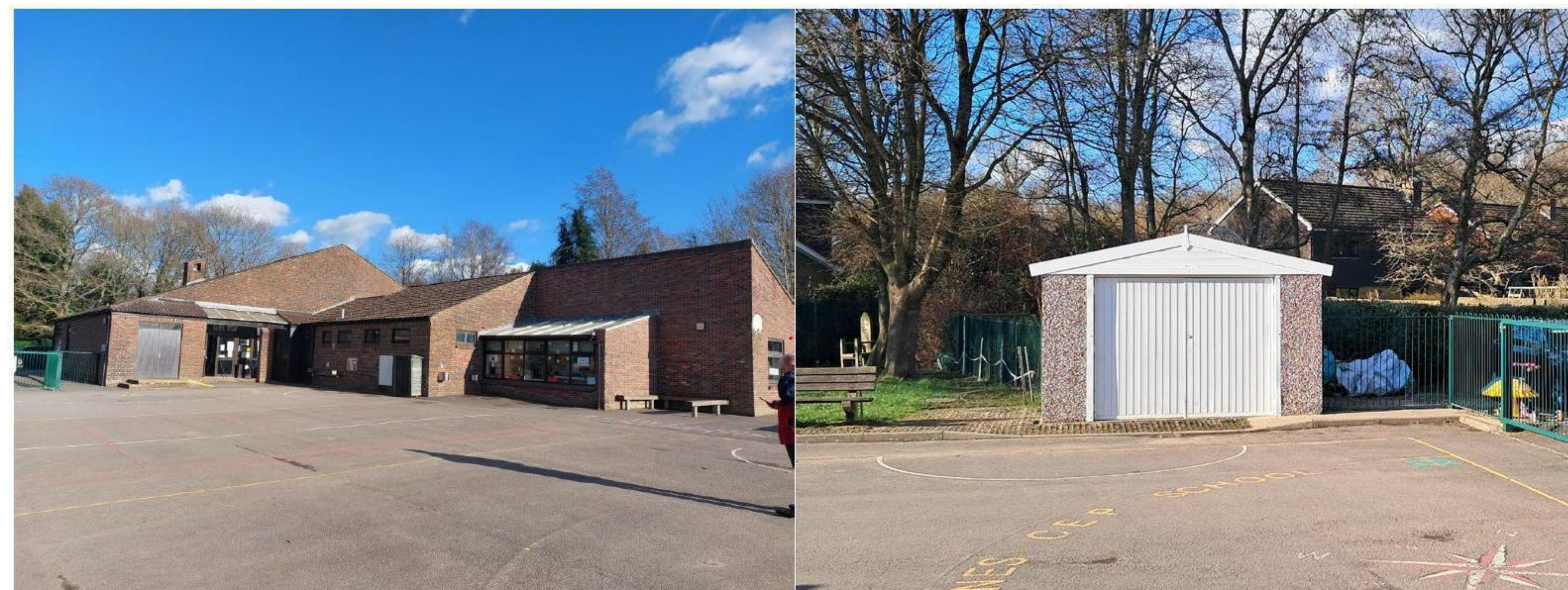
Images 02-03: North facing side of B01 (left) and south facing side of B02 (right).
