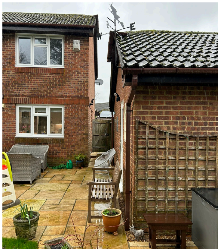
Rear view of garage & house
