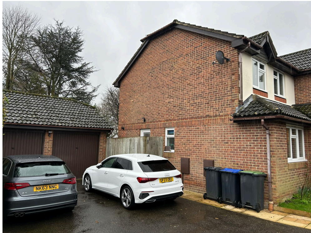
View of side of 1 Dexter Drive
