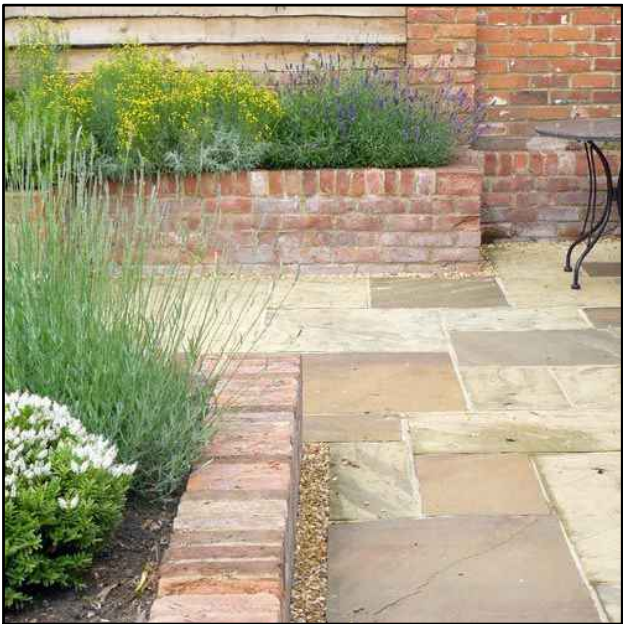
Reference Image: Brick retaining walls to patio perimeter
