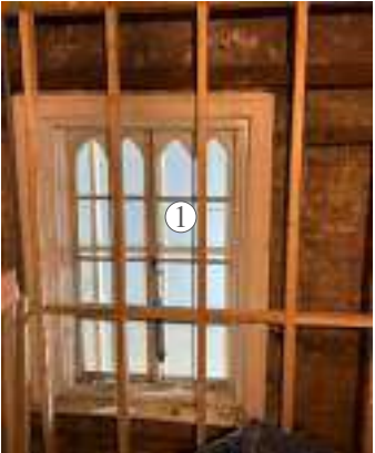
Photograph of the gothic window retained but hidden behind internal wall (wall
