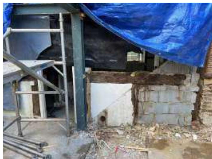
Breeze block within external and internal walls
