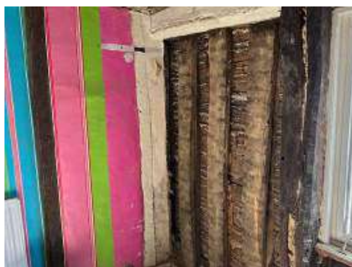
Gypsum plaster infill panels and wallpaper to walls, plastered ceiling hiding timber frame underneath
