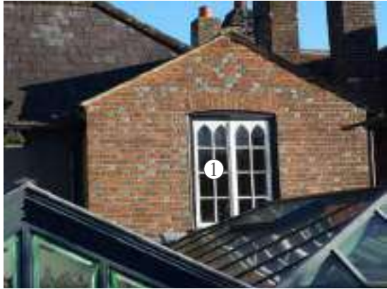
Photograph of the historic rear extension gable with gothic window
