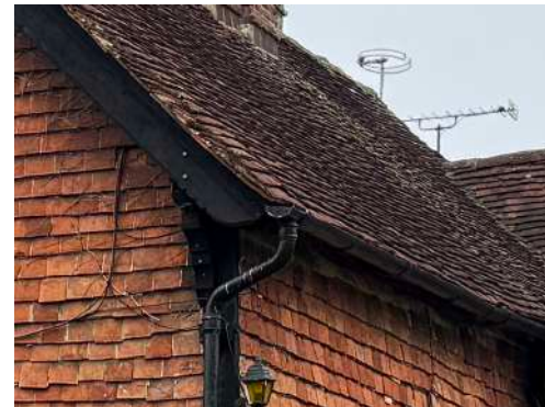
verge and eaves to west elevation of C17th range
