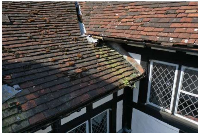
valley & abutment to north elevation of C17th range
