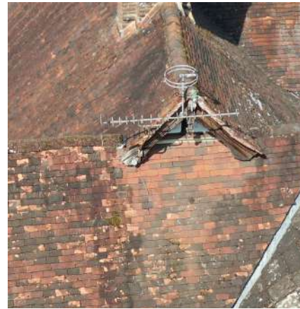
verge of gablet to east elevation of C17th range
