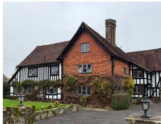
west elevation of C17th range
