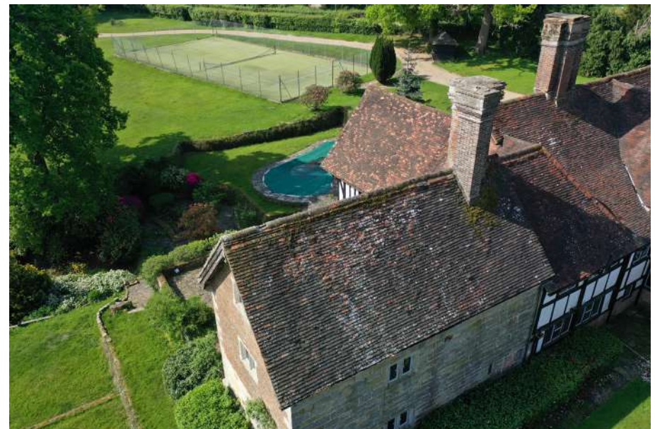
clay plain tile to north slope
