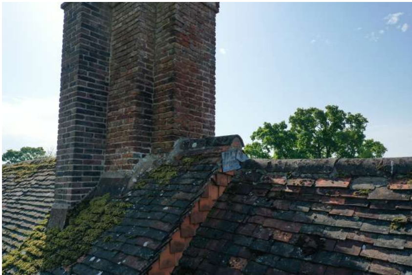
lead dressings and tiled fillets to chimney
