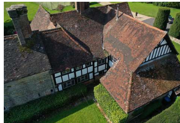
east elevation of C20th range
