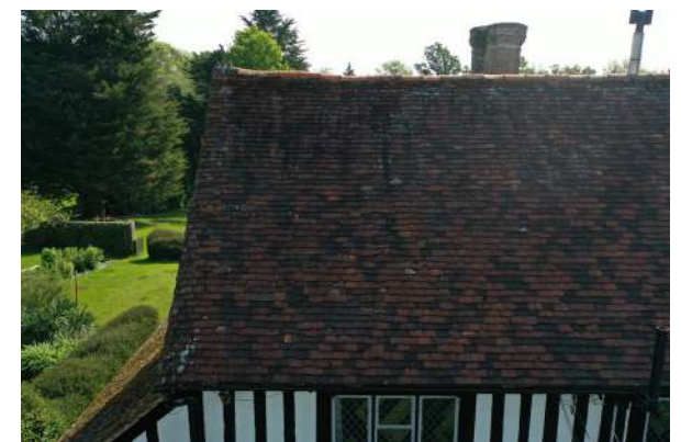
characteristic variation in pattern and gauge to west slope
