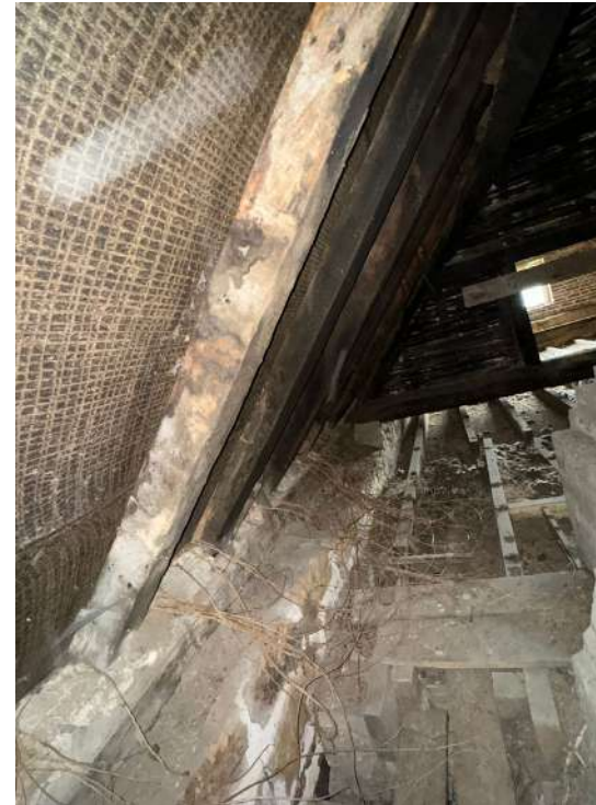
attic space showing sarking felt underlay
