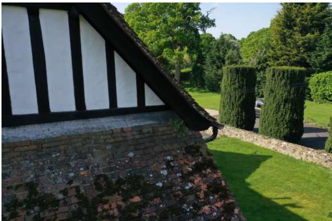
lead flashed abutment to gable
