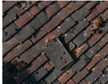
slipped peg tile to C17th range
