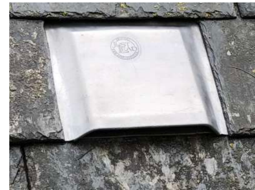
lead bat arch installed in plain clay tile and slate roof
