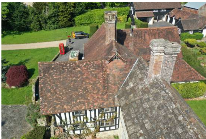
east elevation of C17th range
