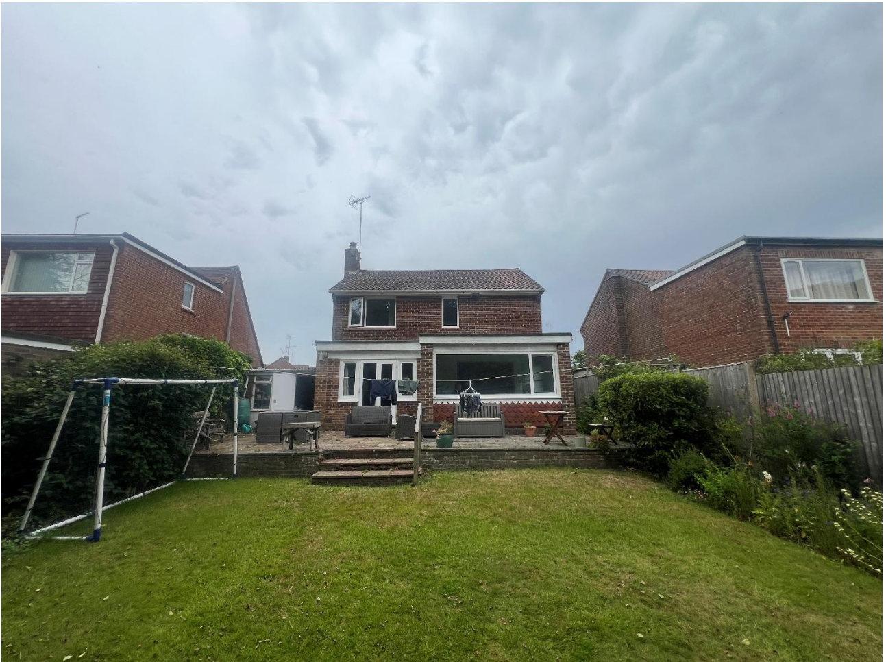
Photo of rear elevation
