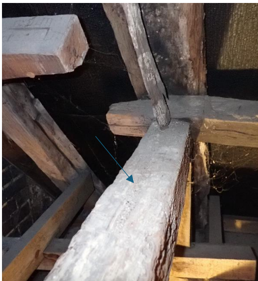
Figure 5: collar clasping the eastern side purlin is not faced with the rafter. The side purlin also truncates just to the north of this collar.
