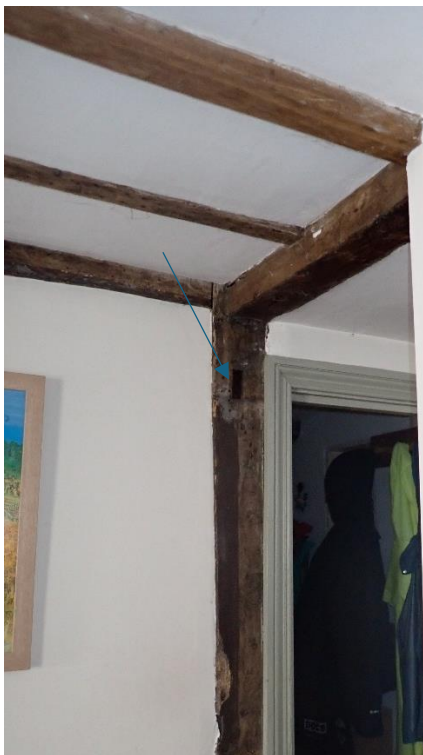
Figure 12: empty mortice for a former doorhead. Leading to the staircase.
