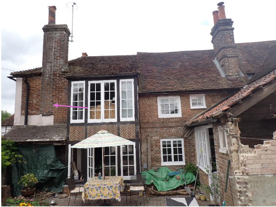
Figure 43: Additional room and a flue added to the south end of Phase A and D1 of The Friary.
