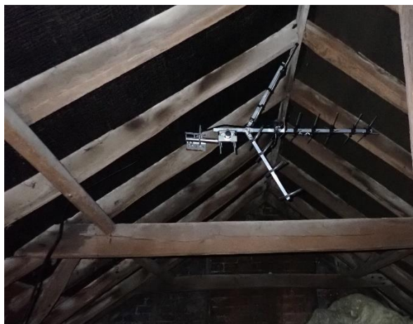
Figure 29: the softwood roof over the front range.
