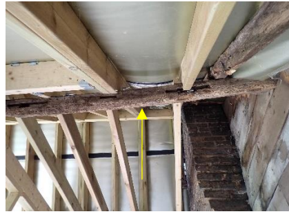
Figure 35: The purlin extending into Bay 7.
