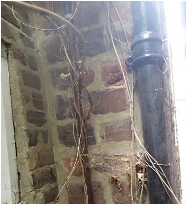
Figure 30: Brick on edge of the northern chimney.
