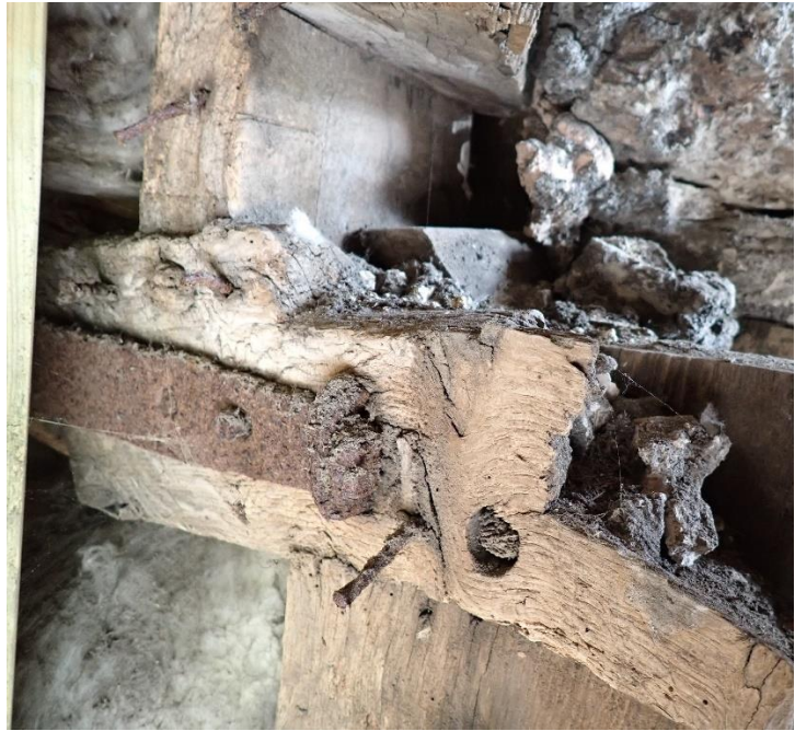
Figure 18: side view of the same bay post, showing the wall plate with a wrought iron strap.
