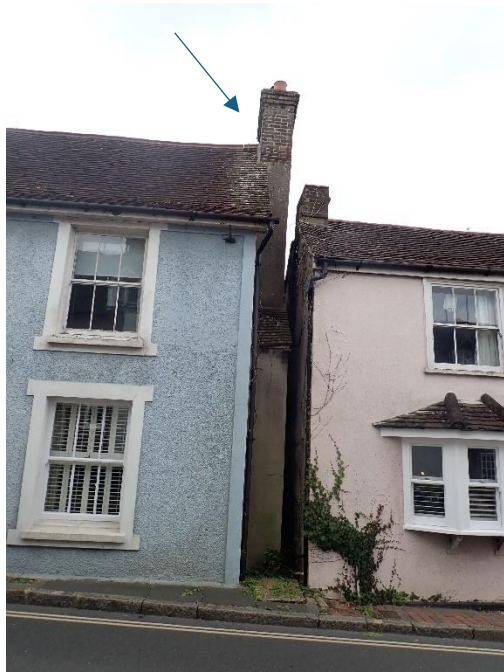
Figure 14: Chimney stack at the south end with three flues.
