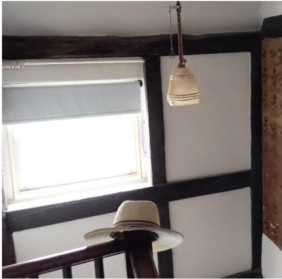
Figure 3: Small panel framing on the east wall of Bay 1.
