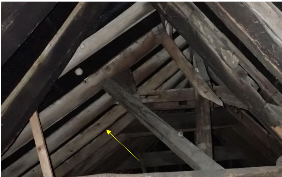
Figure 24: The new rafters over Bay 2, utilising some reused timbers, evidenced by the redundant mortices.
