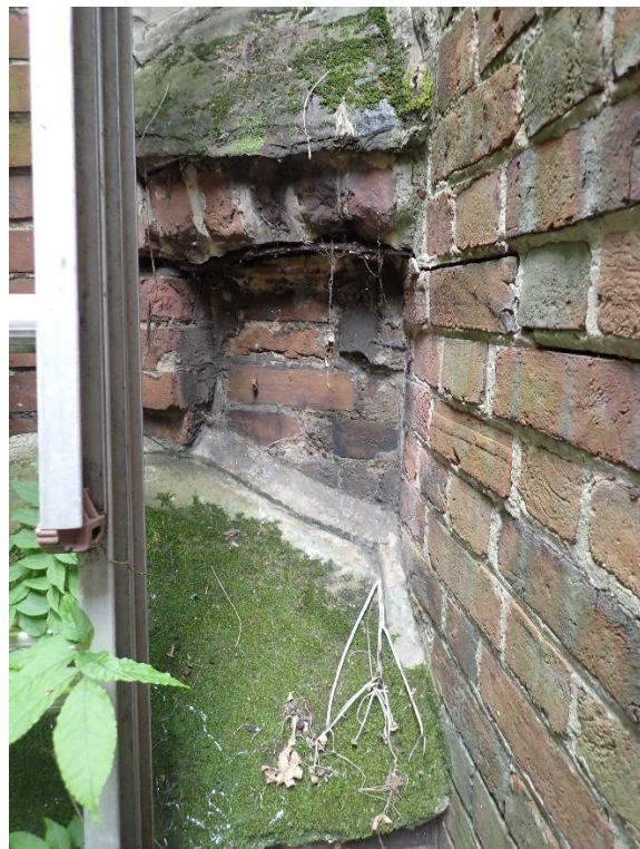
Figure 13: Blocked up opening for a former bread oven, on the southern chimney stack.
