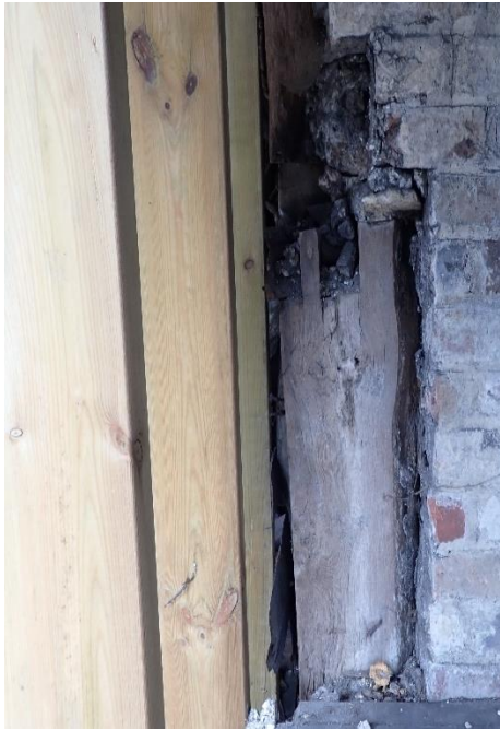
Figure 17: Top of a bay post, in the southern wall, on this Phase C1 extension. Now redundant as the wall was lifted higher in Phase E
