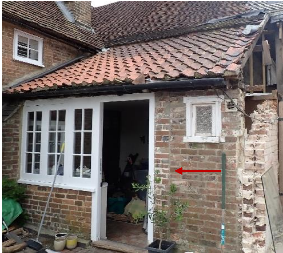
Figure 48: The only remaining part of this Phase, to the east, identified by abutment in the brickwork
