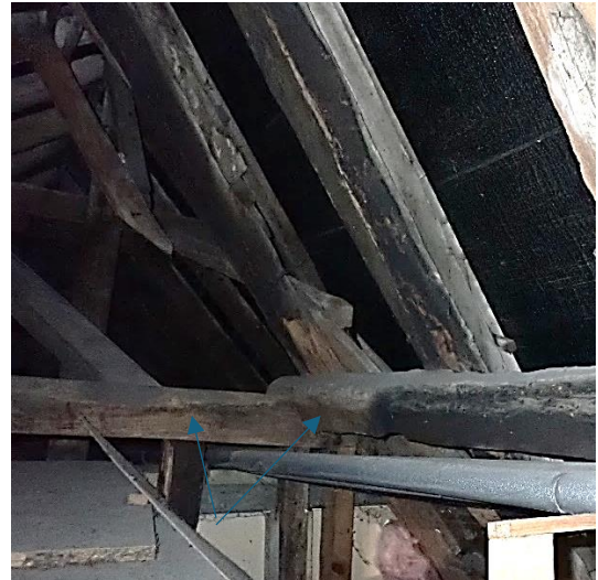
Figure 8: Mixed pattern of smoke blackened and not smoke blackened western side-purlin and collar.
