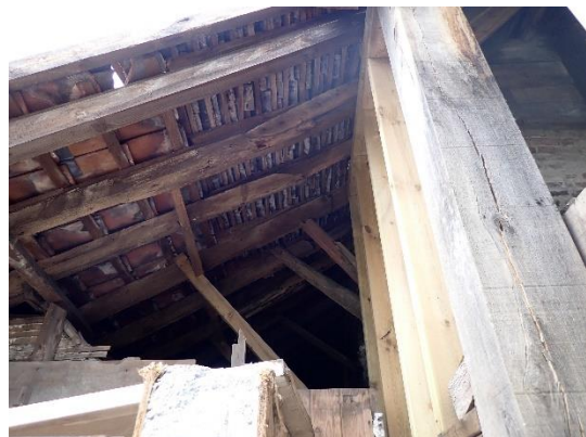
Figure 46: the lean-to roof abutting the framing of Somners , on the right hand side.
