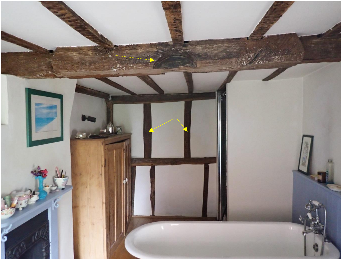
Figure 36: the new chamber in Bay 6. Note the arrowed timbers in the background, raising the eaves and the central floor beam with its redundant semi-circular housing.
