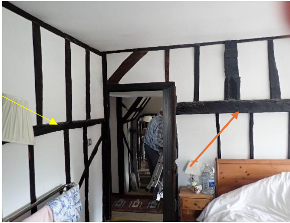
Figure 25: The Phase A wallplate and tie beam are arrowed, with Phase D1 timbers above.
