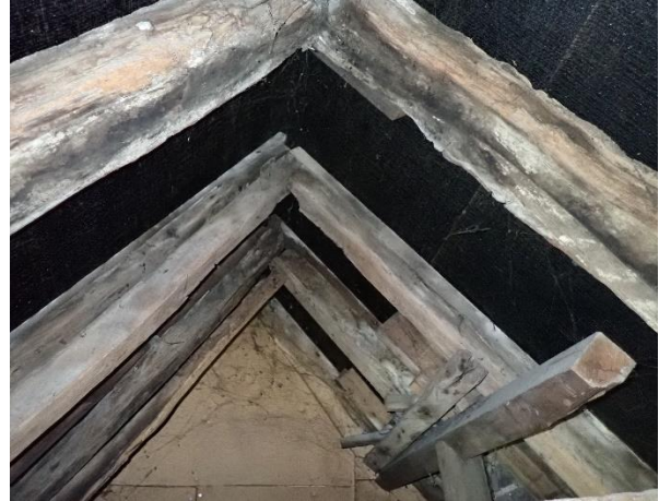
Figure 21: the oak common rafters over the Phase C2 extension.
