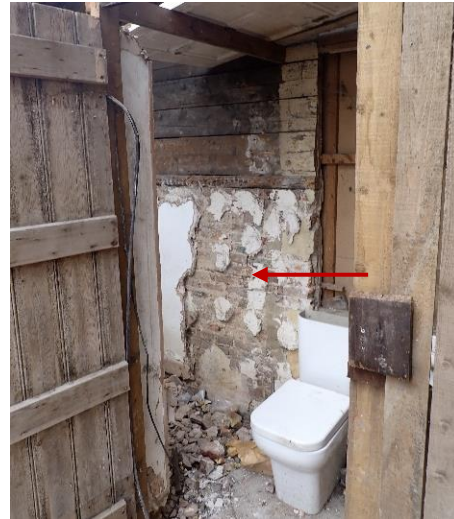
Figure 49: The end wall of the abutting Phase F.
