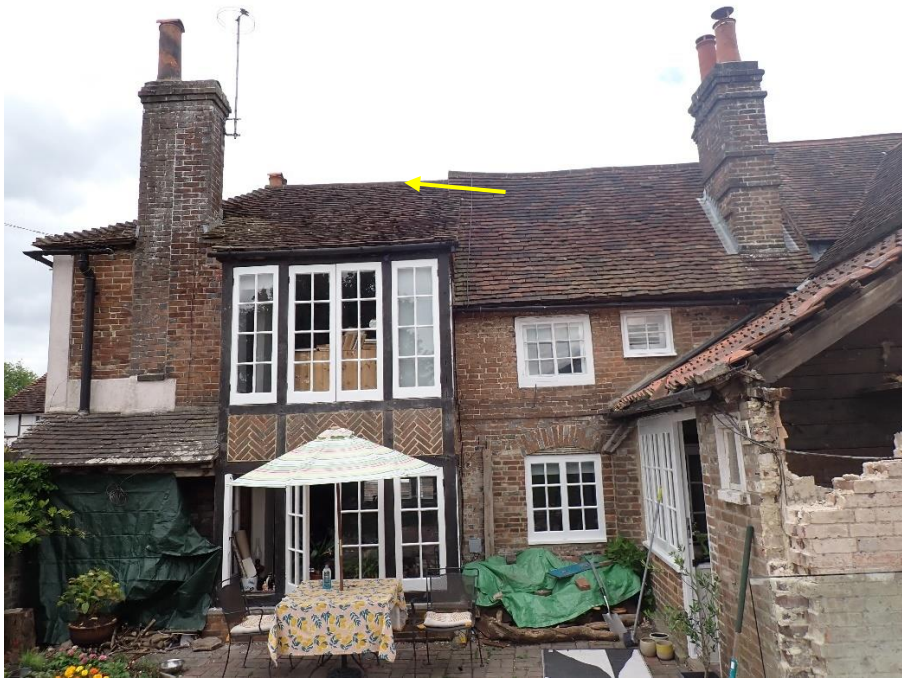
Figure 23: The raised eaves over Bay 2.
