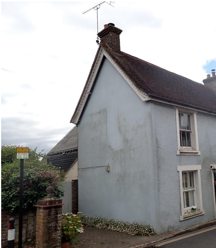
Figure 40: chimney at the north end of the main, front, range.
