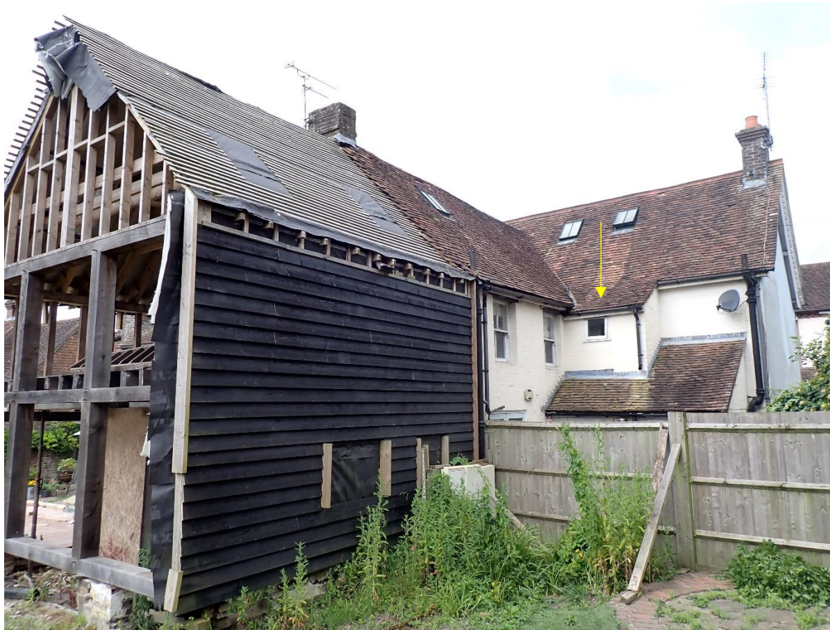
Figure 41: showing the raised eaves and roof of the rear range (left hand side) and the new outshot (arrowed yellow) to the main range.
