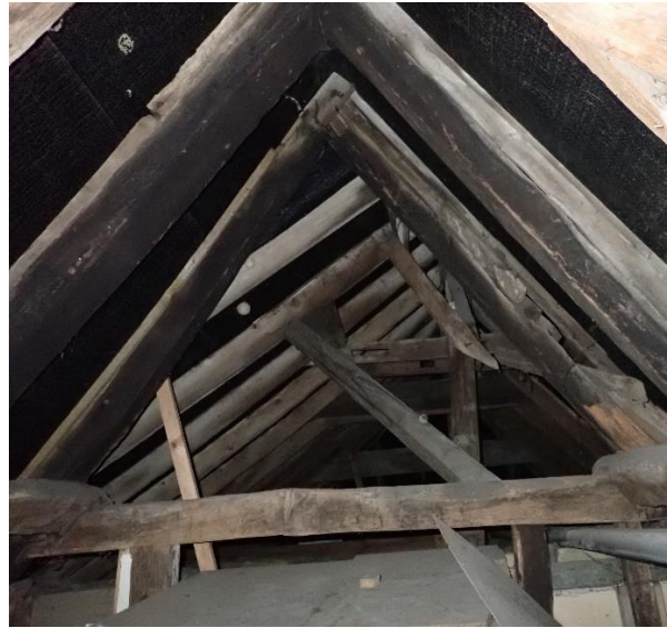
Figure 4: smoke-blackened common rafters in the foreground, over Bay 1.
