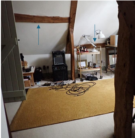
Figure 10: Staggered and tenoned side purlins.
