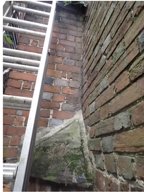
Figure 15: Brickwork of the chimney and flanking wall.
