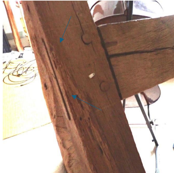
Figure 11: the principal rafter by the entry to the loft. The lack of framing pegholes indicate that there was no tenoned purlin in this bay, as it was intended to provide access.
