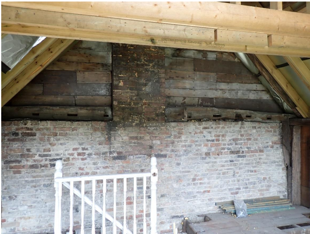
Figure 38: The new brickwork partition, chimney and re-used tie beam between Bays 6 and 7.
