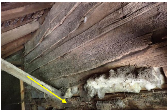
Figure 33: the Phase C1 wallplate (arrowed) with new timbers raising the eaves and weather-boarded, above.
