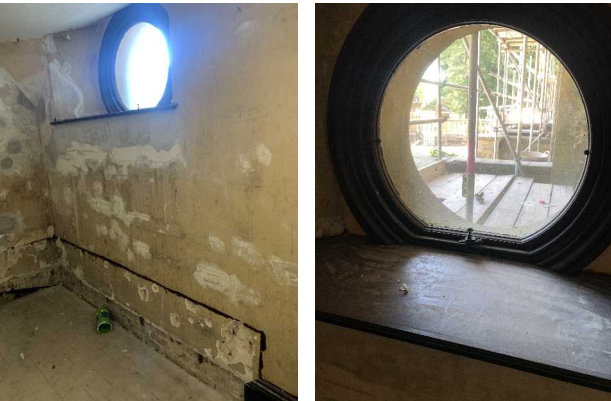
Circular windows seen in Ground Floor bathroom
