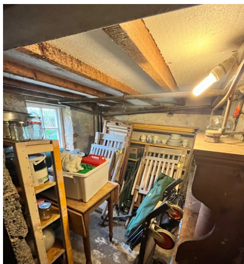
Modern floor joists and ceiling boards and blockwork partition wall in the rear range.
