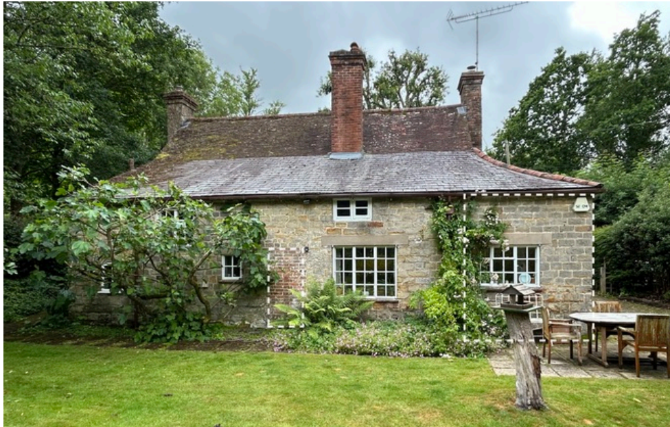
The rear elevation showing evidence of a former doorway and new stonework to the north.
