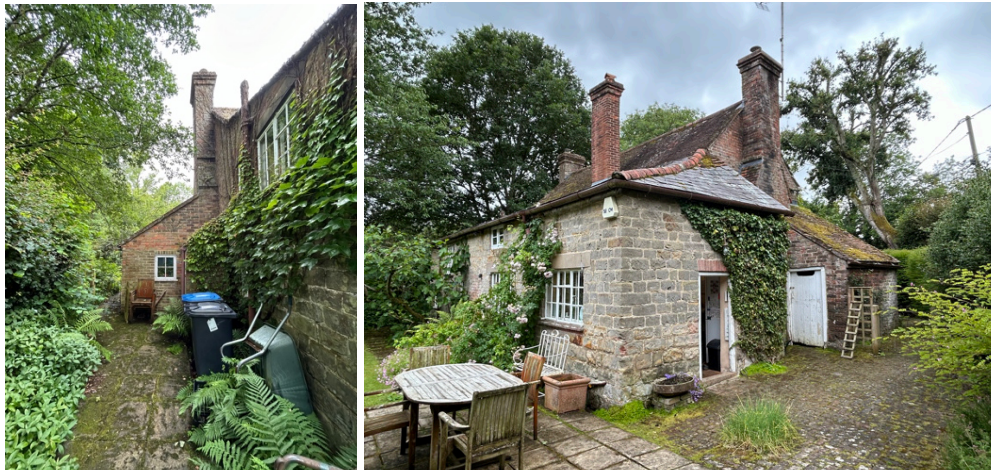
The north and south elevations which both have lean-to additions.
