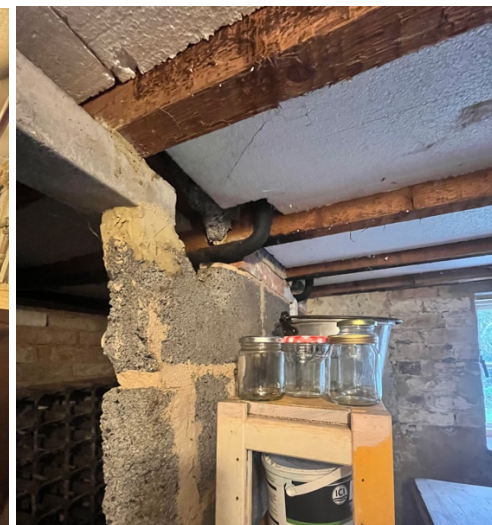
Modern floor joists and ceiling boards and blockwork partition wall in the rear range.
