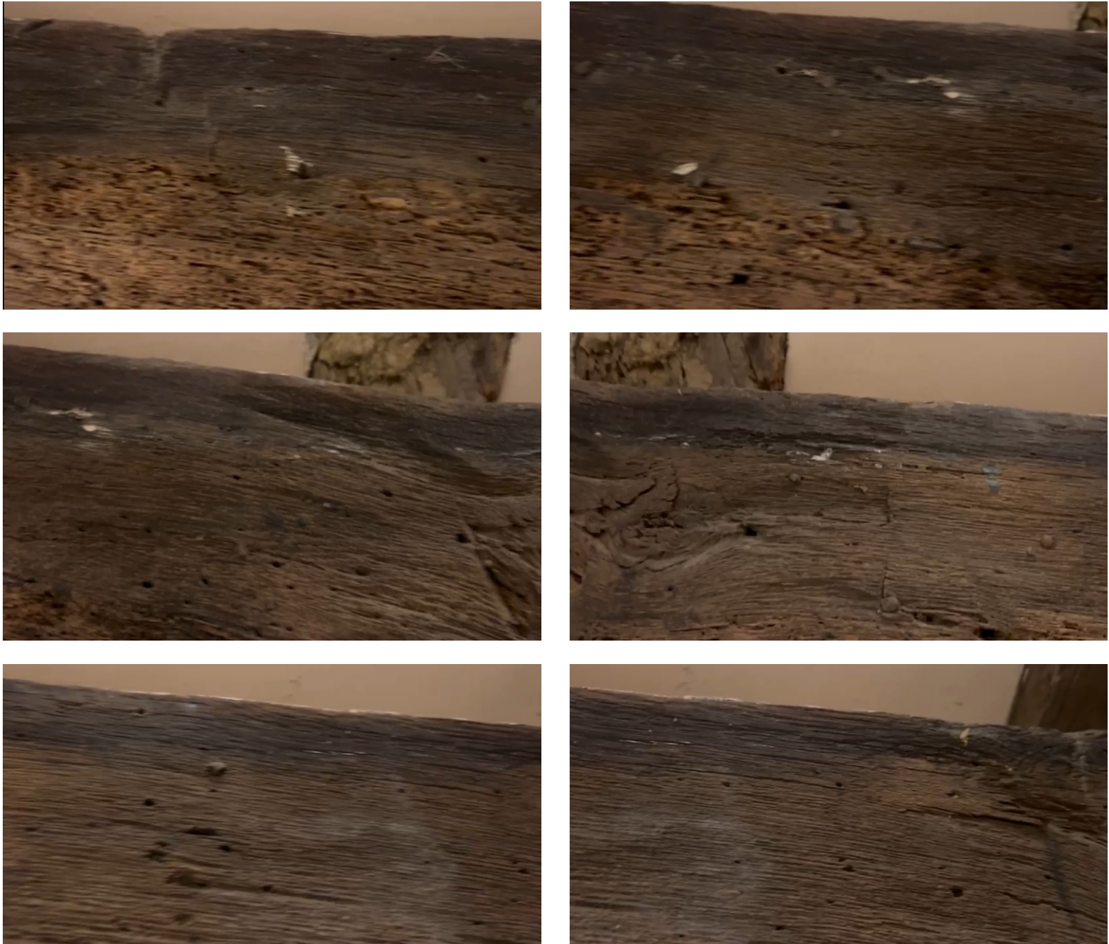
South bedroom timber frame photographs, November 2025
