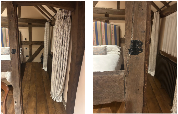
Photographs of the historic door frame hinge stain in the northern bedroom proving there was a door
