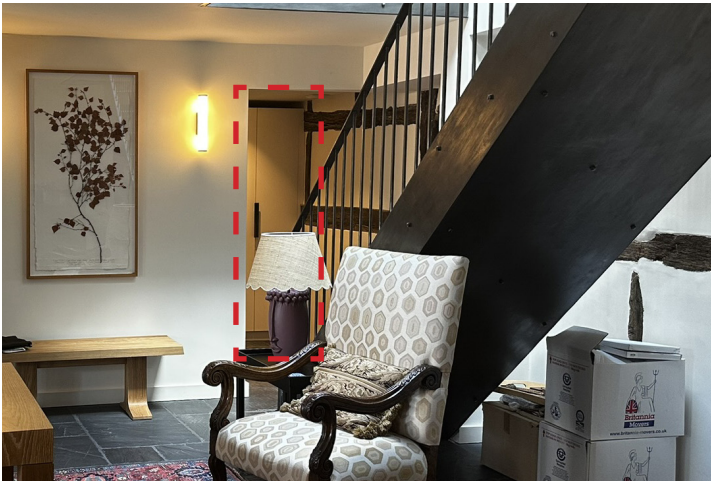
Photograph showing location of the door and exposed timber frame
