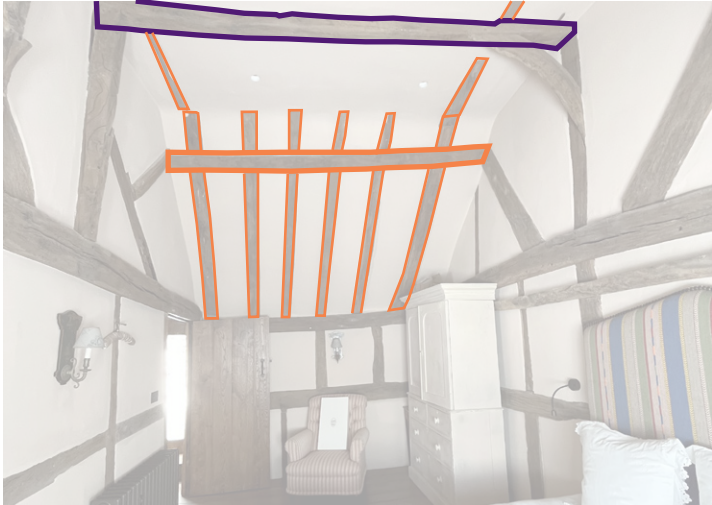
As Implemented - SE Bedroom
