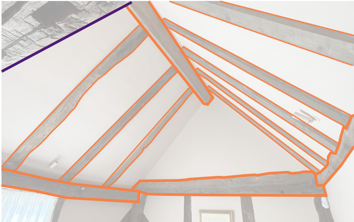
As Implemented - NE Bedroom
