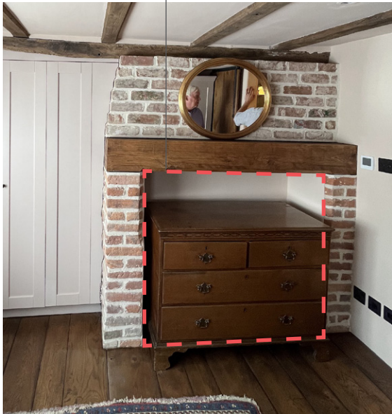
First floor bedroom re-faced chimney breast
