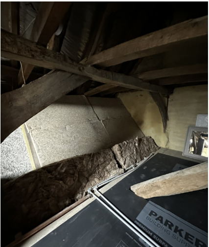
Attic, view of the vaulted ceiling
