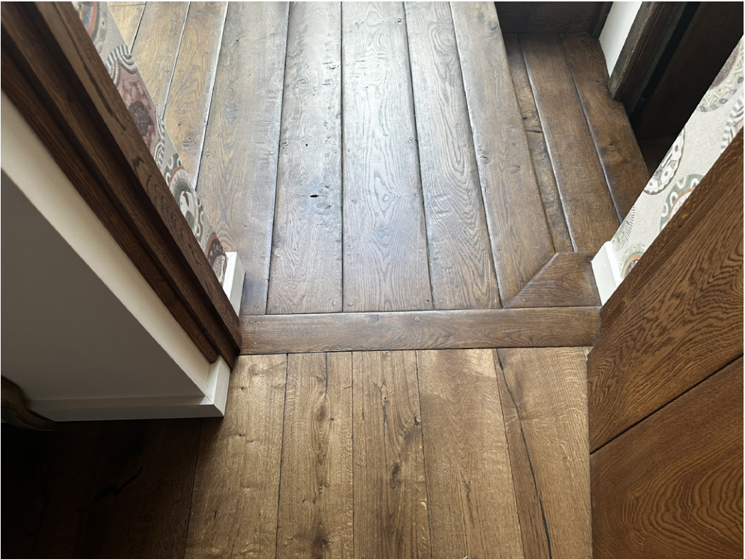
As-built oak flooring
