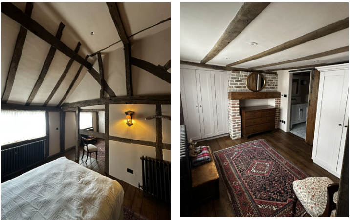
View from north bedroom towards altered wall (timber frame remaining) View towards new fitted wardrobe and en-suite wall and sliding door
