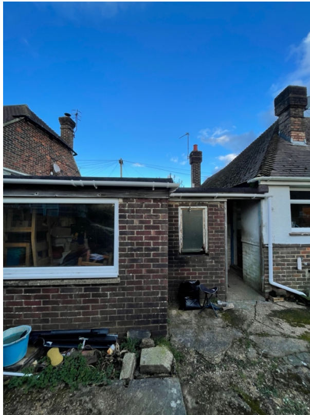
View looking north-east showing garage/store, rear & side elevation
