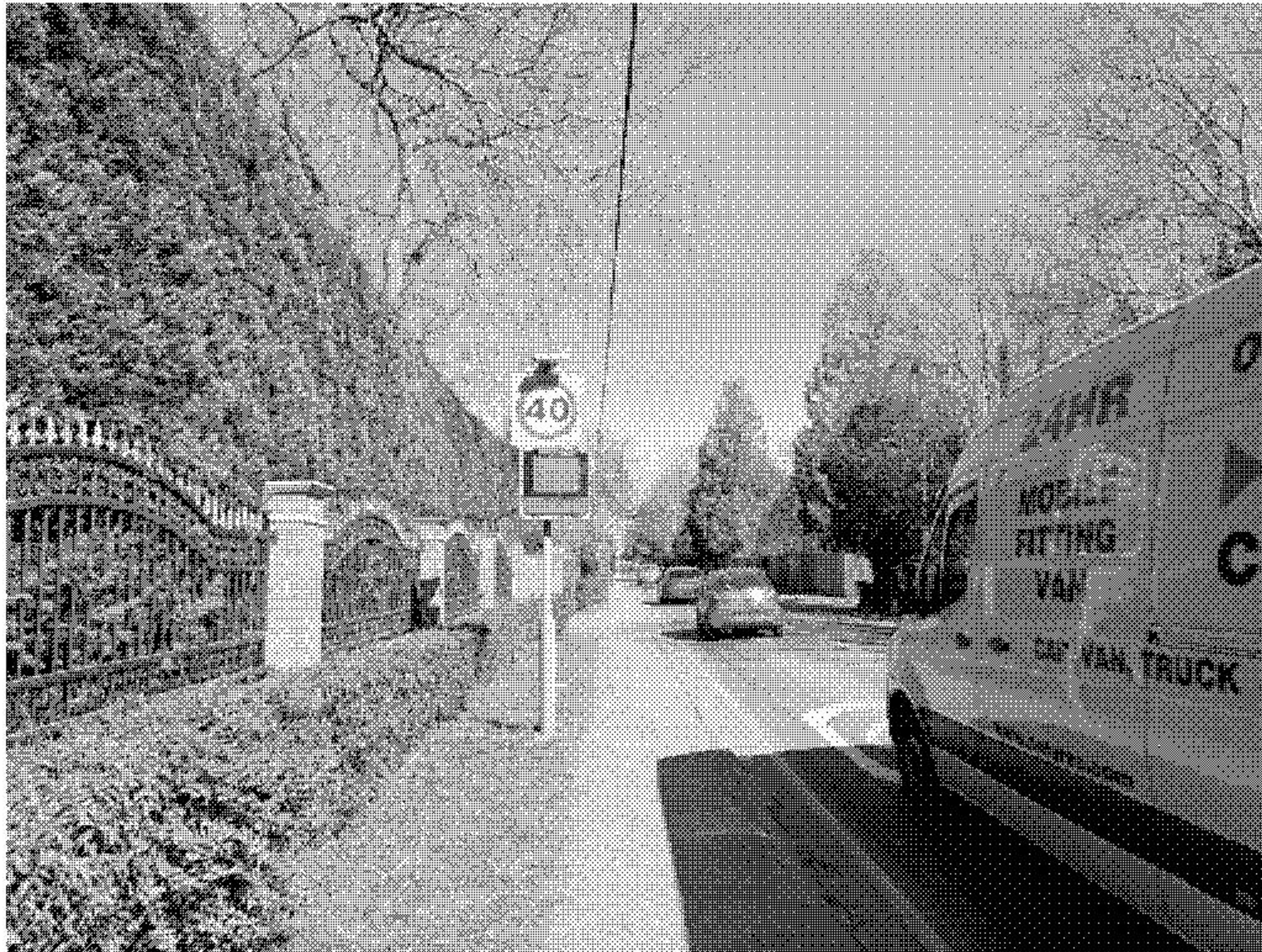
Figure 1: Vehicle-Activated Sign installed on A272
