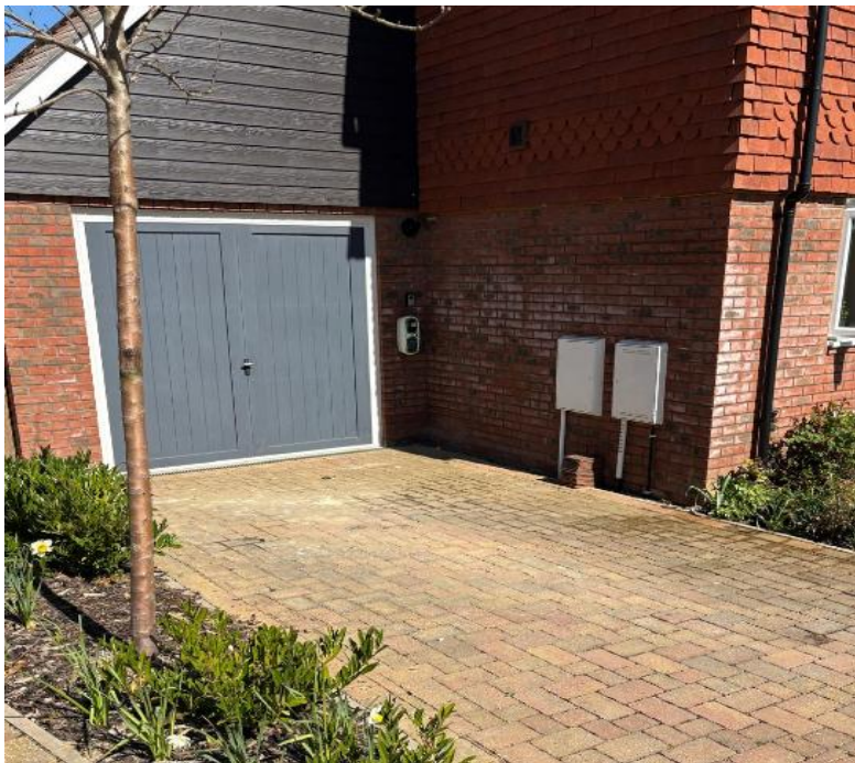
Appendix 6 – Development garage door remains in situ and street scene remains unchanged
