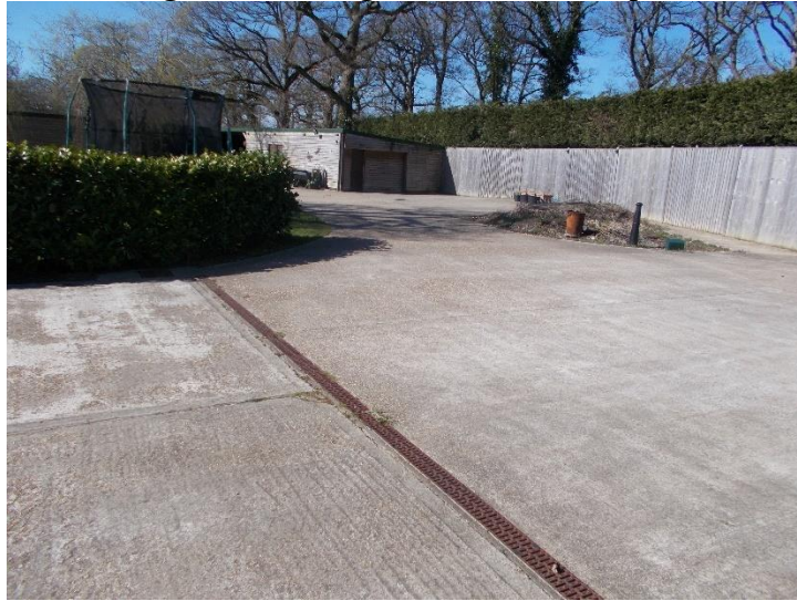
Parking area showing surface water strip drains
