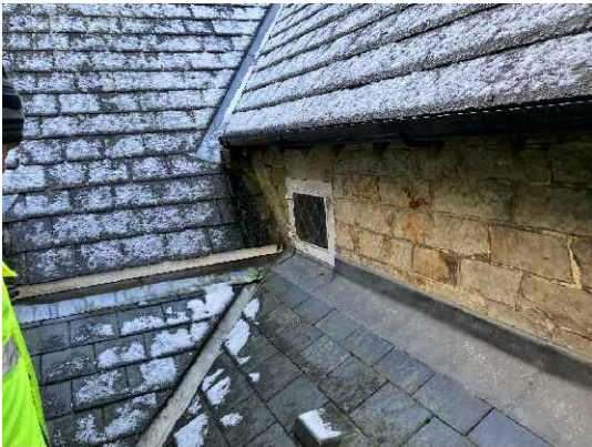
FIGURE 6: ORIGINAL SINGLE GLAZED TIMBER WINDOW TO BE RETAINED.
