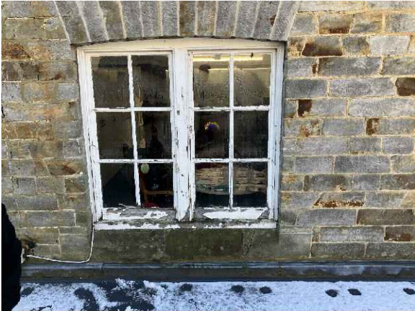
FIGURE 2: WINDOW TO BE REPLACED TO FACILITATE ACCESS. TO BE AGREED WITH CONSERVATION OFFICER
