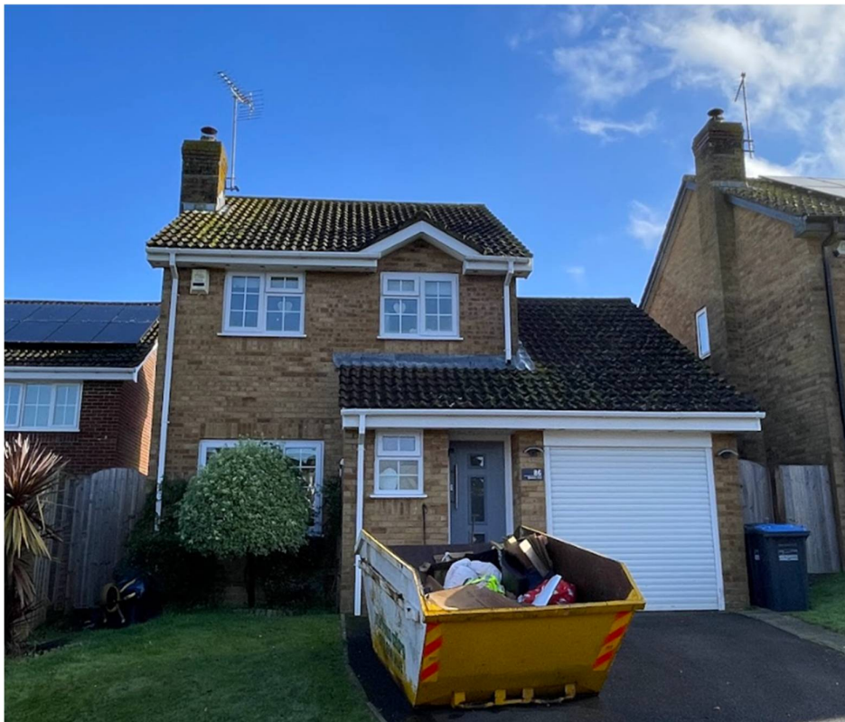
Photograph 1 – Existing front elevation
