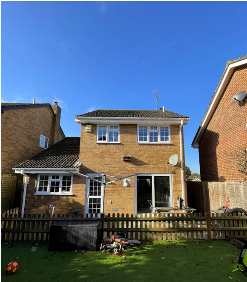
Photograph 2 – Existing rear elevation of the property
