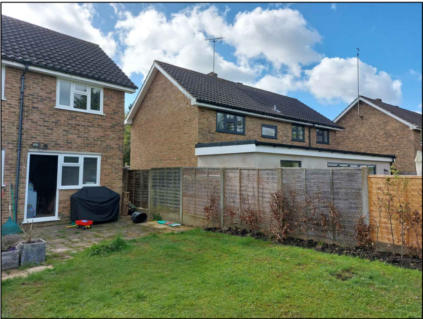
2 - Rear elevation looking to 15 Blackthorns
