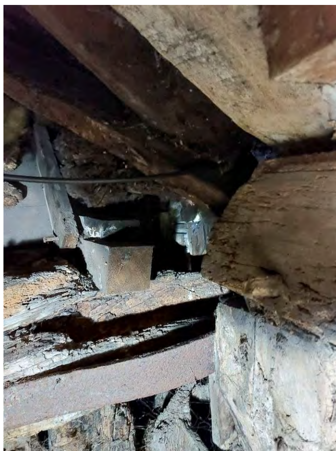
Photograph 2: NE corner of Bay 5
