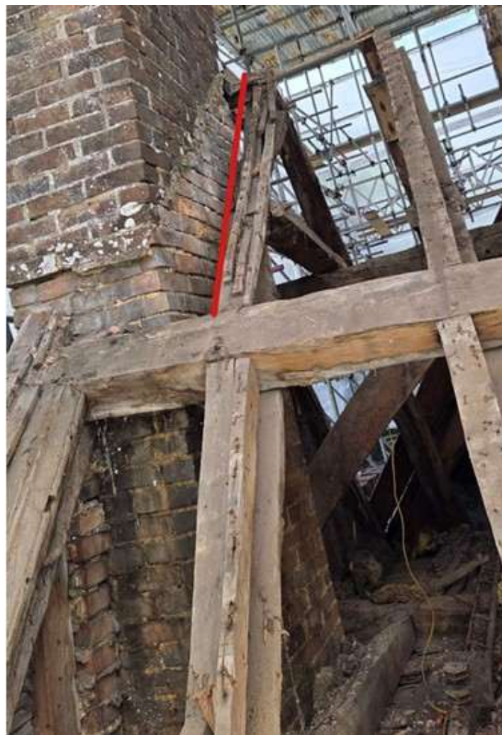
Photograph 18: Rafter formed from multiple firring pieces
