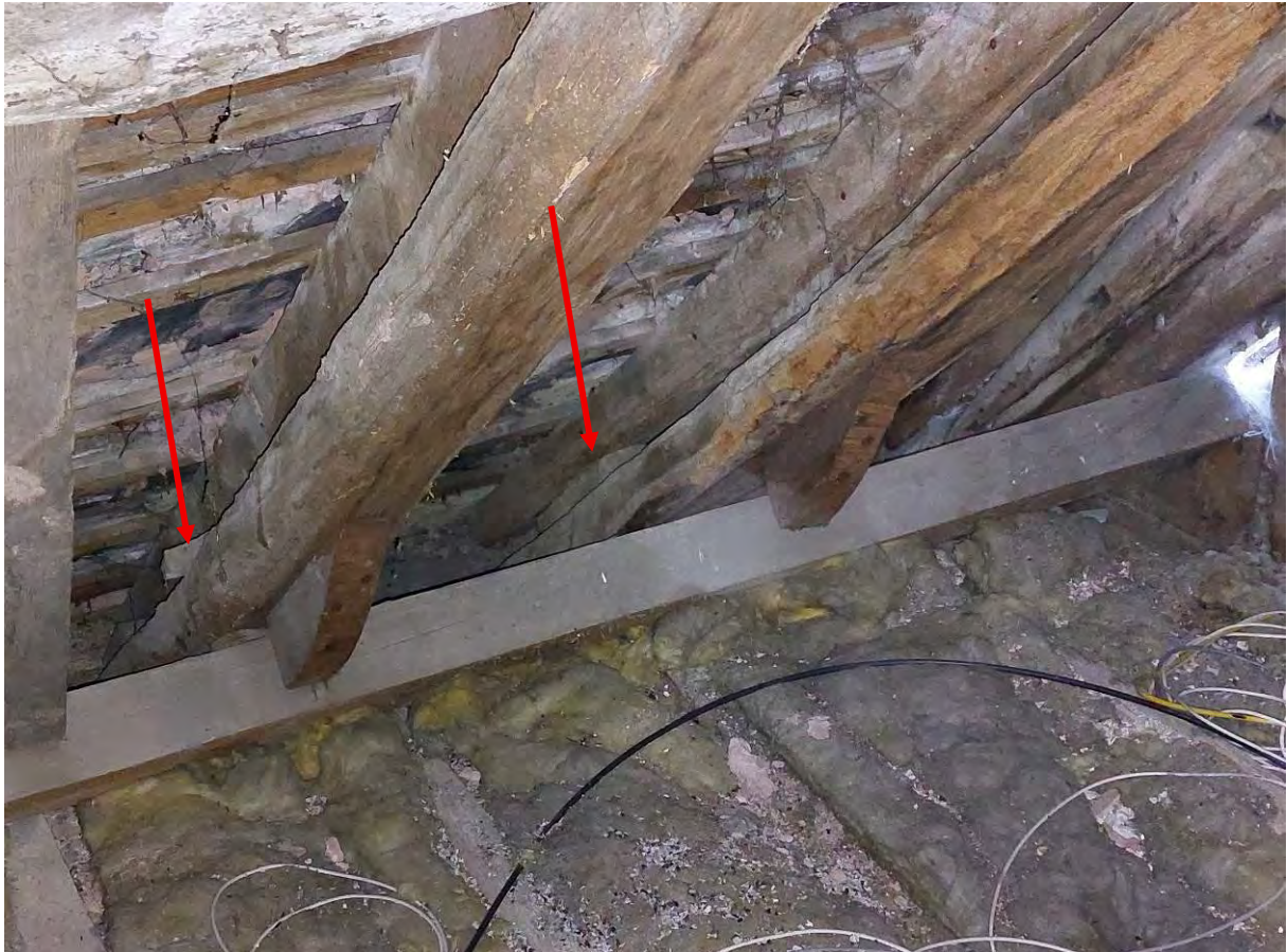
Photograph 6: Wedges between earlier rafters and added rafters
