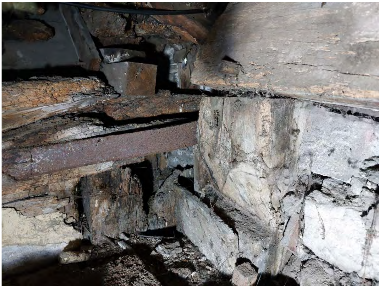
Photograph 1: NE corner of Bay 5
