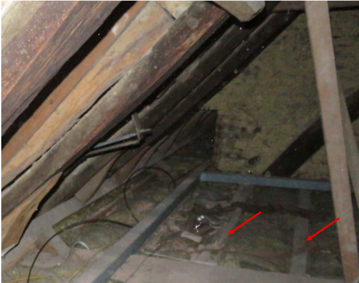
Photograph 14: Ceiling joists in Bay 4
