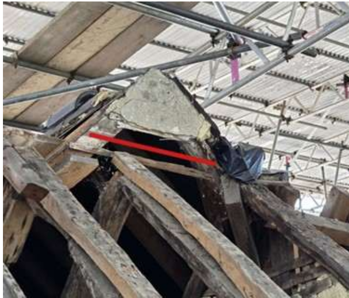
Photograph 19: Interface between Main Range roof and East Range roof
