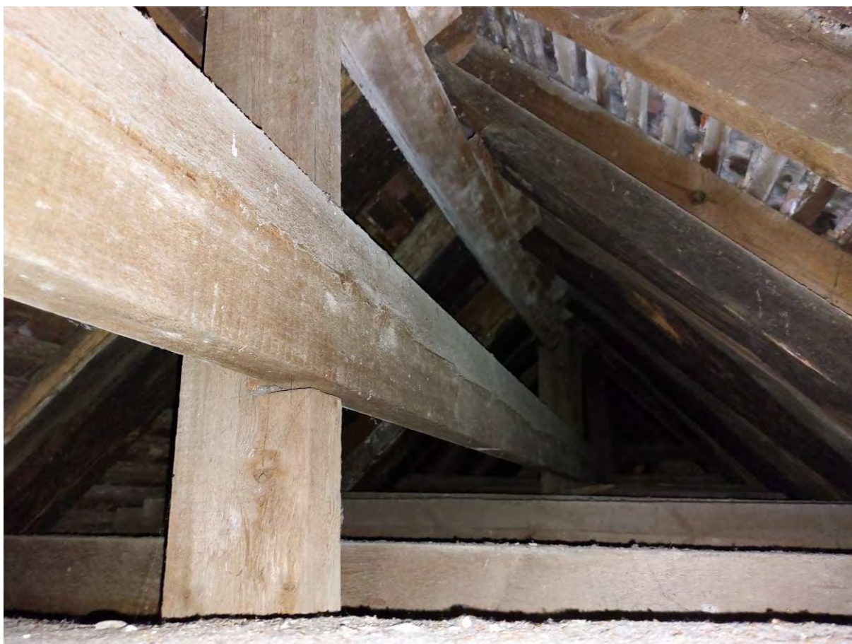
Photograph 10: Added frame above collars purlins to Bay 3 and 4
