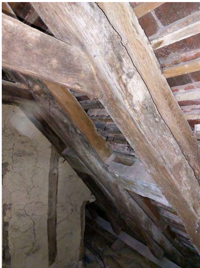
Photograph 3: Purlin to west elevation of Bay 5
