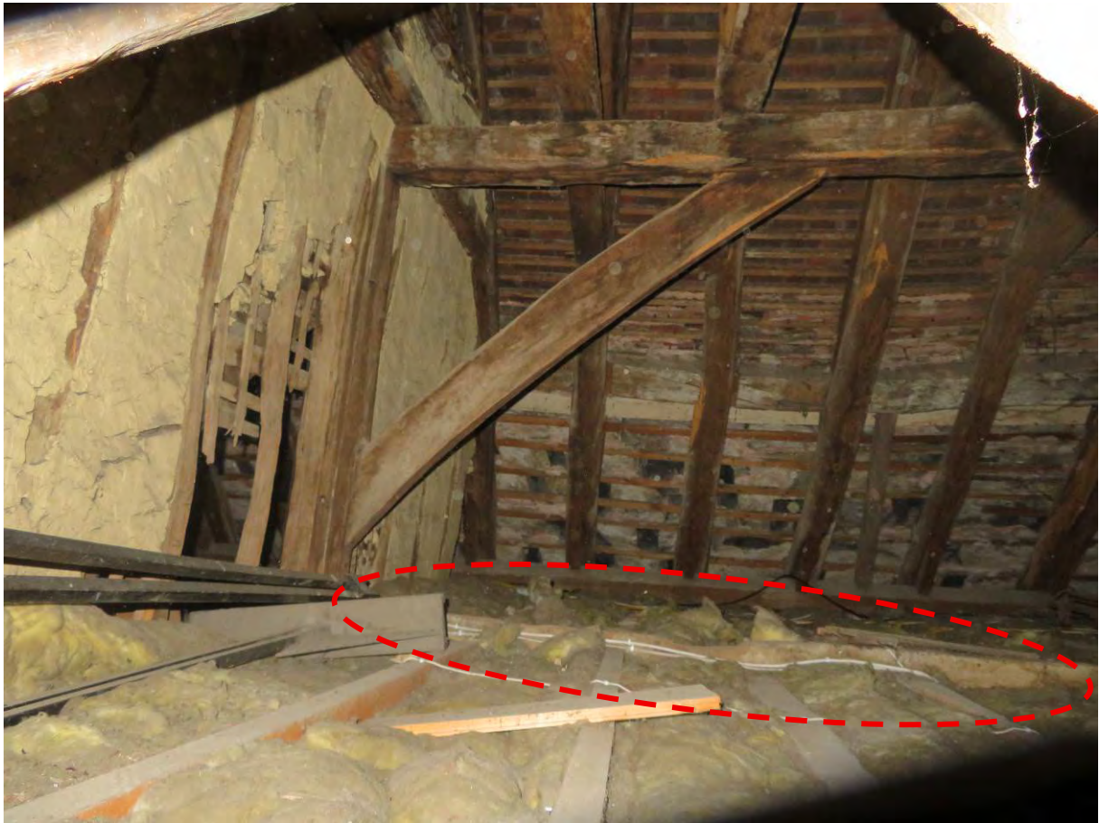
Photograph 13: Ceiling joist and spine beam jointing to Bay 5
